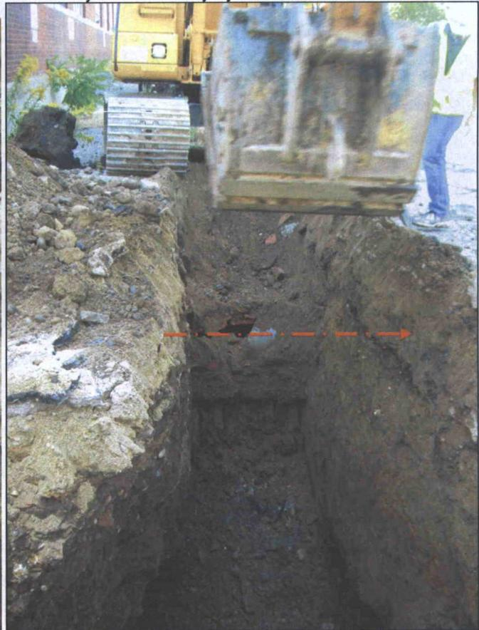
17. Mon. 8/1/11 Left Photo: Looking east down TP-2 toward the outer wall the concrete tank. Soil here was compacted and competent (the location of an old Libbey Mill building?). A branch of TP-2 also extends south (right) toward the building. The arrow near the bottom marks a 20" diameter old water pipe into the substation building basement.
