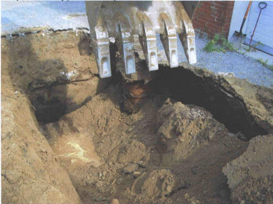
20. Mon. 8/1/11: Excavation of **Test Pit TP-4** within the smaller, south concrete tank compartment. Water was found within the compartment with no evidence of oil saturated soil of free product. In the center is what appears to be a buried 55-gallon drum that may have been a manway.
