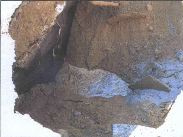
13. Mon. 8/1/11: In TP-1, water in the tank with a discontinuous layer of black oil. The concrete tank's walls appeared reasonable well cleaned. Gray oil-contaminated soil but not oil-saturated soil was found within the bottom several feet depth of the concrete tank (Soil sample SS-1).
