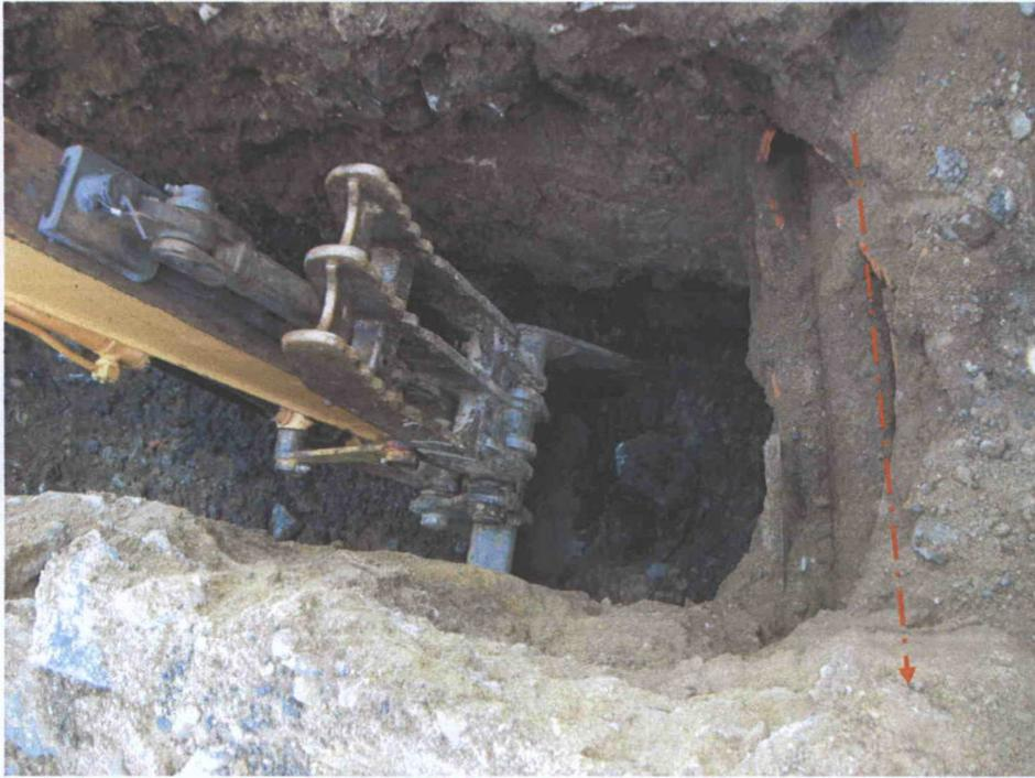
19. Mon. 8/1/11: Looking down into south end of TP-2 over the 15" clay pipe with the 8" iron (offset fill) pipe exposed. That goes west under Mill Street to the location of the Libbey Mill UST facility (see P-561-2011).
