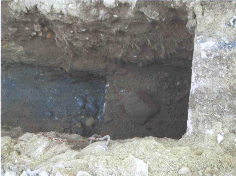
14. Mon. 8/1/11: **Test Pit TP-2** located just outside the west tank wall with black-oil saturated soil below the footer for the concrete UST (circled) on the silt/clay soil layer.
