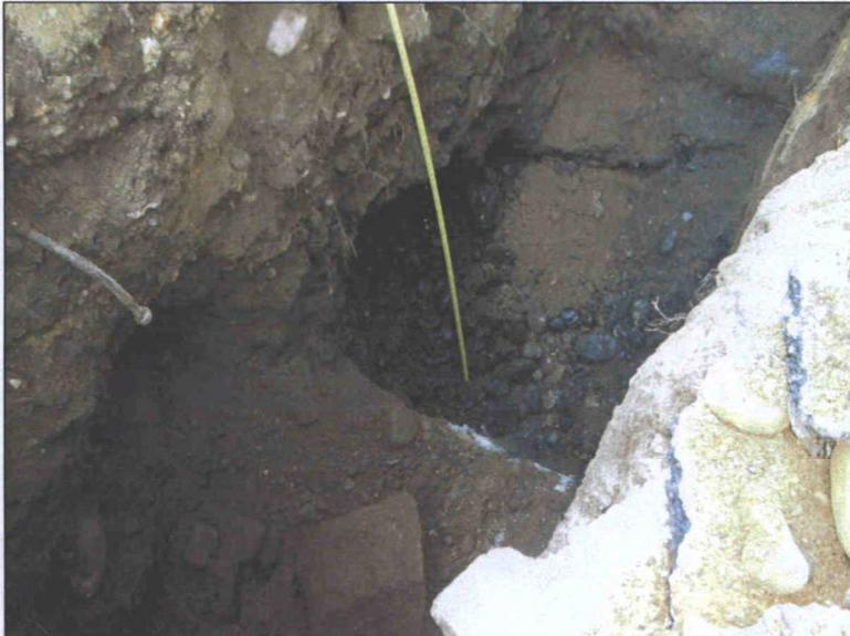
15. Mon. 8/1/11: Another view into oil-saturated soil at the north end of TP-2 @ about 7.5' below grade. At lower left is the concrete footer for the UST.
