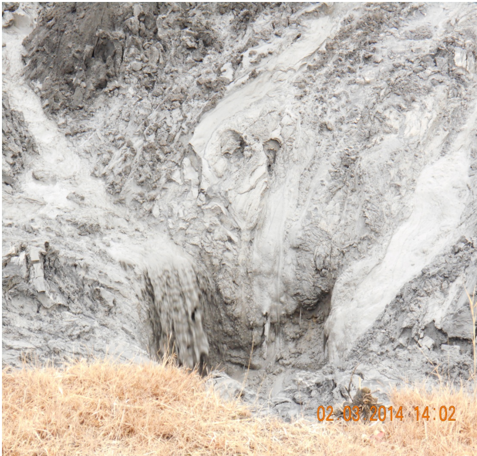
Close-up of 48" RCP failure area.
