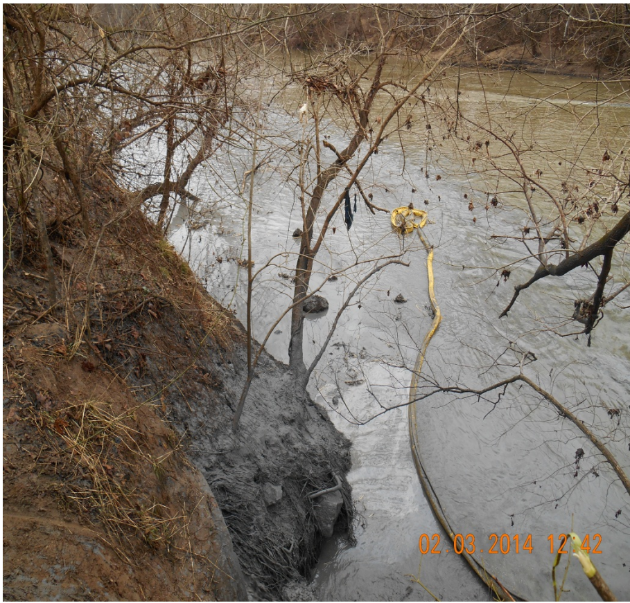
Looking at outlet of 48" RCP where it empties into the Dan River. You can visibly see the ash plume in the river.
