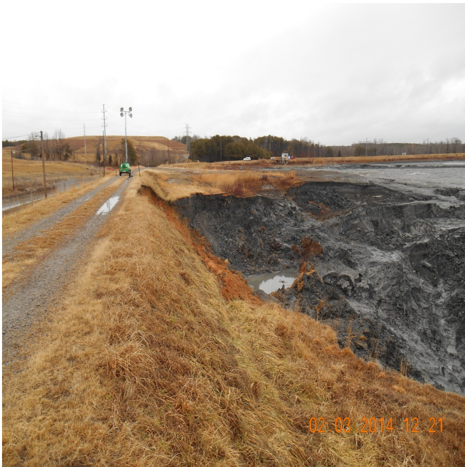
Looking at upstream slope failure on west side of dam. Slope is vertical back to crest of dam. Picture taken on west side of dam looking toward northeast direction.
