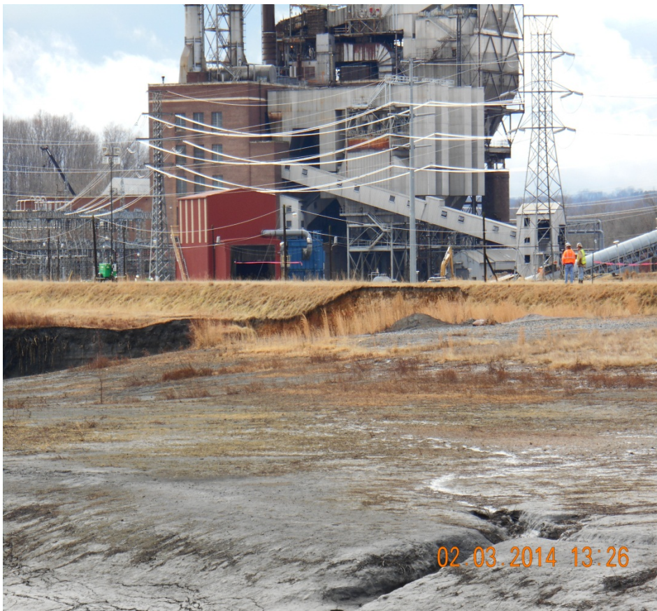
Standing on riser intake structure looking across impoundment area. Close-up of upstream slope failure.
