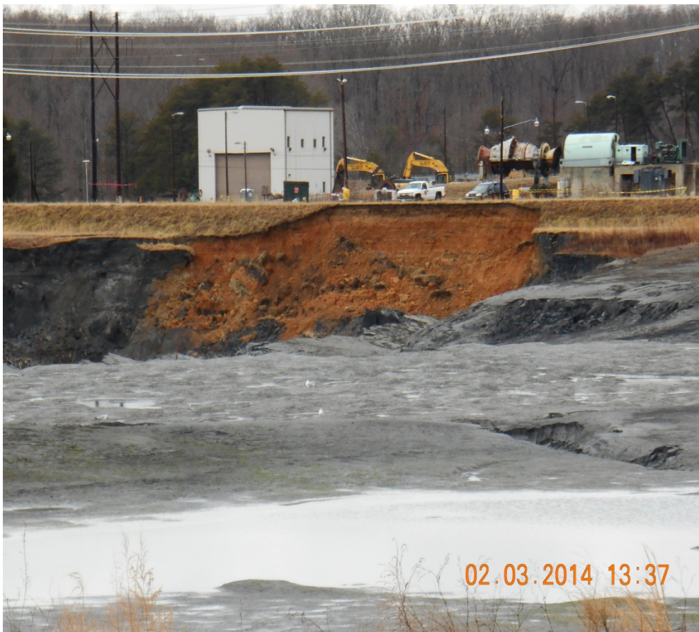
Standing on northeastern embankment looking across impoundment area to west embankment. Close-up of upstream slope failure.
