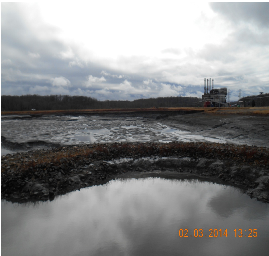
Standing on riser intake structure looking toward pipe failure area and upstream slope of the west side of dam.
