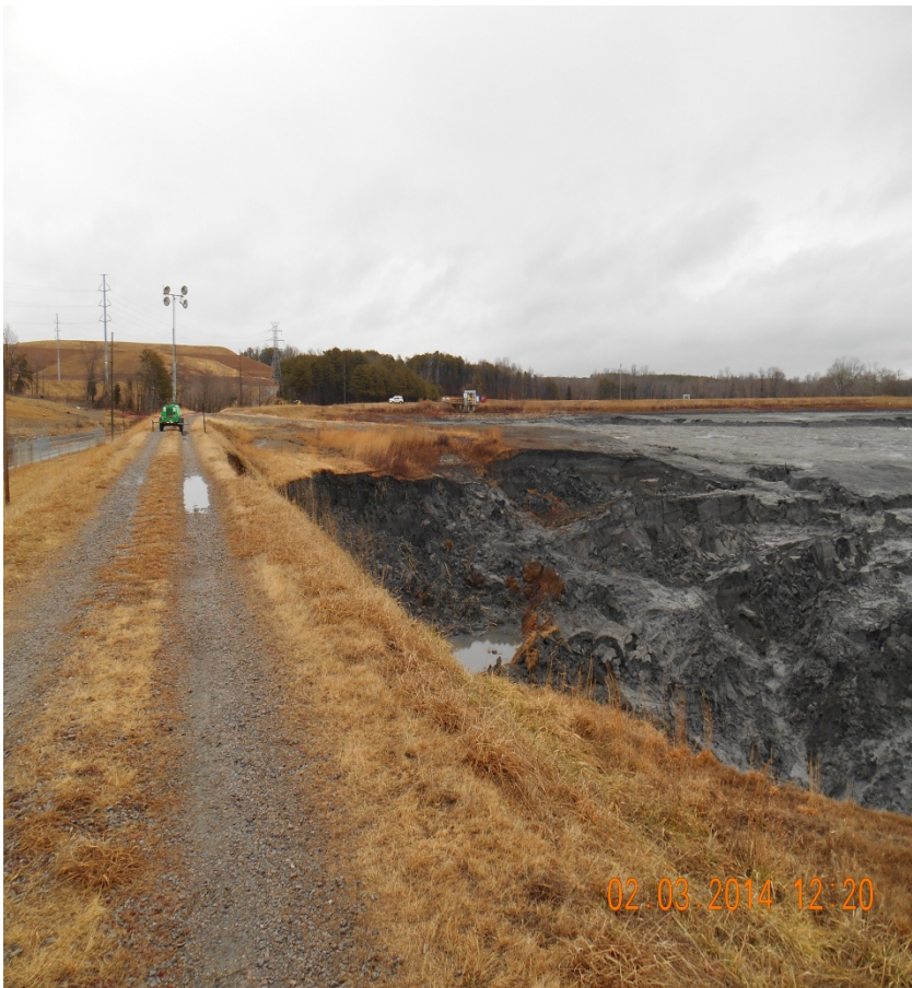
Looking at upstream slope failure on west side of dam. Slope is vertical back to crest of dam. Picture taken on west side of dam looking toward northeast direction.
