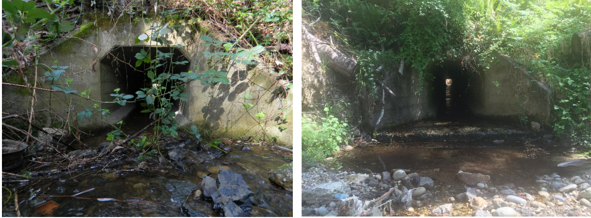
Figure 3. Existing Box Culvert Inlet (Left) and Outlet (Right)
