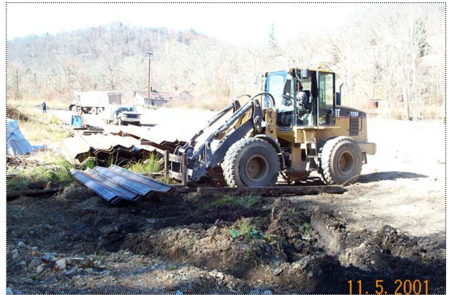
DCP01099 - Ahern personnel and fork lift moving and stacking sheet prepared for driving
