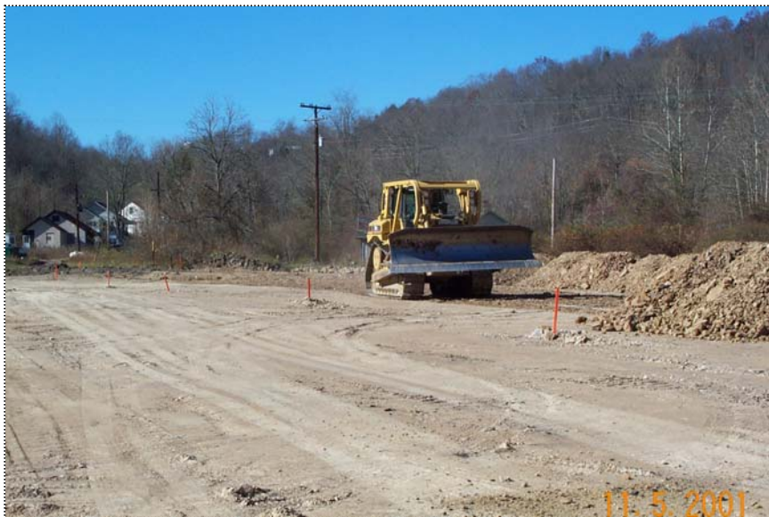
DCP01094 - Dozer scarifying the fill, before placing the next lift
