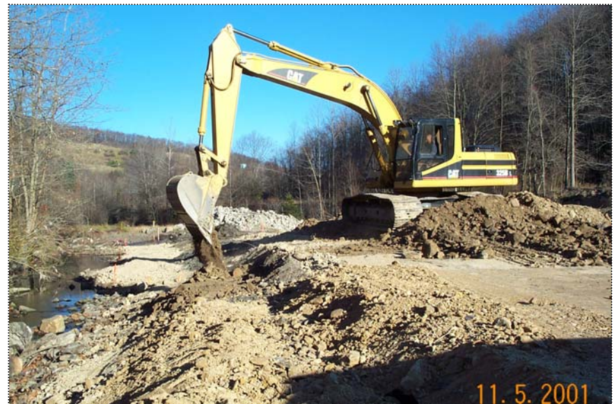
DCP01103 - Track hoe placing sub grade material on the sheet pile alignment
