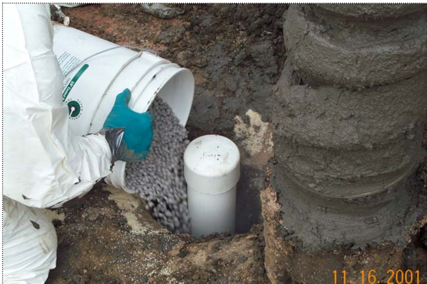
DCP1287 - Triad personnel placing bentonite tablets in the bore hole around the stand pipe
