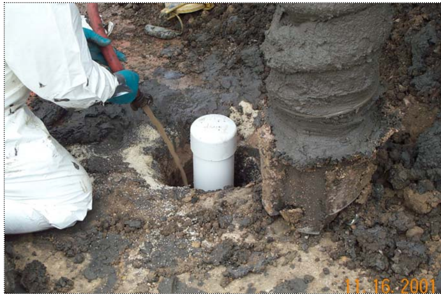
DCP1288 - Triad personnel adding water to hydrate the bentonite
