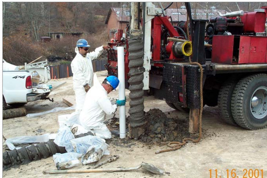
DCP1289 - Triad personnel installing additional stand pipe on SS-12
