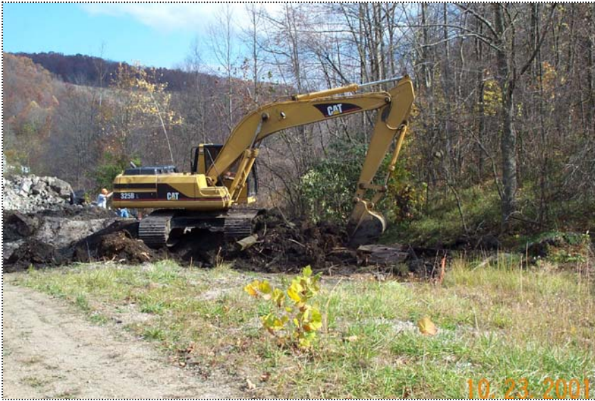
DCP0989 - Track Hoe excavating new drainage feature per drawings. (Found ditch intercepted a gas main, relocated entrance to Arbuckle creek)
