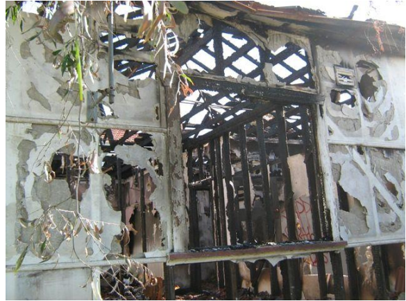
Asbestos in fire-damaged building
