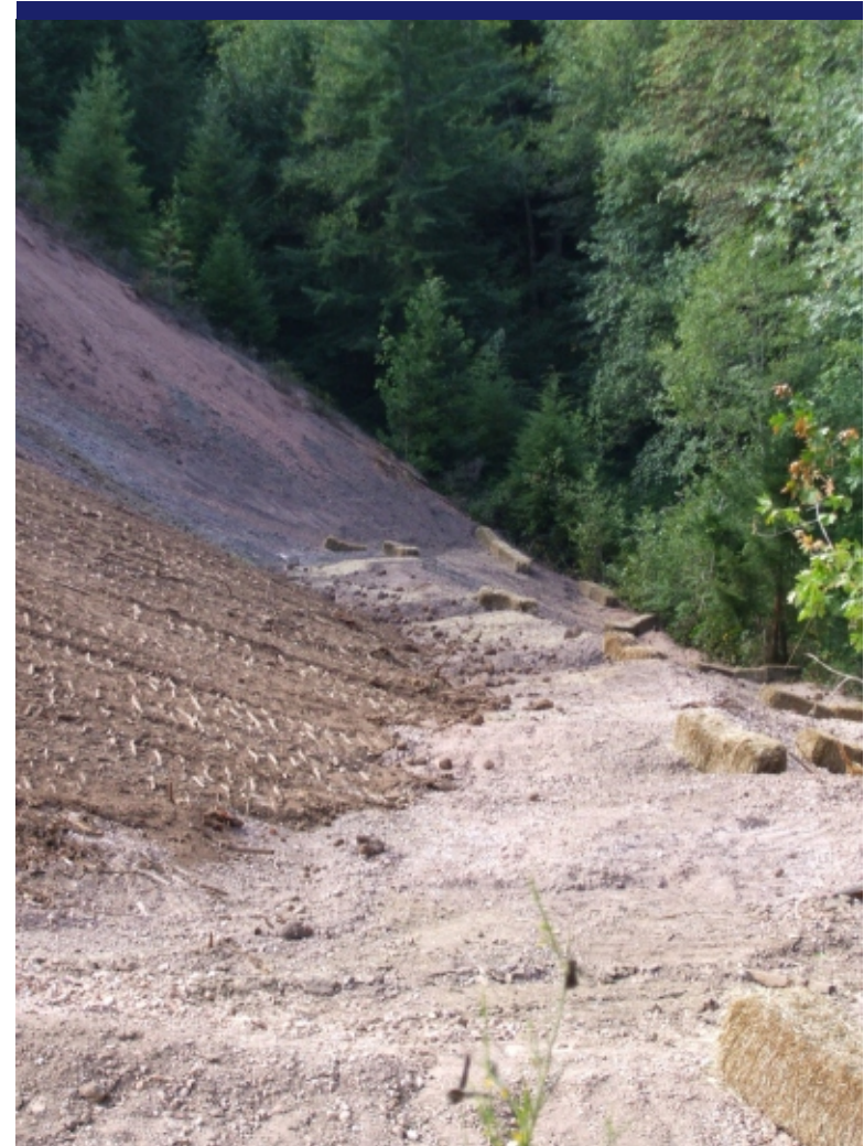
Photo 6 Main Tailings Pile - West slope showing soil cap and water bar.
