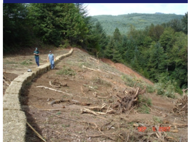
Photo 13 Main Tailings Pile - West slope showing woody debris placed on surface. Direction: West Date: 9/4/2007 Time: By: KP
