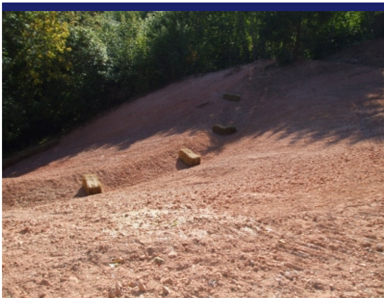
Photo 20 Main Tailings Pile - East slope prior to topsoil and hydroseed.
