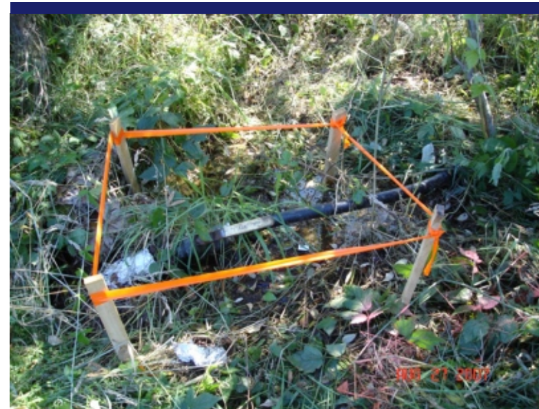
Photo 31 High visibility flagging around residential water line.
