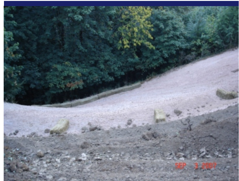
Photo 25 Straw bales at base of Main Tailings Pile - East slope.
