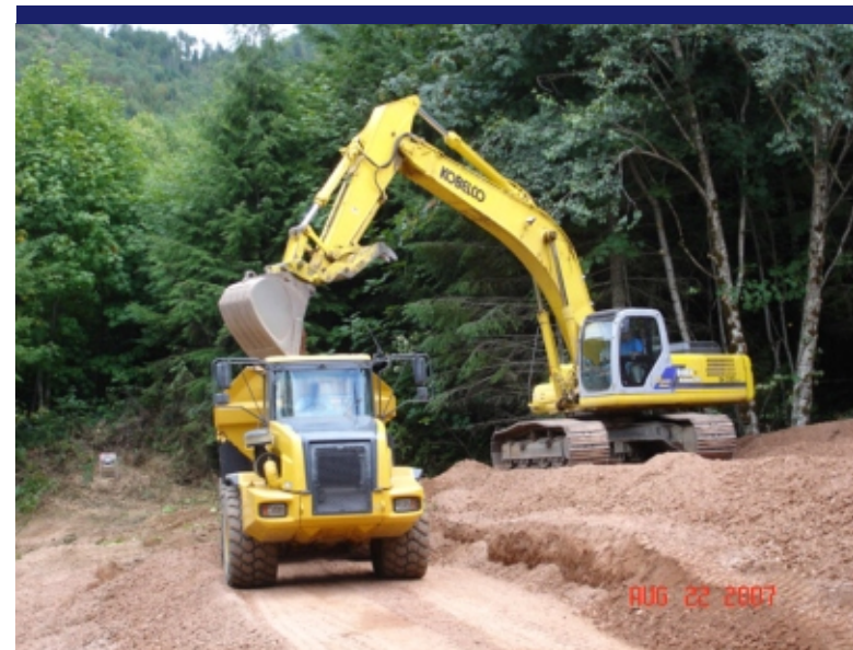
Photo 17 Main Tailing Pile - East slope tailings removal.
