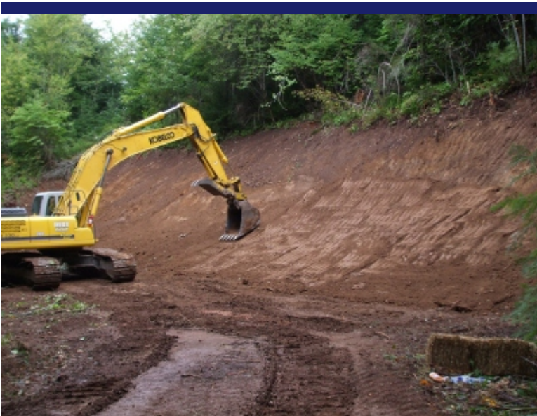
Photo 52 South of New Furnace - Slope reconstruction after fill material removal.
