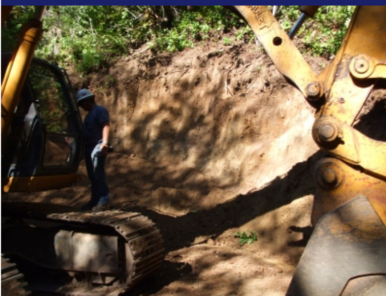
Photo 50 Soil removal area near New Furnace for final Main Tailings Pile slope cover.
