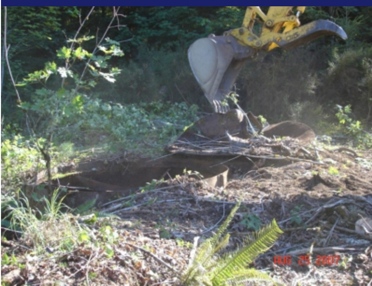
Photo 28 Opening buried tank in Old Ore Furnace Area.
