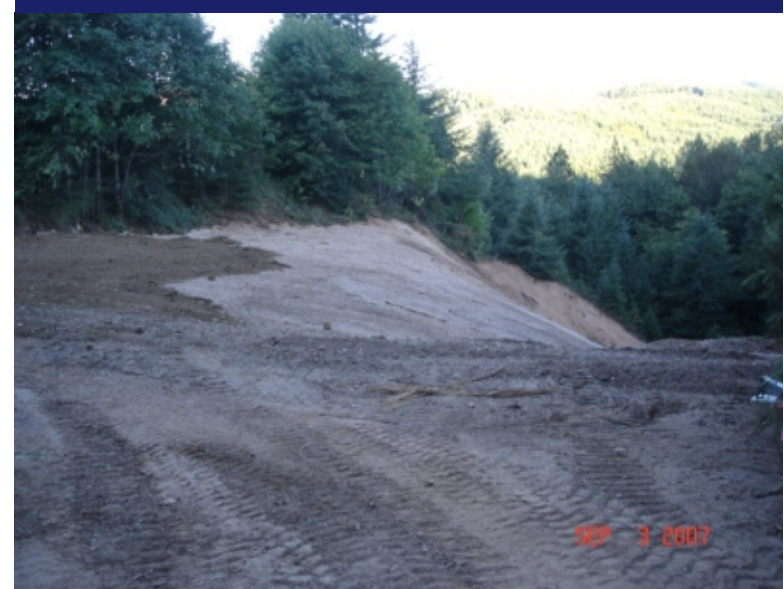
Photo 9 Clean soil placed on top of Main Tailings Pile - West slope.
