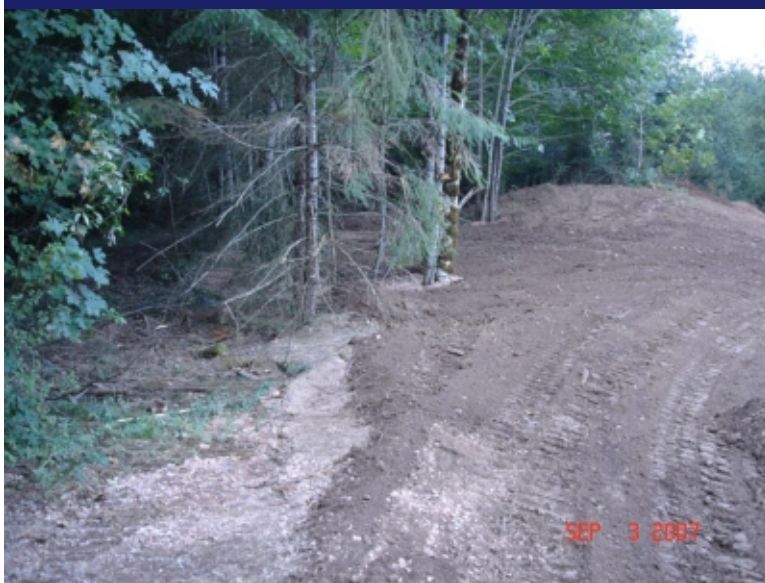
Photo 26 Clean soil placed on top of Main Tailings Pile - East slope.
