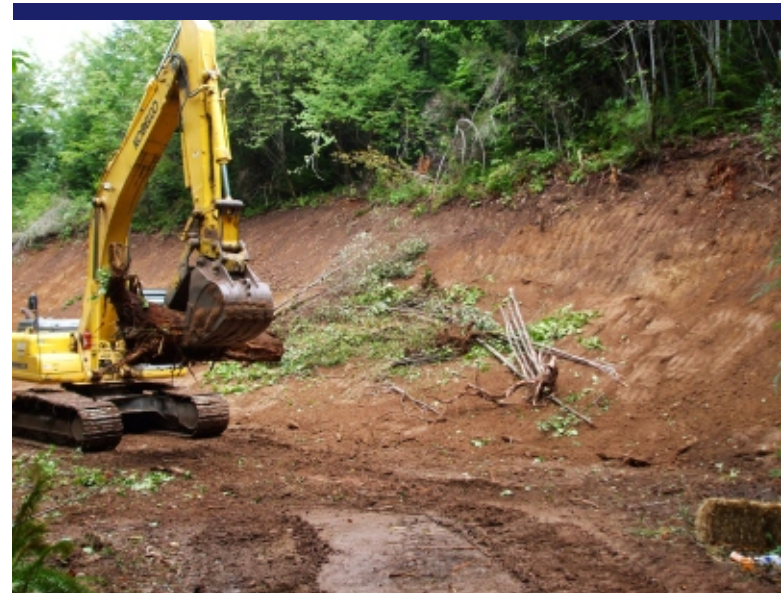
Photo 53 South of New Furnace - Slope reconstruction after fill material removal.
