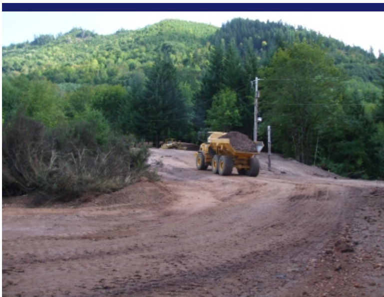
Photo 34 Hauler taking capping materials to Old Ore Furnace for capping.
