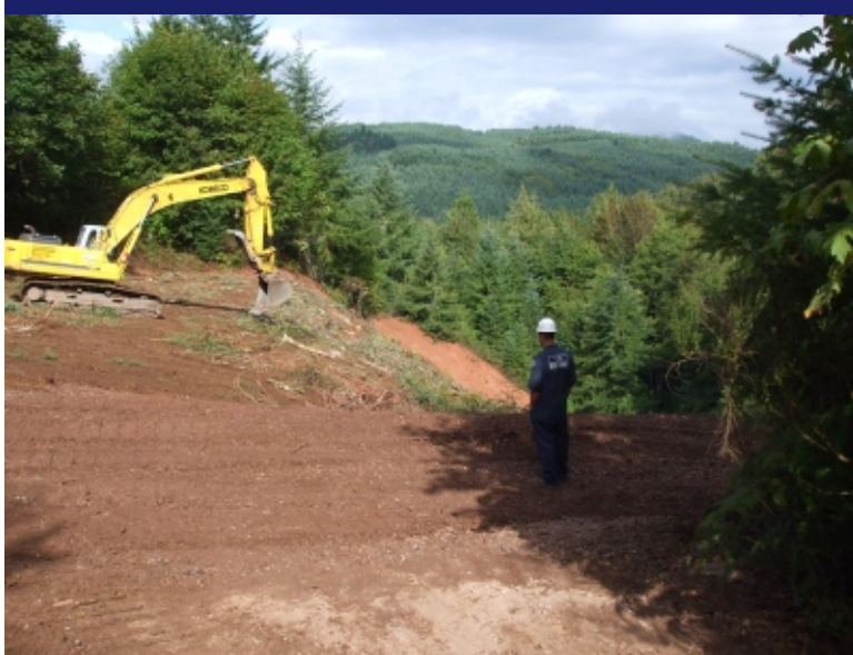
Photo 12 Main Tailing Pile - West slope showing soil cap with woody debris on surface . Direction: North Date: 9/4/2007 Time: 10:01 By: BC
