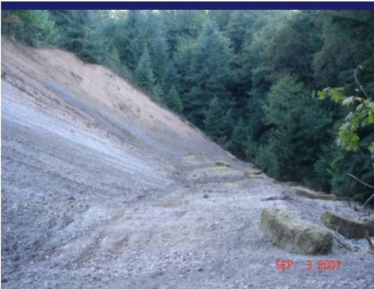
Photo 7 Straw bales placed on Main Tailings Pile - West slope.
