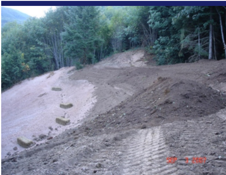
Photo 24 Clean cover soil placed on Main Tailings Pile - East slope.
