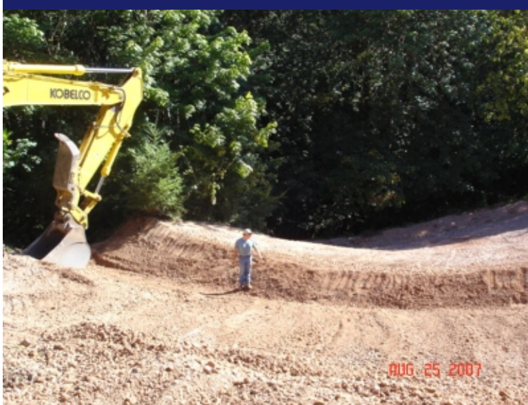
Photo 18 Cutting water bars on Main Tailings Pile - East Slope.
