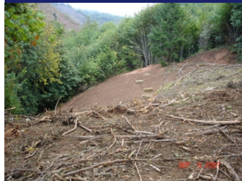
Photo 27 Woody debris placed on final slope of Main Tailings Pile - East slope.
