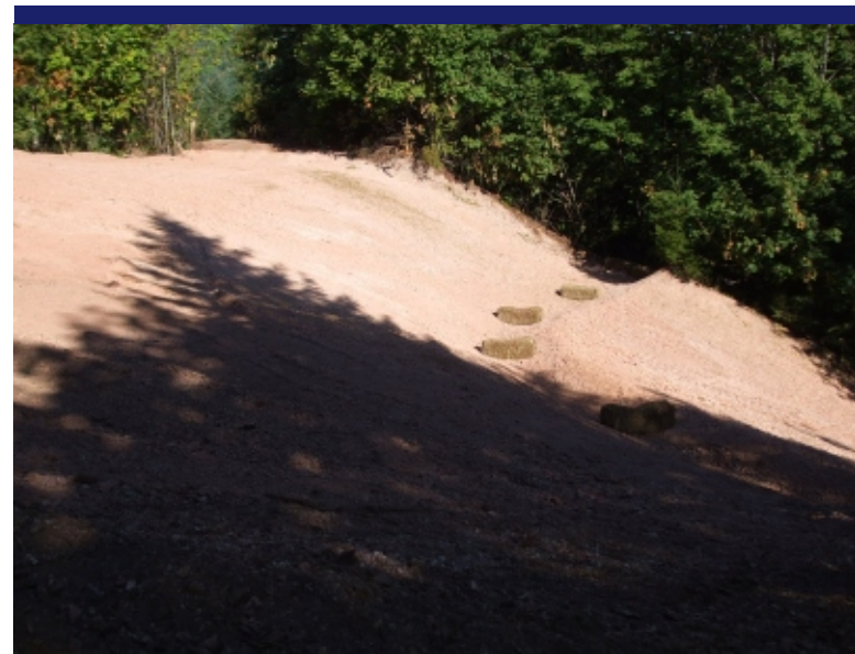
Photo 21 Main Tailings Pile - East slope prior to topsoil and hydroseed.
