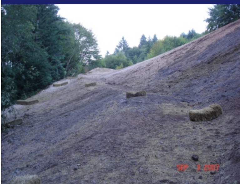
Photo 8 Straw bales placed on Main Tailings Pile - West slope.
