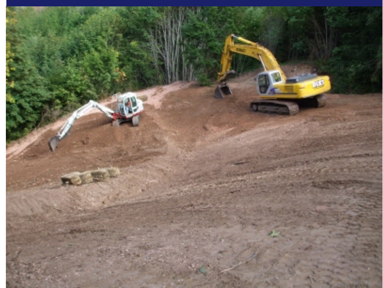
Photo 23 Main Tailings Pile - East slope adding soil cap.
