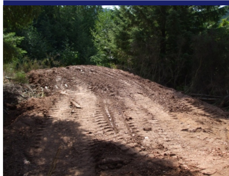
Photo 33 Capped tailings at area down slope of Old Ore Furnace.
