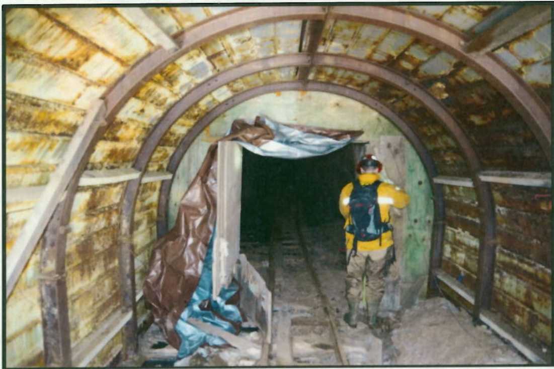
Photo 6: First Air Door to be replaced
