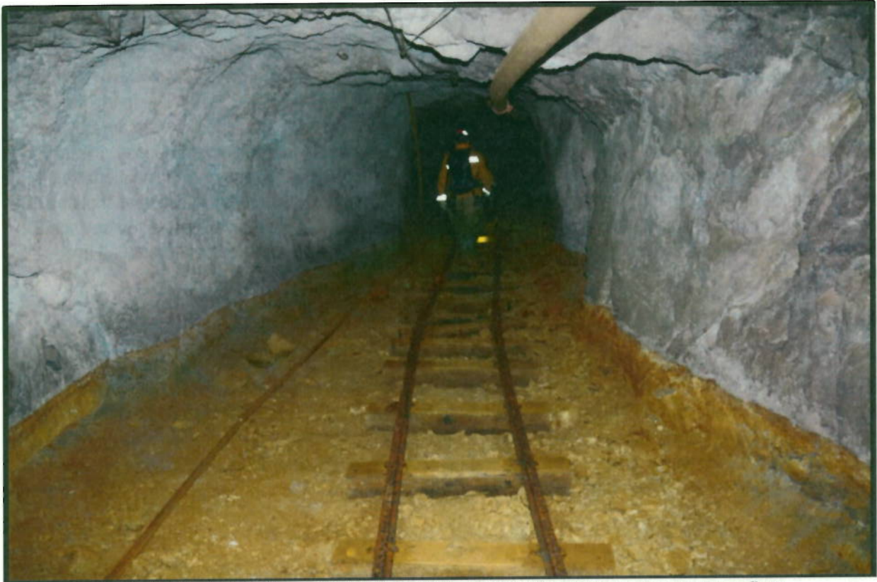
Photo 59: Typical draft near 50+00; Note high water line from upper mine pool overflow
