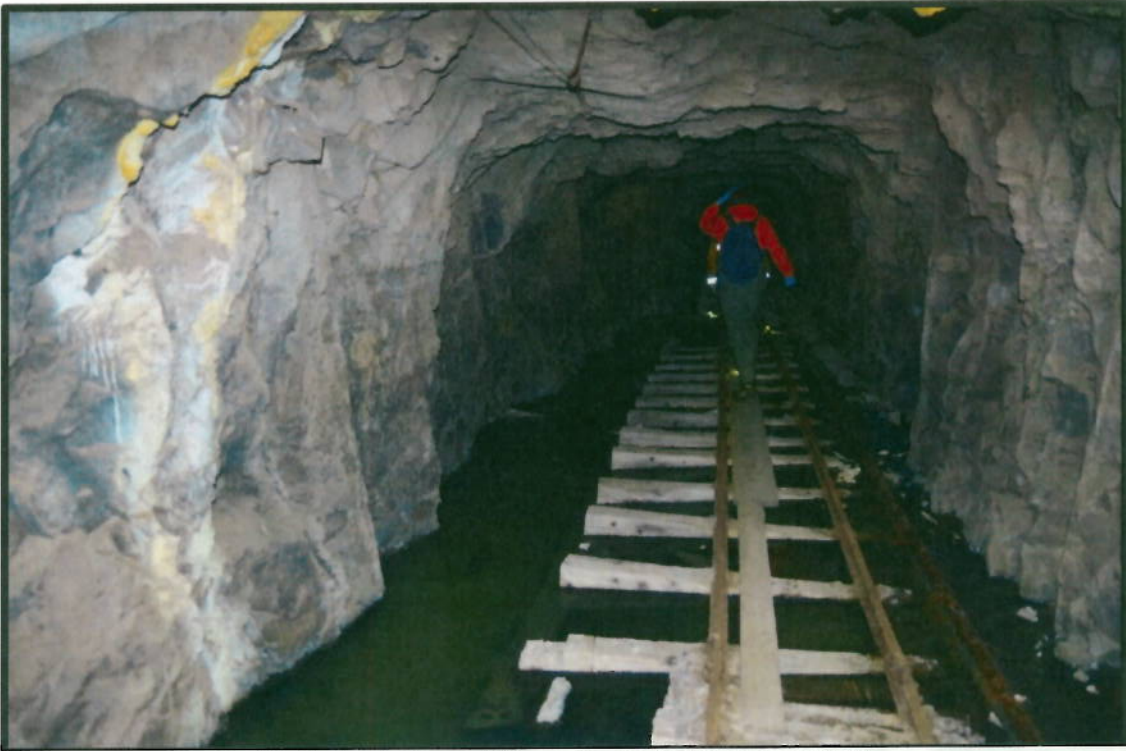
Photo 7: Floating rail ties and poor drainage near 1+00
