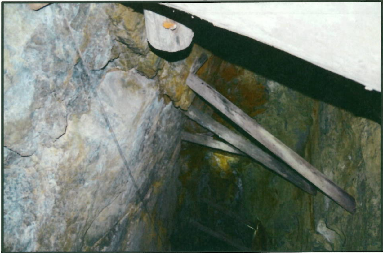
Photo 35: Typical timber stulls; Note hanging wall, Amethyst vein, and foot wall
