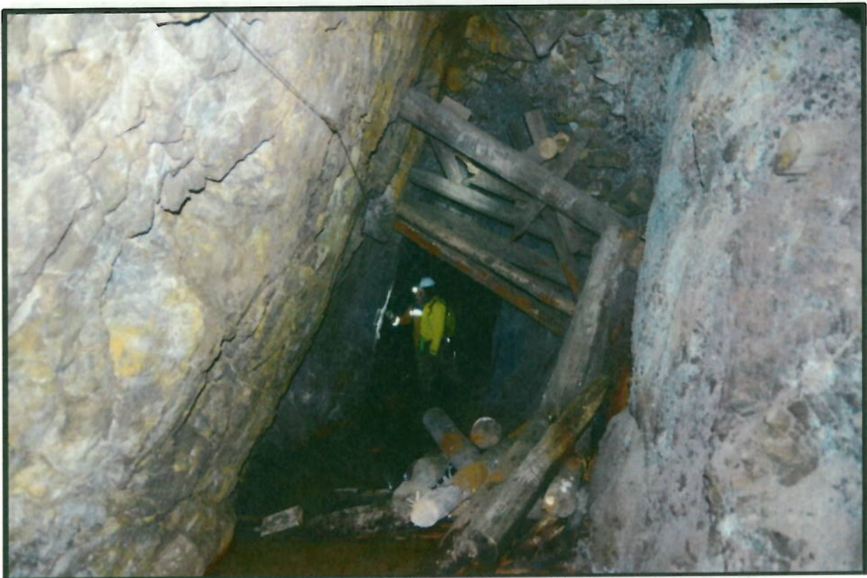
Photo 40: Failed timber stulls near 32+80
