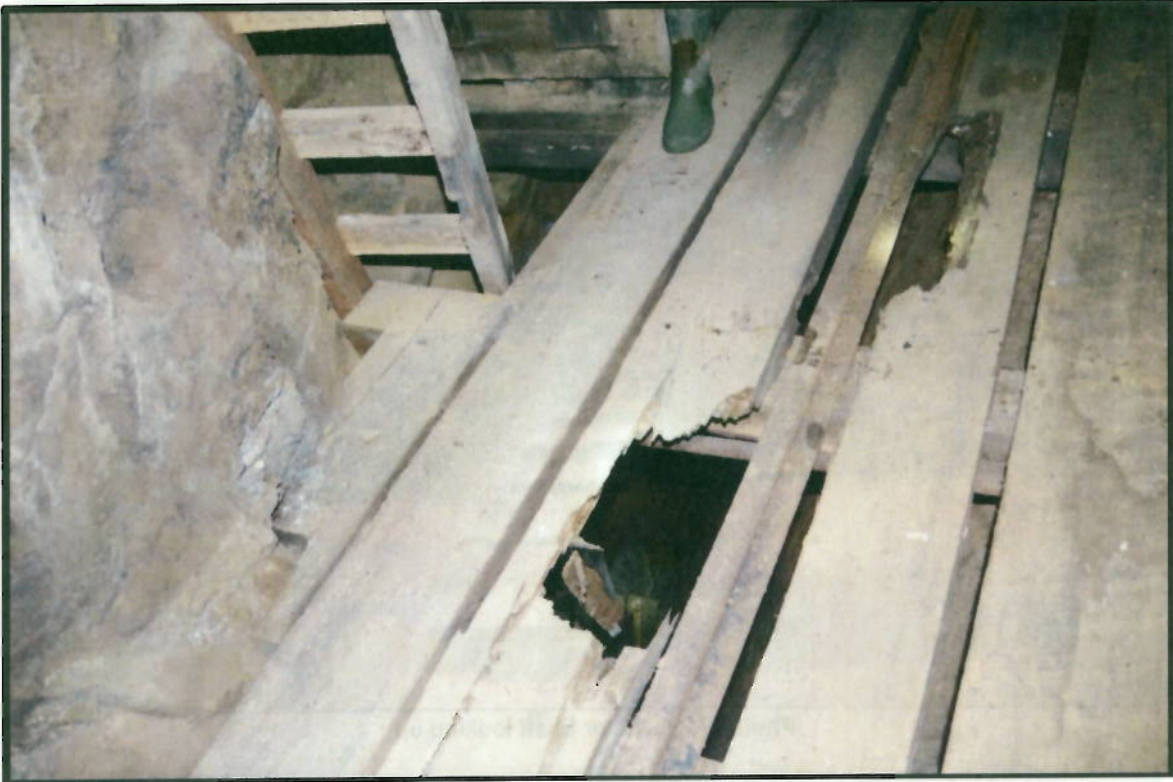
Photo 17: Daylight Winze with rotten wood cover
