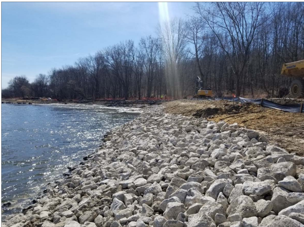
Photo 48: BRSA 9 joint planting riprap (March 2018).
