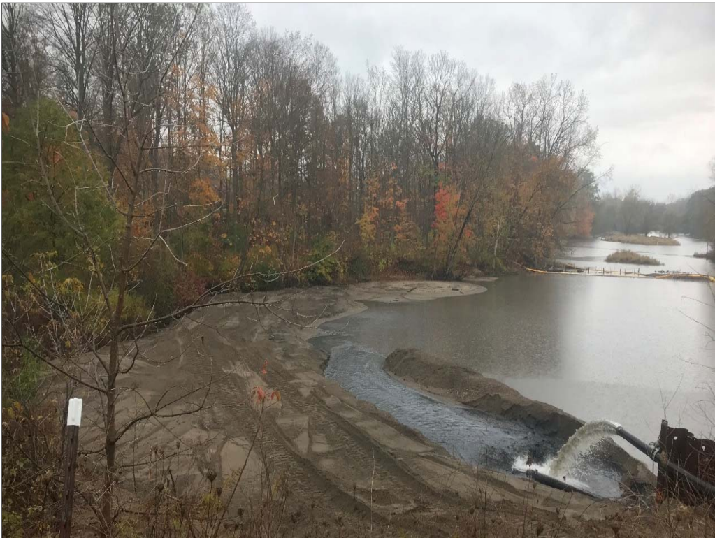
Photo 38: Dredge material filling left descending bank of plunge pool (December 2017).
