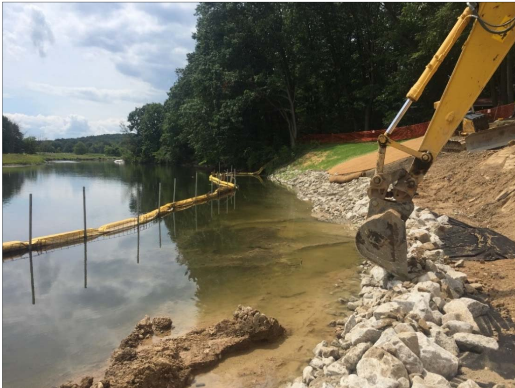
Photo 24: Reinforced turbidity curtain at stream tube 17D (BRSA 4, August 2017).
