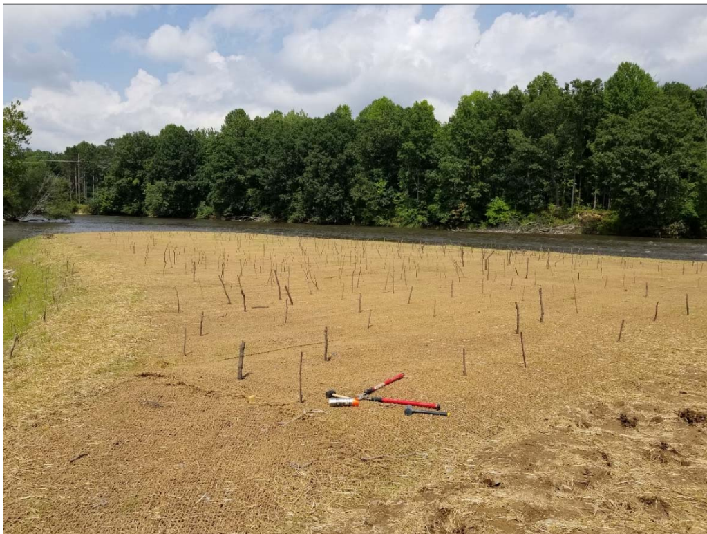
Photo 54: Live stake planting (peninsula between former WCS corridor and plunge pool, August 2018).
