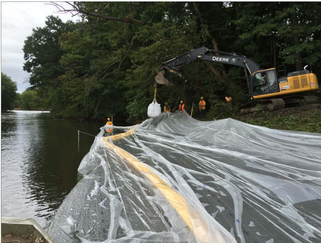
Photo 10: Installation of sandbag cofferdam (BRSA 1, September 2016).
