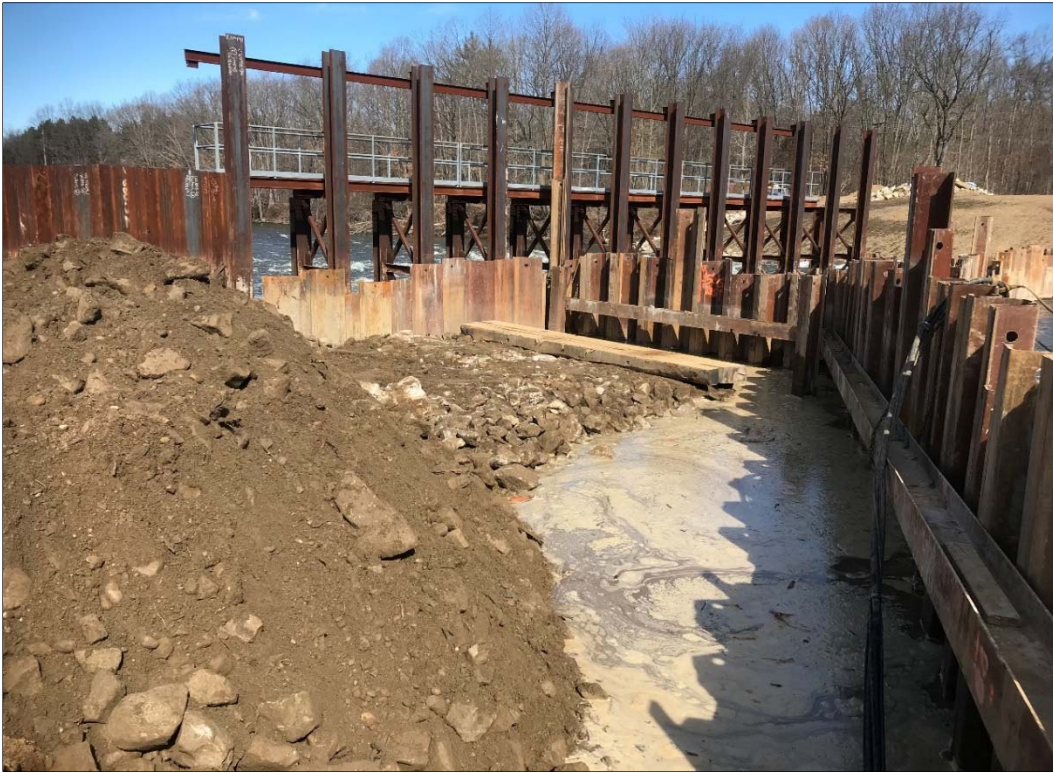
Photo 51: Construction of crane pad for removal of southern portion former WCS (March 2018).
