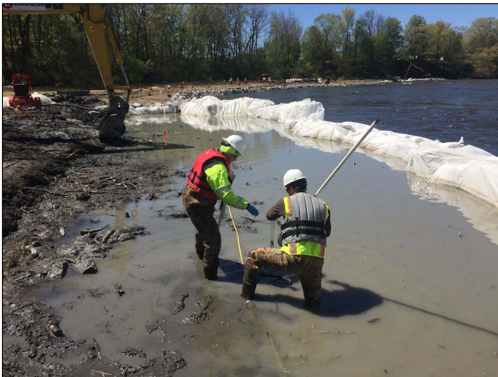
Photo 4: Collecting post-excavation confirmation sample (May 2017)
