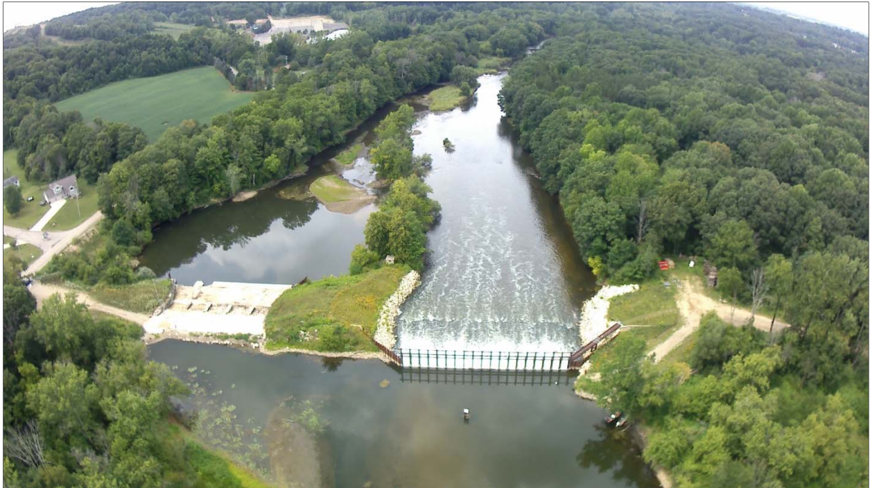
Photo 55: View of former WCS and former auxiliary spillway prior to removal, looking downstream.
