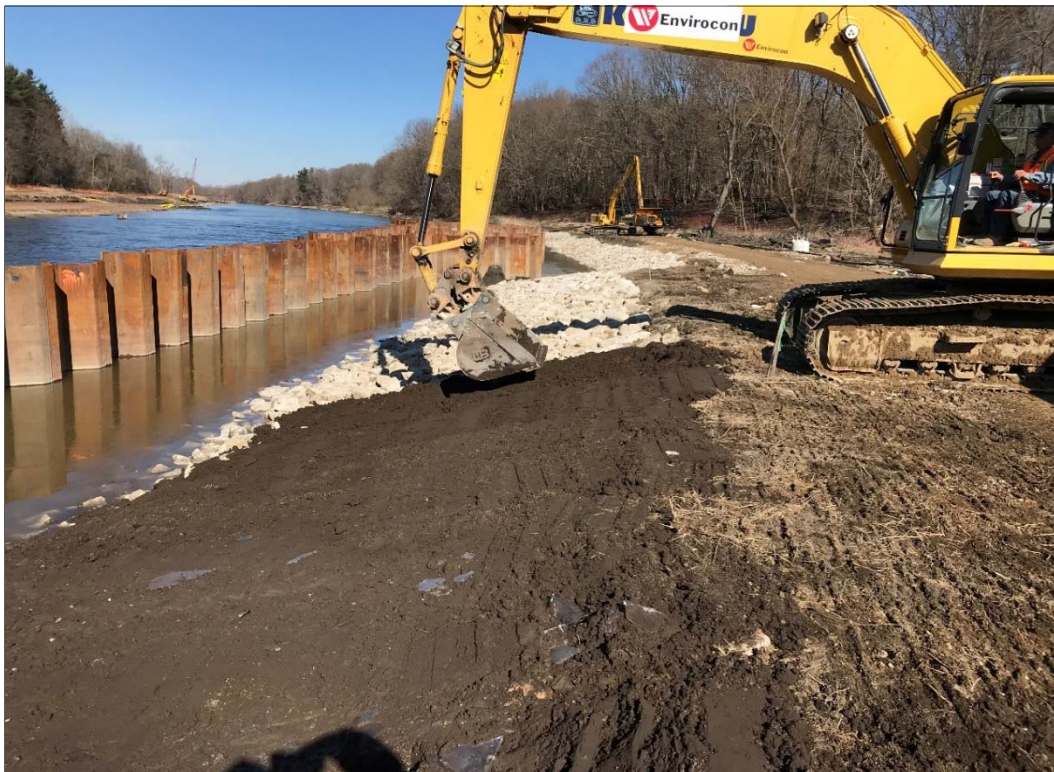
Photo 34: Topsoil placed over joint planting rock during BRSA 7 restoration (March 2018).
