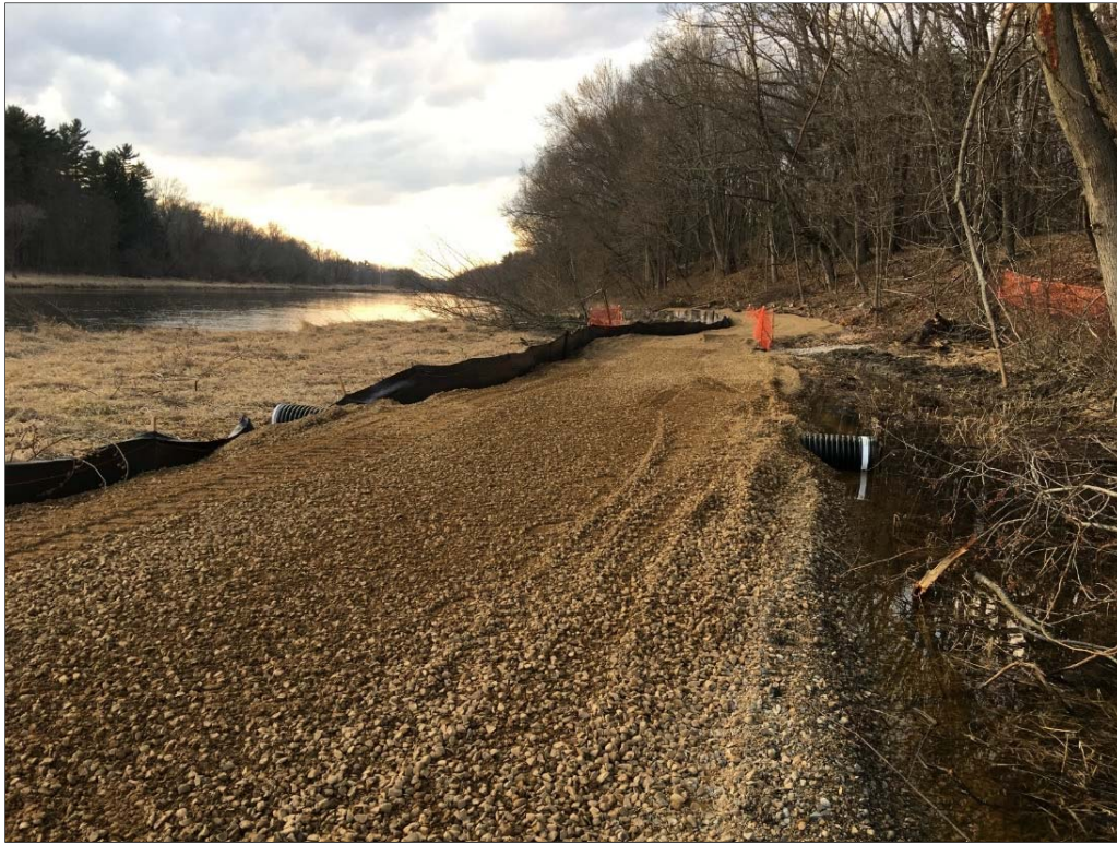
Photo 27: Culvert installed beneath BRSA 6 access road for feeder stream flow (February 2017).
