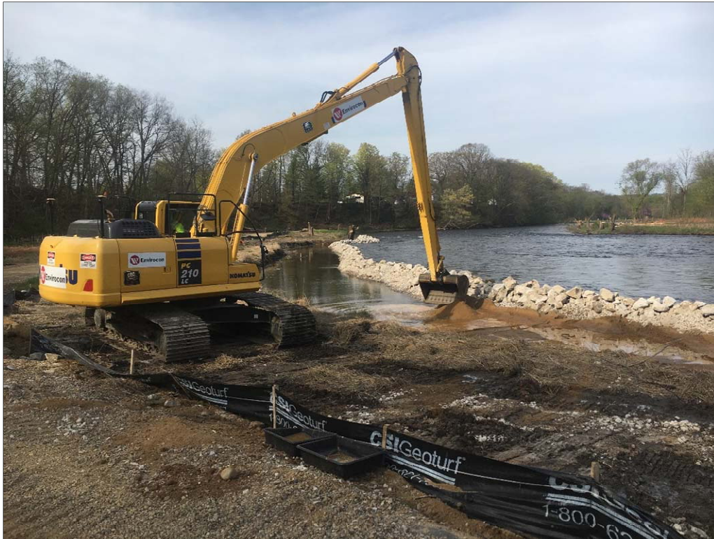
Photo 17: BRSA 3 riprap cofferdam (April 2017).
