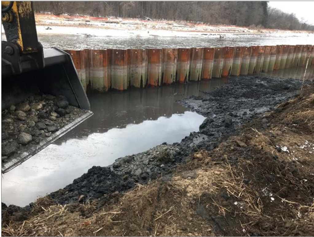
Photo 33: BRSA 7 stream tube Grid 8 excavation inside sheet piling cofferdam (December 2017).
