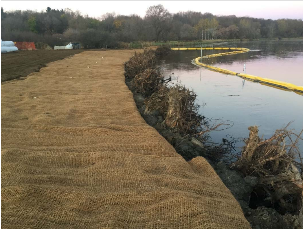
Photo 13: Coir fabric installed over root wads (BRSA 1, October 2016).
