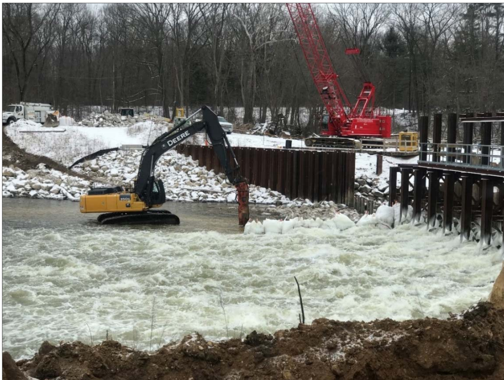
Photo 50: Demolition of grouted riprap during removal of northern half of former WCS (January 2018).
