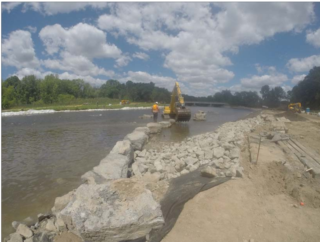
Photo 18: Installation of BRSA 3 J-hook (June 2017).
