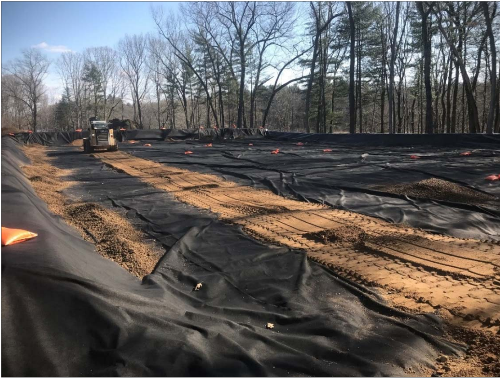
Photo 35: Construction of BRSA 7 stabilization/load out pad at Command Center (April 2018).
