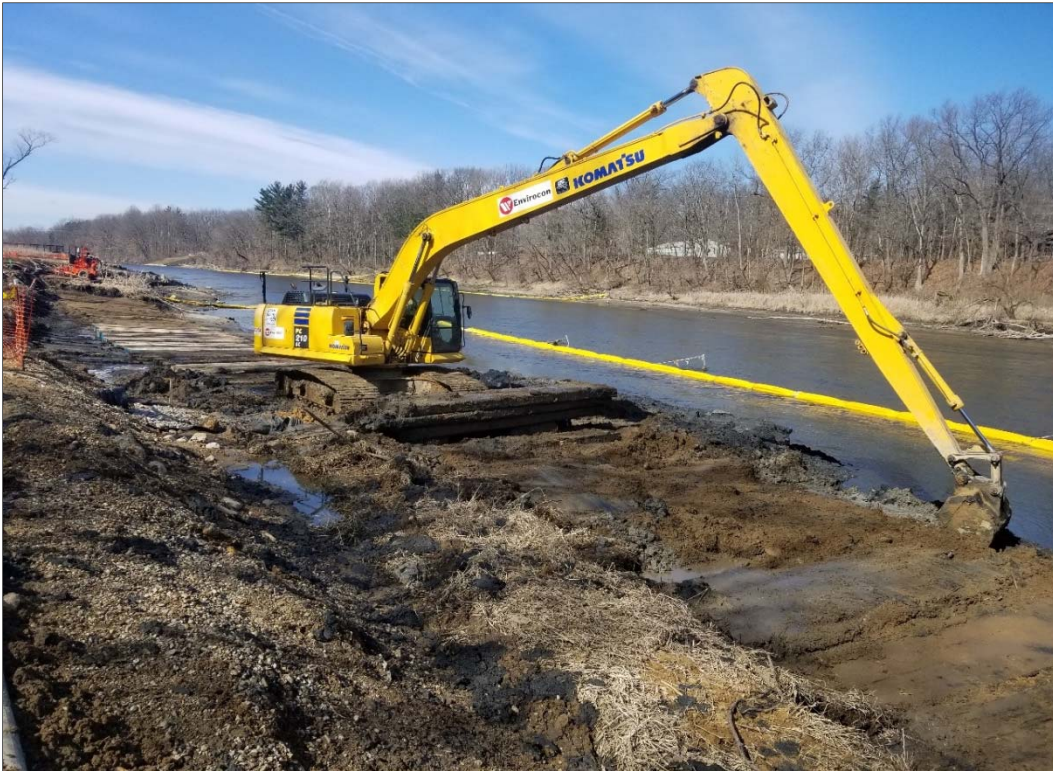
Photo 39: Constructing BRSA 8 bank buildout (March 2018).
