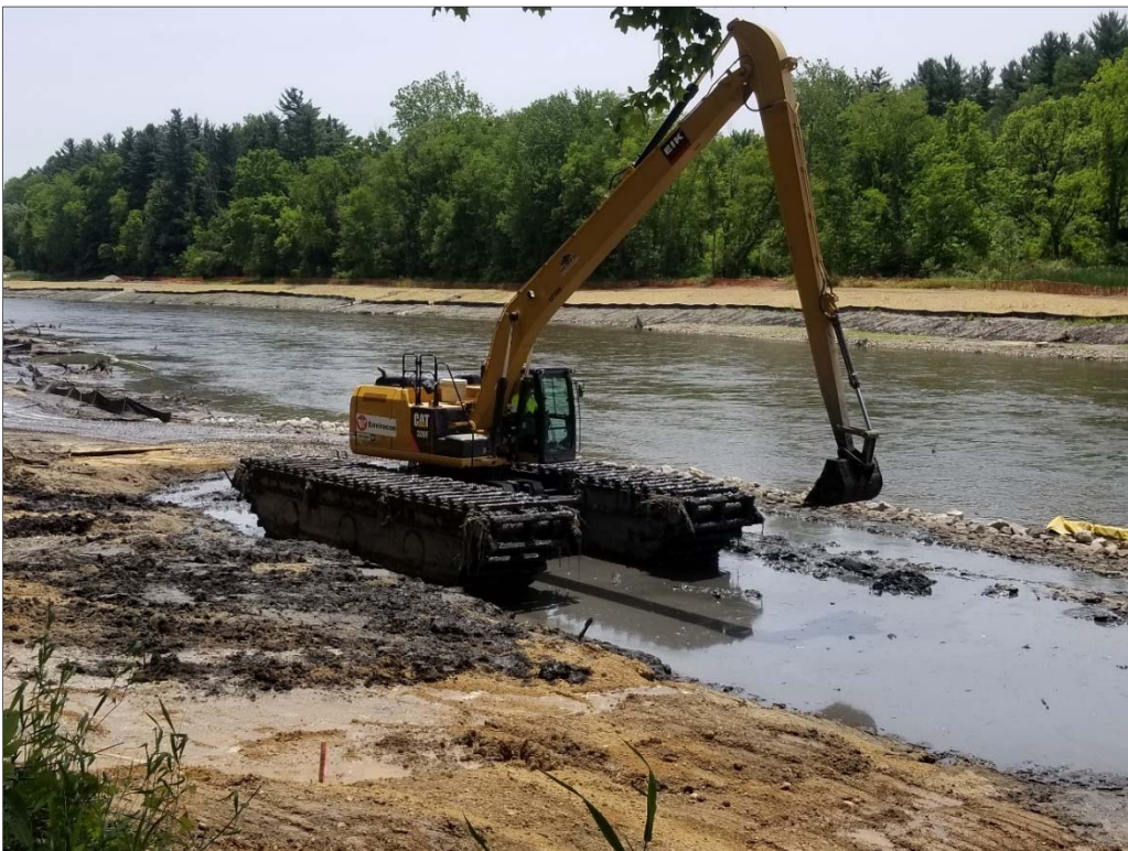
Photo 36: Marsh excavator used during BRSA 7 and 8 construction (June 2018).
