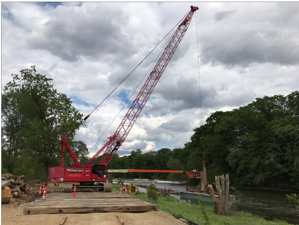
Photo 22: Installing sheet pile cofferdam at stream tube 22C (BRSA 4, May 2017).
