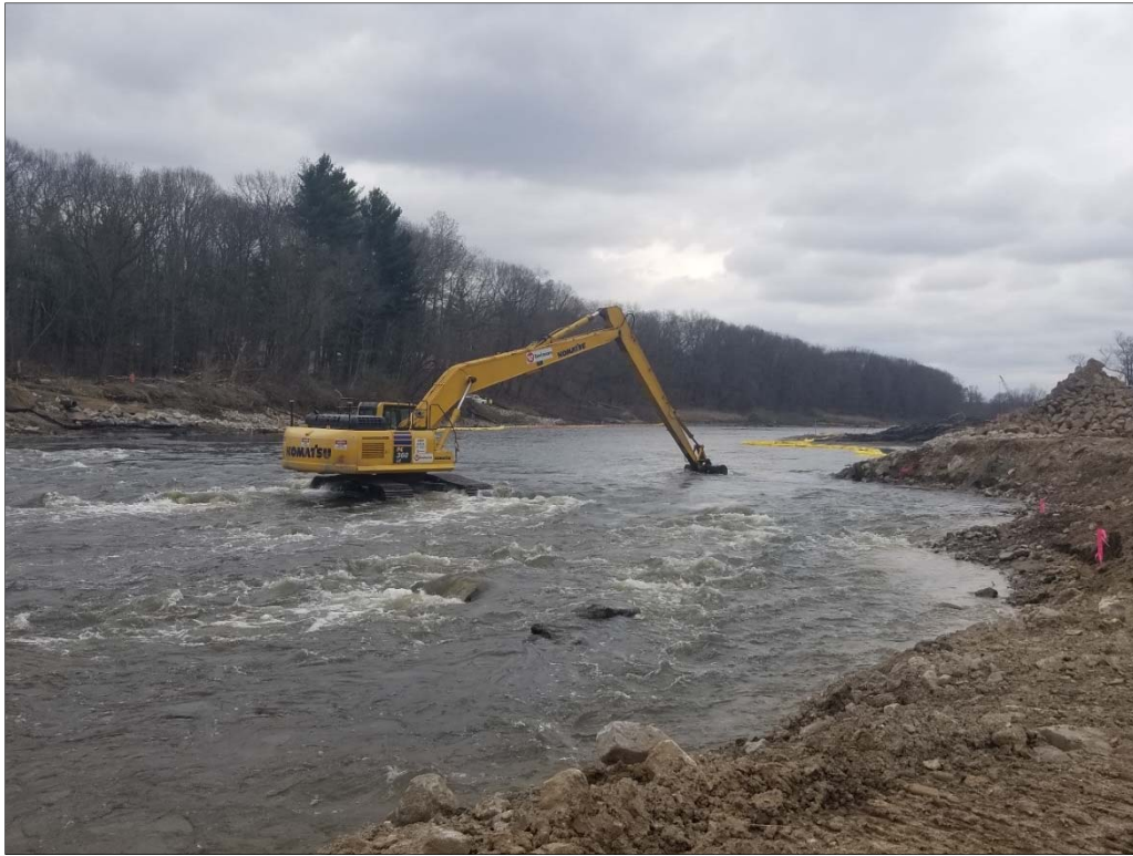
Photo 53: Excavator grading 2% riverbed slope (former WCS corridor restoration, April 2018).
