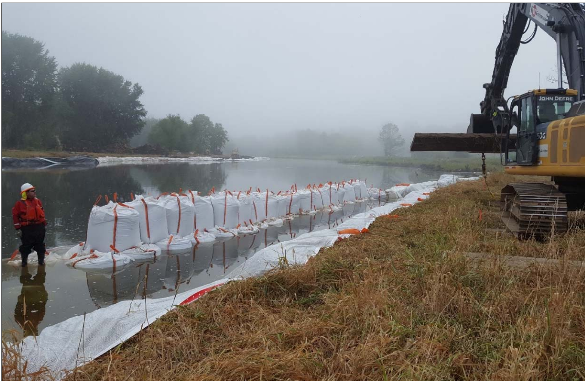
Photo 44: BRSA 9 sand bag coffer dam installation (August 2017).
