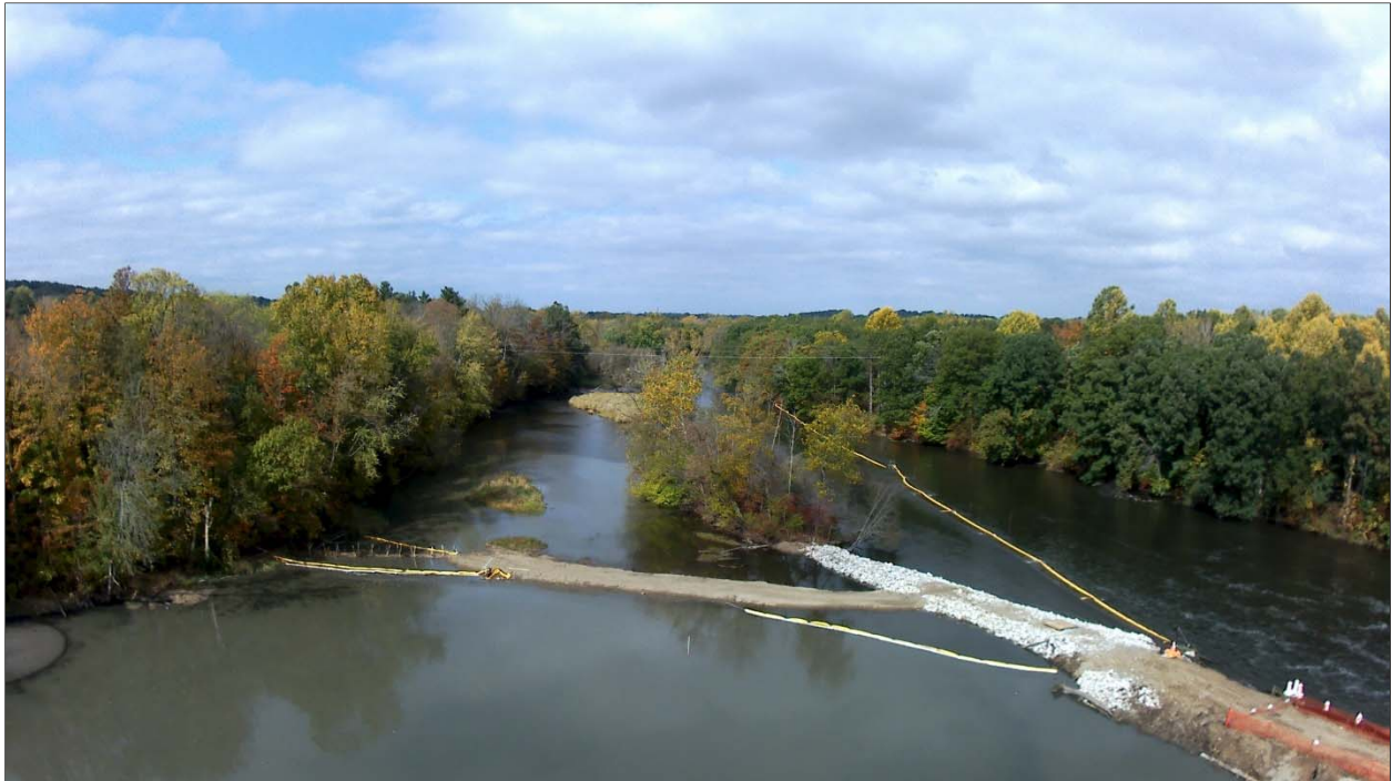
Photo 31: Turbidity controls installed downstream of former WCS and plunge pool during pilot channel dredging (September 2017).
