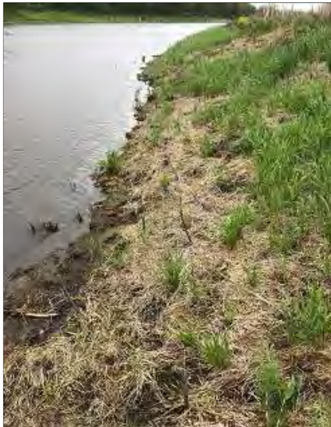
Photo 24: Approx. 20 ft. of BRSA 8 bank with no signs of growth on live stakes.
