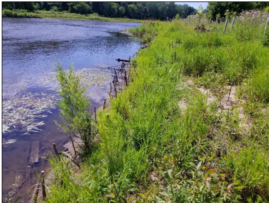
Photo 6B (After): BRSA 6 near RS 48+00, additional live stakes planted in area of low-growth (July 2019).
