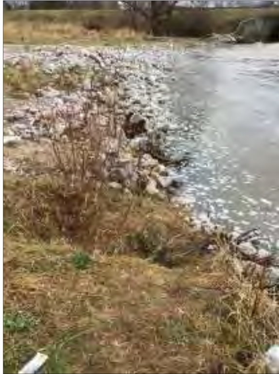
Photo 3: BRSA 1 along RDB of Pine Creek confluence. Void observed below coir fabric at rootwad/joint planting transition (same location as Photo 2).
