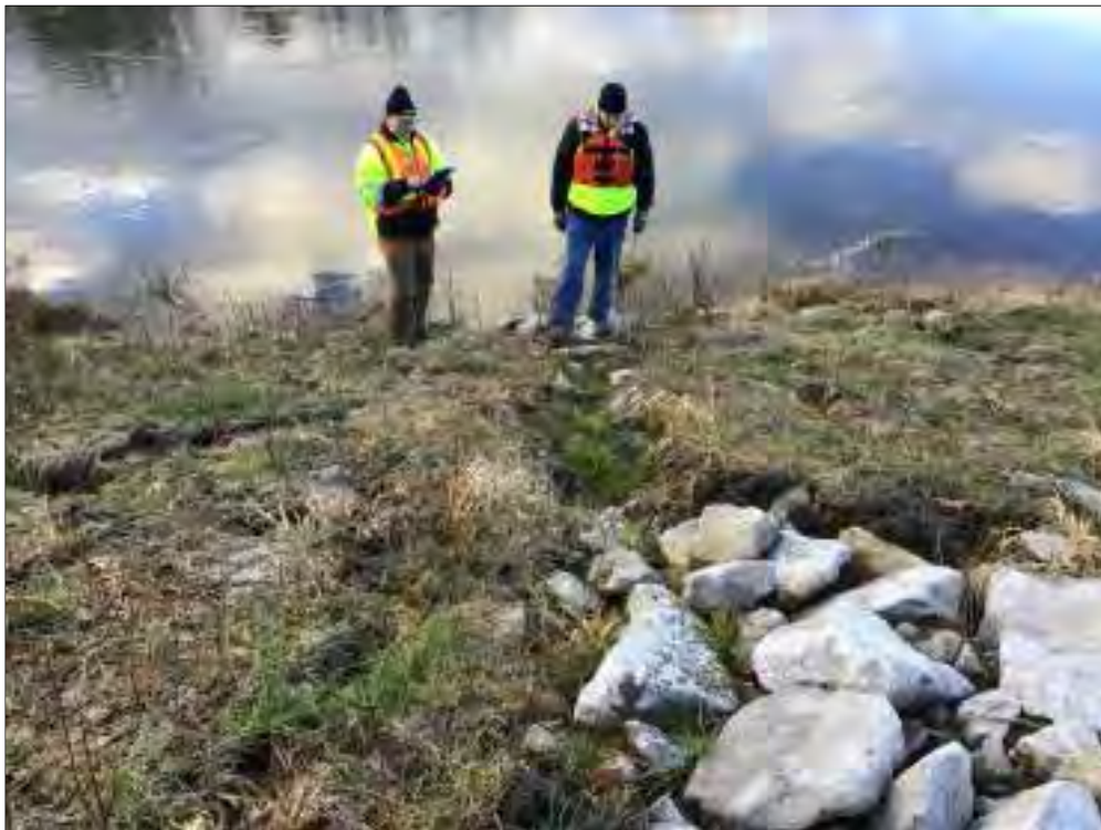
Photo 28: Approx. 8 lineal feet (perpendicular to river) of erosion observed at drainage area on RDB of former water control structure (WCS) corridor.
