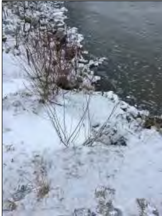
Photo 1: BRSA 1 along right-descending bank (RDB) of Pine Creek confluence. Void observed below coir fabric at rootwad/joint planting transition. No new erosion observed since first quarterly inspection.
