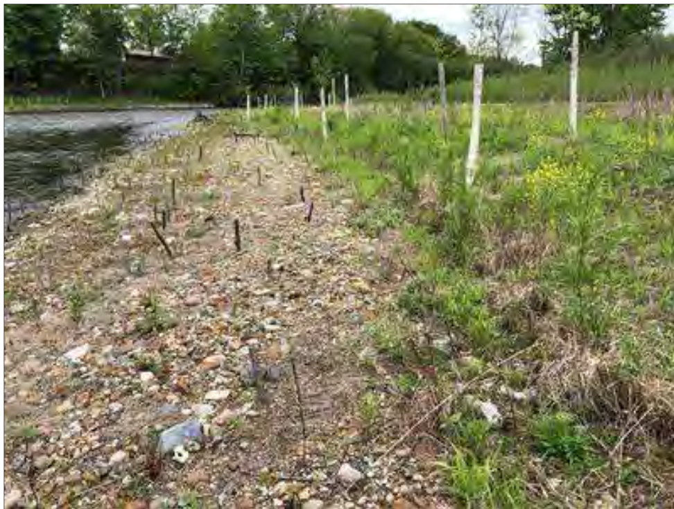
Photo 14: BRSA 4 live stakes do not appear to be growing in area where mid-channel bar material was placed; live stakes are growing higher on bank.
