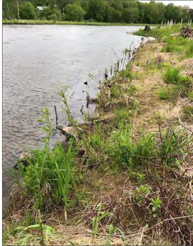
Photo 6A (Before): BRSA 6 near RS 48+00, area of low-growth on live stakes along approximately 50 LF (May 2019).
