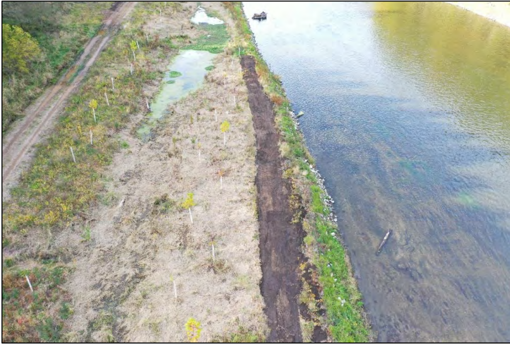
Photo 13: BRSA 8 near RS 26+50, topsoil, seed, and straw placed at top of bank in area of sparse vegetation. Repaired at the request of MDNR during October repair activities (October 2019).
