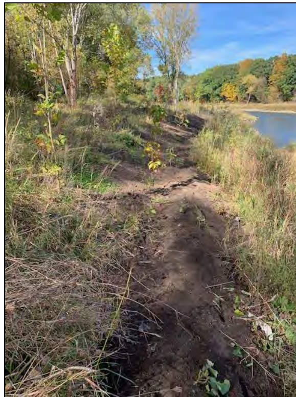
Photo 16B (After): BRSA 9 near RS 34+00, coir fabric repair (October 2019).
