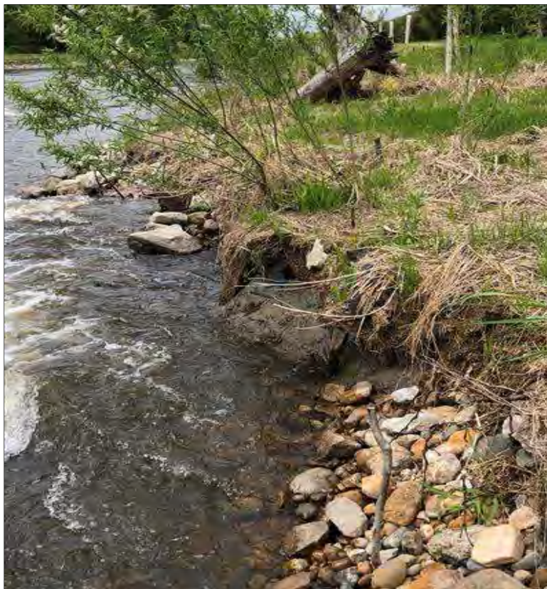
Photo 18: Approx. 75-100 linear feet of scouring along BRSA 6 bank.
