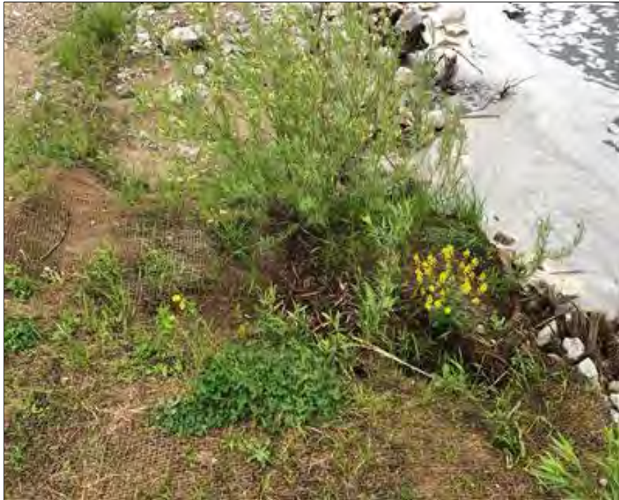
Photo 1A (Before): BRSA 1 near RS 50+00, along the right-descending bank (RDB) of the Pine Creek confluence. Void observed below coir fabric at rootwad/joint planting transition (May 2019).
