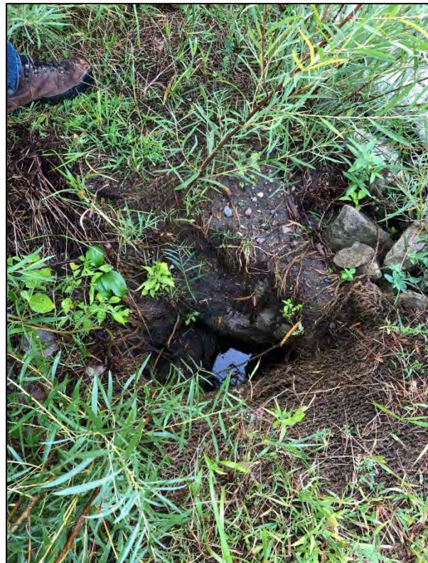
Photo 2: BRSA 1 right-descending bank of Pine Creek confluence. Void observed at rootwad/joint planting transition (observed during previous inspections).
