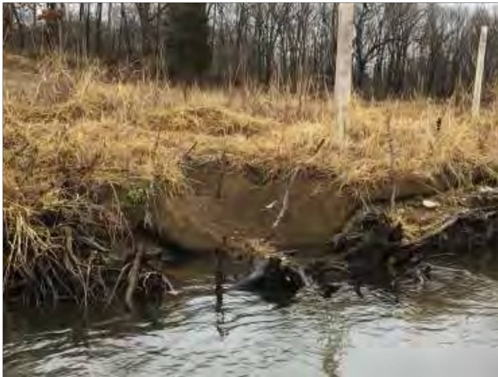
Photo 8: Area of settling observed on BRSA 4 bank, downstream of staging area (approx. 120 feet upstream of location in Photo 7).
