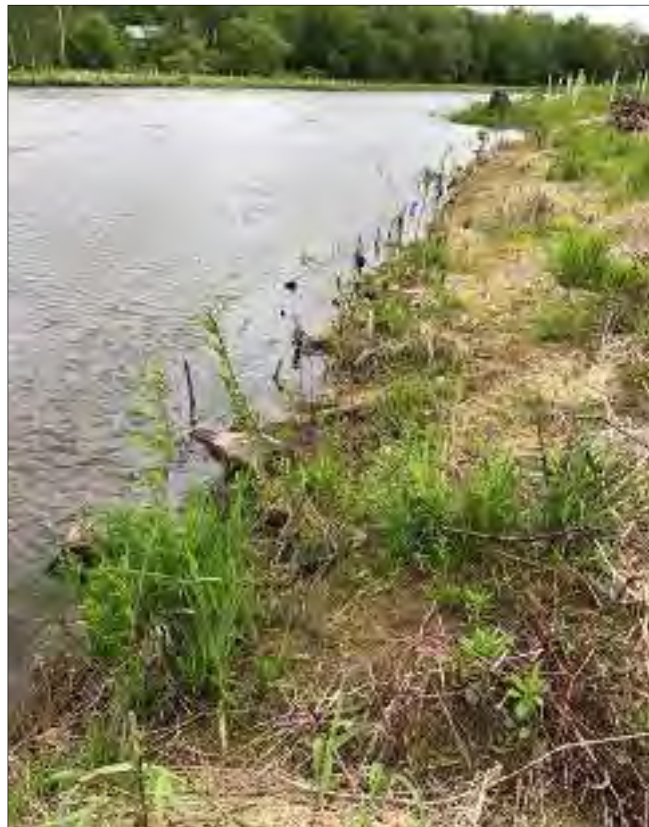
Photo 16: Approx. 50 ft. of BRSA 6 with low-growth on live stakes. Previously identified, no new issues observed.
