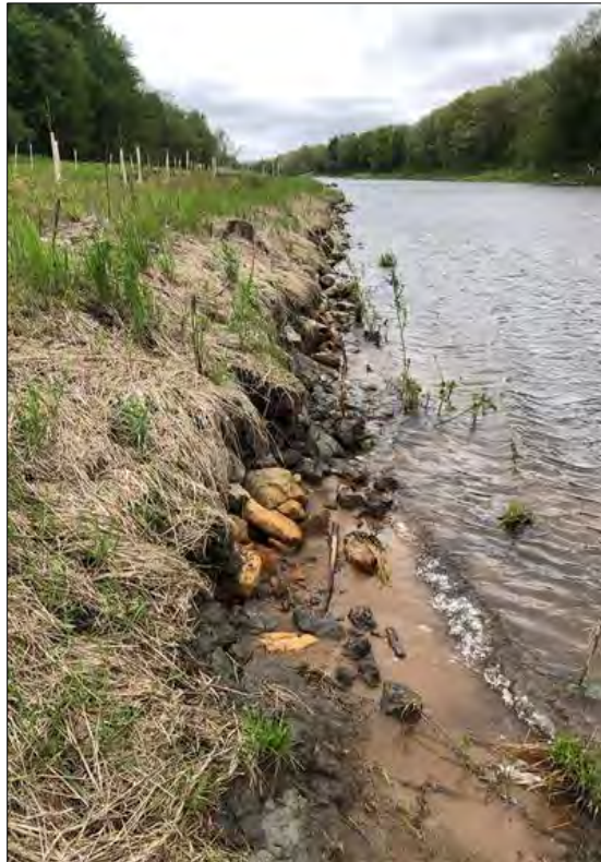
Photo 9A (Before): BRSA 8 starting near RS 24+75, area of scouring observed along approximately 300-400 LF of bank (May 2019).
