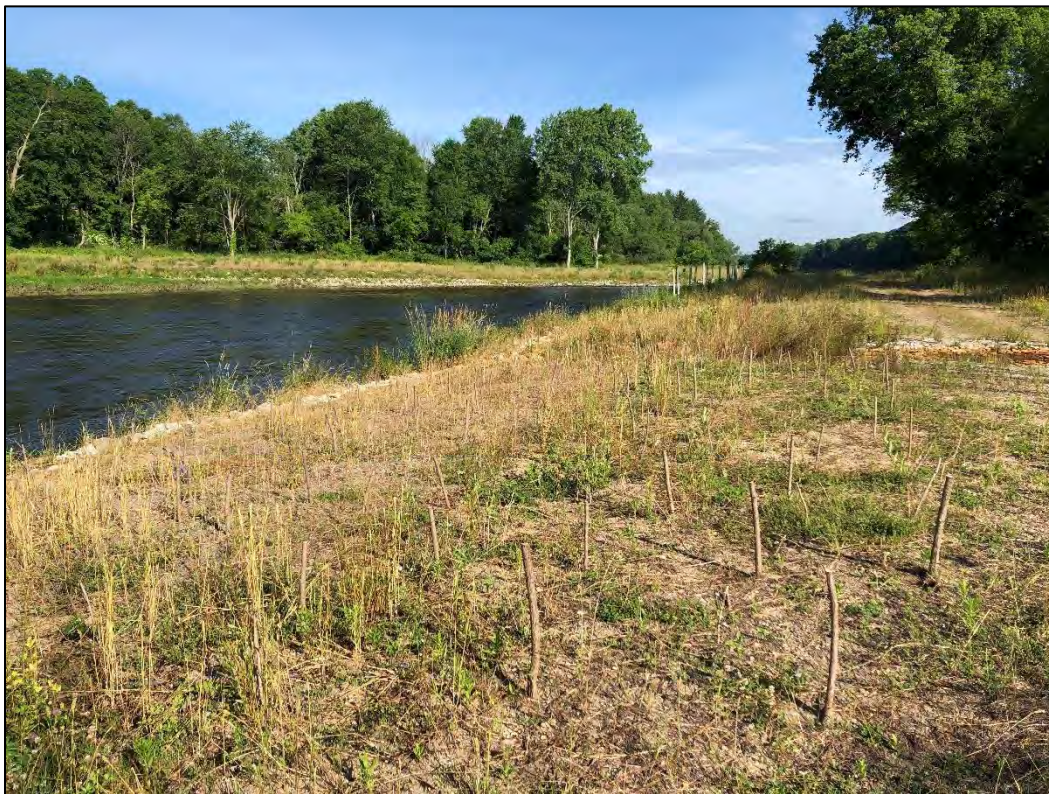
Photo 7B (After): BRSA 6 near RS 37+00 (oxbow discharge area), additional live stakes planted in area of no growth (July 2019).
