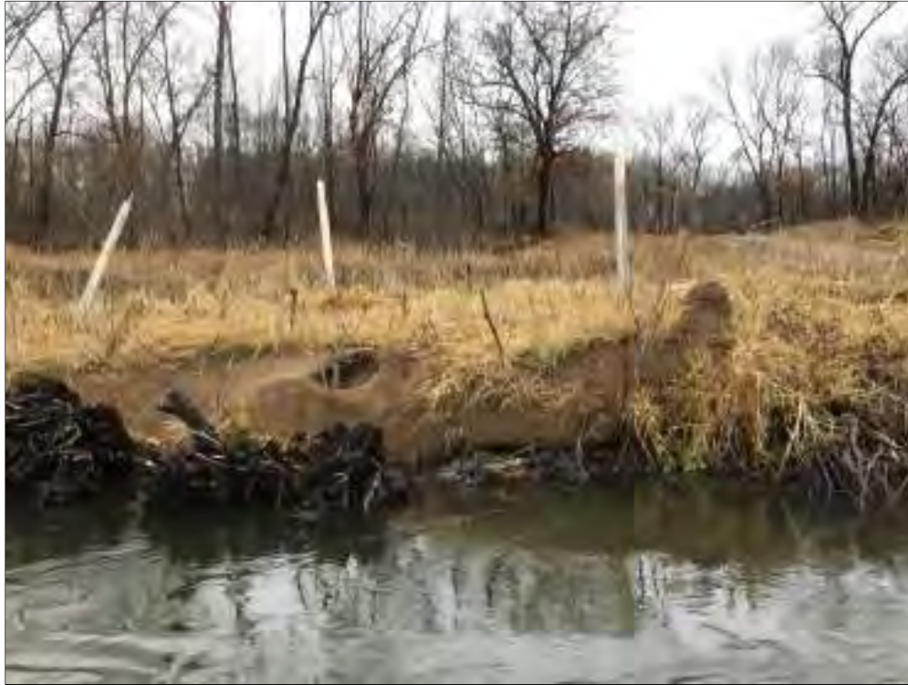
Photo 7: Area of settling observed along approx. 32 lineal feet of BRSA 4 bank, downstream of staging area.
