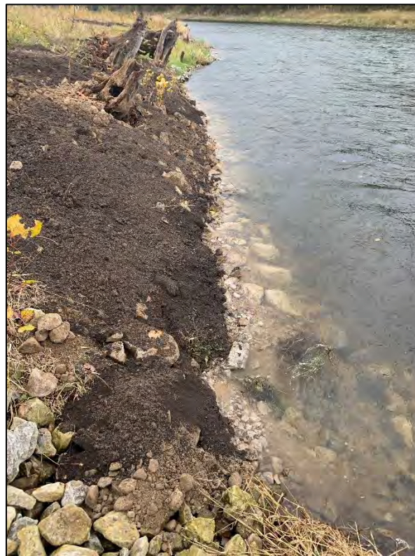
Photo 14: BRSA 8 near RS 32+00, erosion observed during October 2019 repairs. Repaired at the request of MDNR by installing riprap, common fill, topsoil, seed, and live stakes (October 2019).
