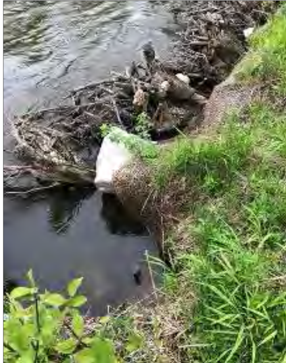
Photo 13: BRSA 4 area of sloughing observed across from BRSA 3 J-hooks during 1st and 2nd Quarterly Inspections. No new issues observed.
