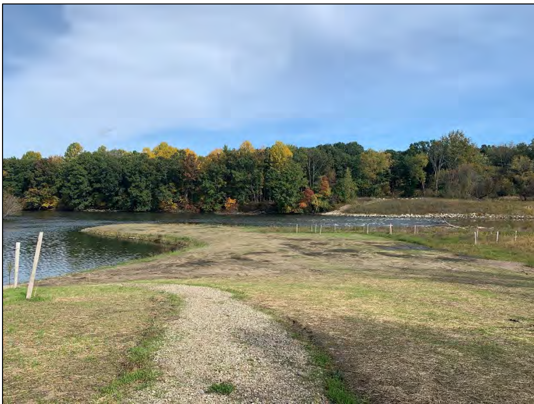
Photo 17B (After): Plunge Pool near 0+00, new topsoil and seed installed (October 2019).
