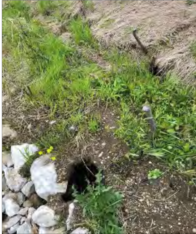
Photo 19: Hole observed in BRSA 6 bank, approx. 1 ft. deep, extending landward approx. 3 ft. Continue to monitor.
