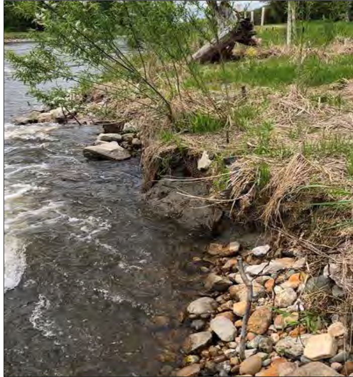
Photo5A (Before): BRSA 6 near RS 38+50, bank scour along approximately 75-100 linear feet (LF) of bank (May 2019).
