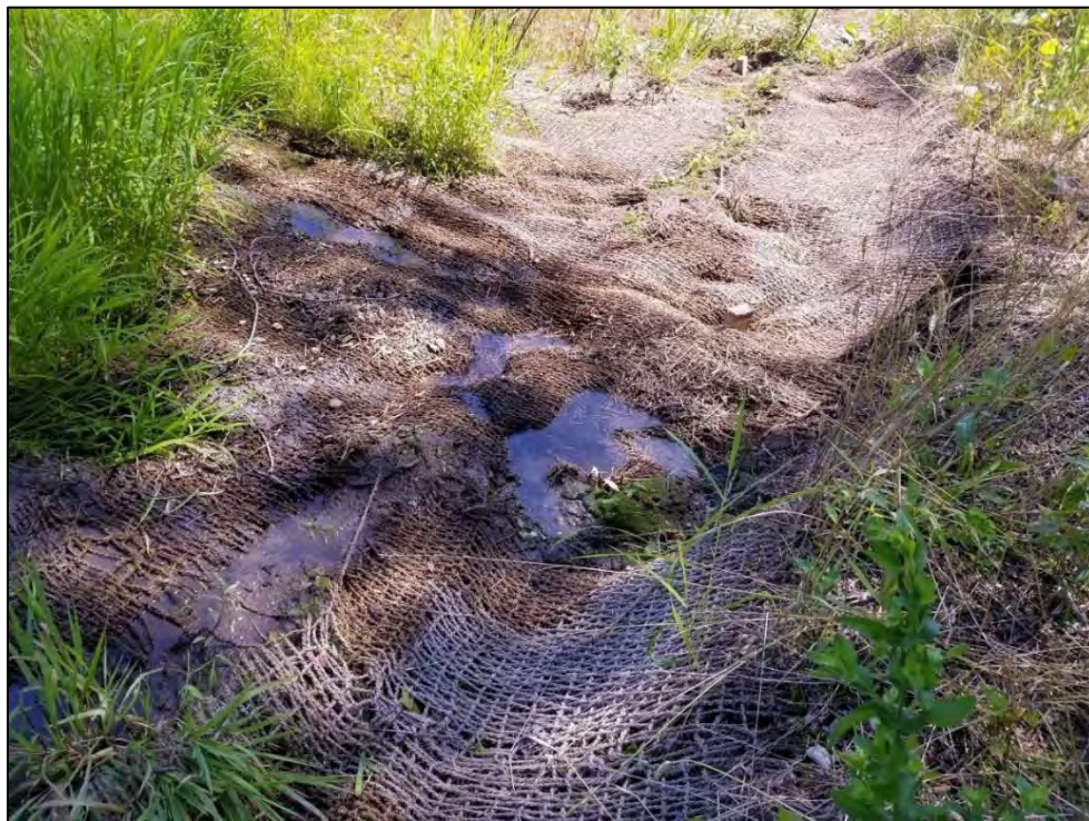
Photo 15B (After): BRSA 9 near RS 36+00, area of coir fabric repair (July 2019).
