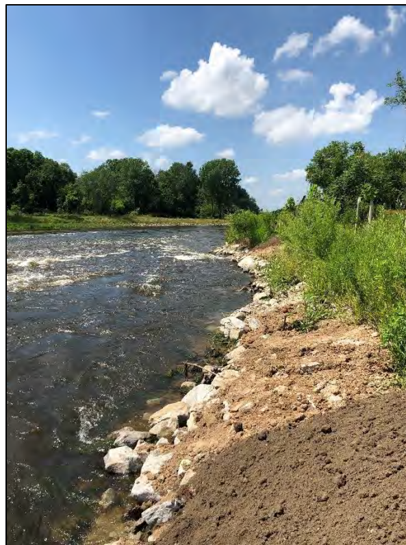
Photo 5B (After): BRSA 6 near RS 38+50, bank scour repair (July 2019).
