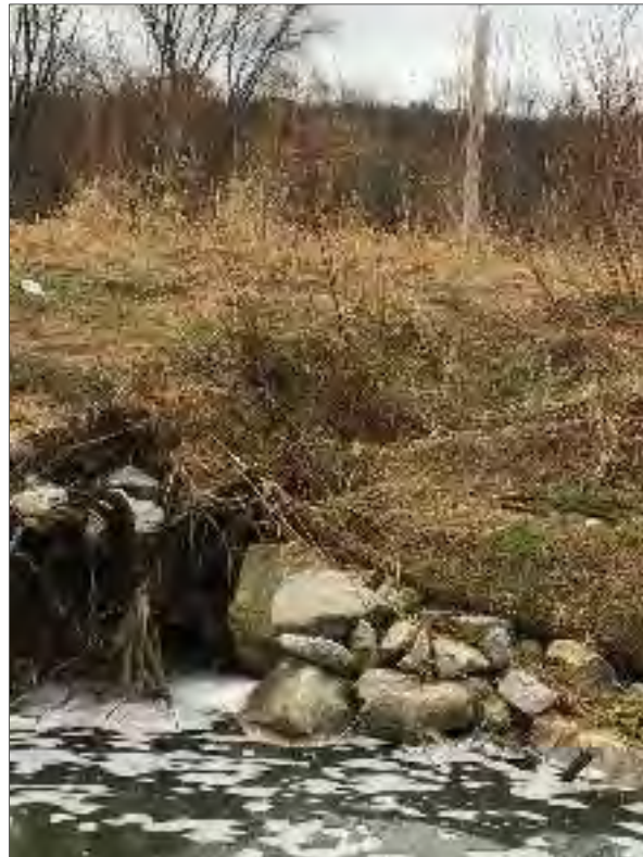
Photo 2: BRSA 1 along right-descending bank (RDB) of Pine Creek confluence. Void observed below coir fabric at rootwad/joint planting transition. Void measures approx. 2 ft. deep by 3 ft. parallel to river by 6 ft. perpendicular to river.
