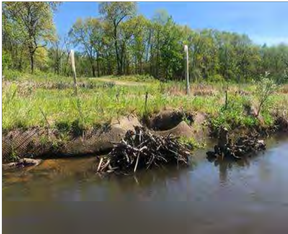
Photo 12: Boat-based view of BRSA 4 area of sloughing observed during 1st and 2nd Quarterly Inspections.
