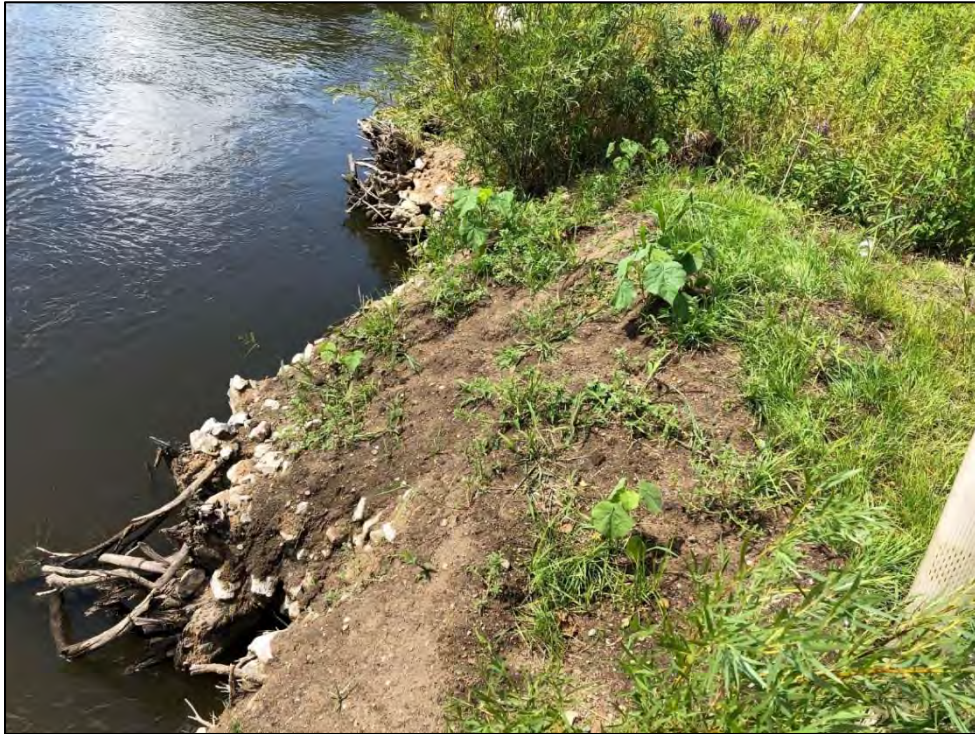
Photo 9: BRSA 4 bank repair area (repair completed July 2019), no live stakes were installed as part of the repair.
