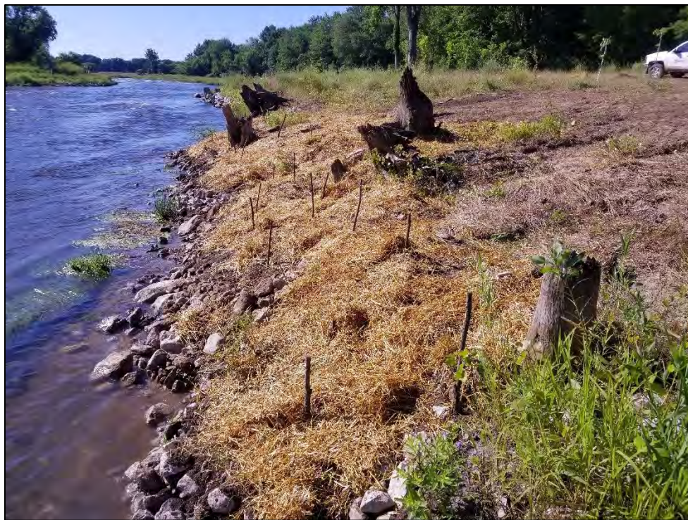
Photo 9B (After): BRSA 8 near RS 27+00, area of scouring bank repair (July 2019).
