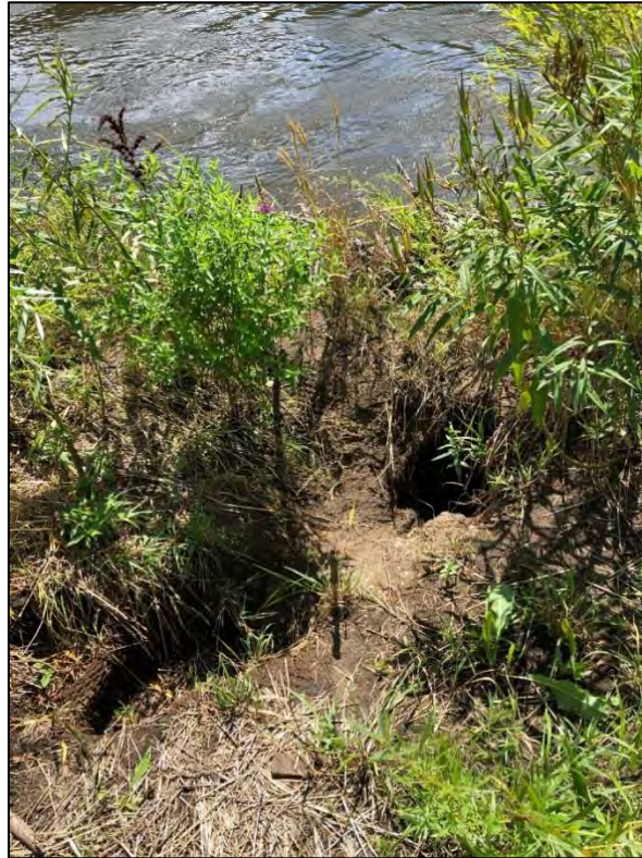
Photo 3A (Before): BRSA 4 near RS 71+50, area of erosion approximately 25-50 feet upstream of July 2019 repairs (August 2019).
