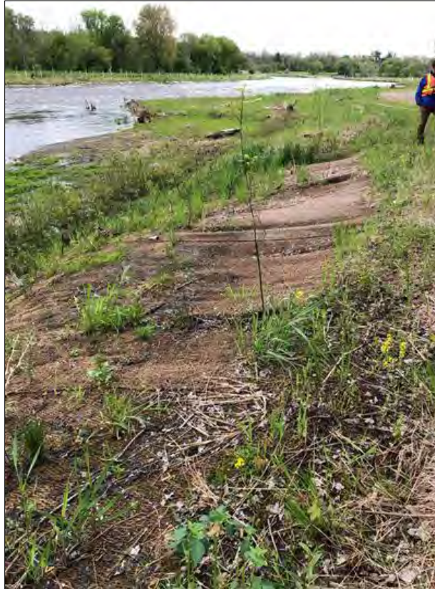
Photo 15A (Before): BRSA 9 near RS 36+00, void beneath approximately 35 LF of coir fabric observed during Q1 through Q3 inspections (May 2019).
