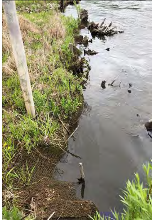
Photo 2A (Before): BRSA 4 near RS 70+00, area of sloughing observed during Q1 through Q3 Inspections (May 2019).
