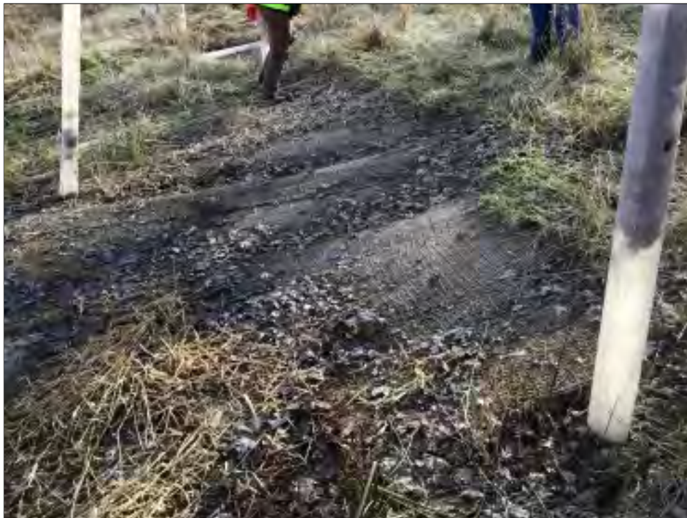
Photo 22: BRSA 9 approaching transition to BRSA 8, coir fabric not secure.
