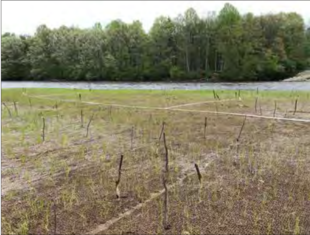
Photo 17A (Before): Plunge Pool near 0+00, general view of peninsula. Limited grass and live stake growth observed (May 2019).
