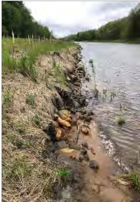
Photo 25: Scour observed along approx. 300-400 linear feet of BRSA 8 bank, beginning near RS 24+75.
