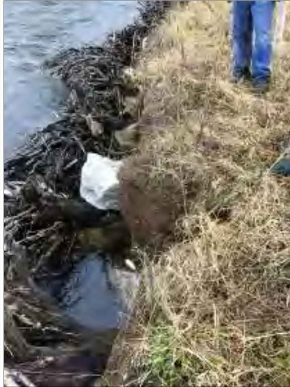
Photo 9: Area of settling observed along approx. 20 lineal feet of BRSA 4 bank, located in root wads across from BRSA 3 J-hooks.
