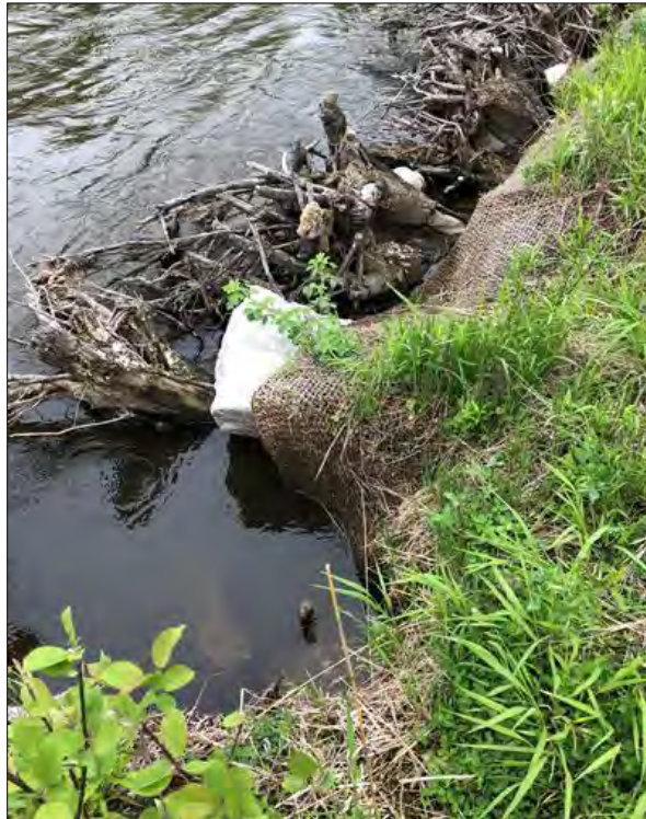
Photo 4A (Before): BRSA 4 near RS 86+00, area of sloughing observed across from BRSA 3 J-hooks during Q1 through Q3 Inspections (May 2019).
