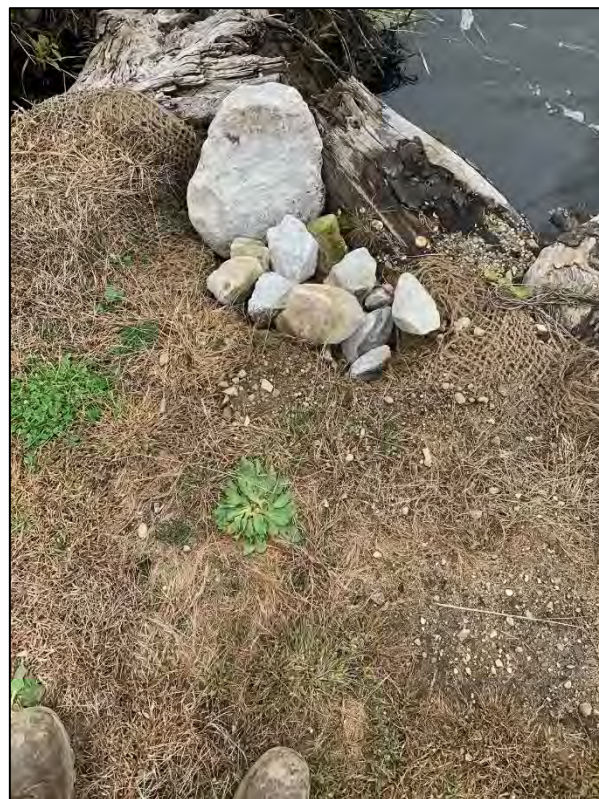
Photo 1B (After): BRSA 1 near RS 50+00, repair of void along RDB of Pine Creek confluence at rootwad/joint planting transition (October 2019).
