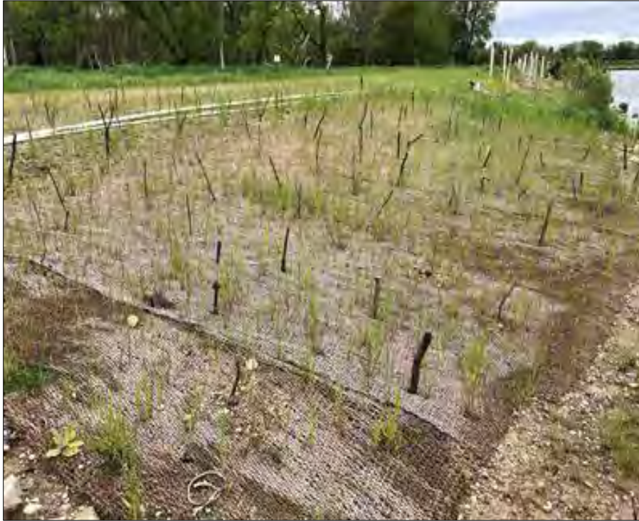
Photo 7A (Before): BRSA 6 near RS 37+00 (oxbow discharge area), live stakes not showing signs of growth (May 2019).
