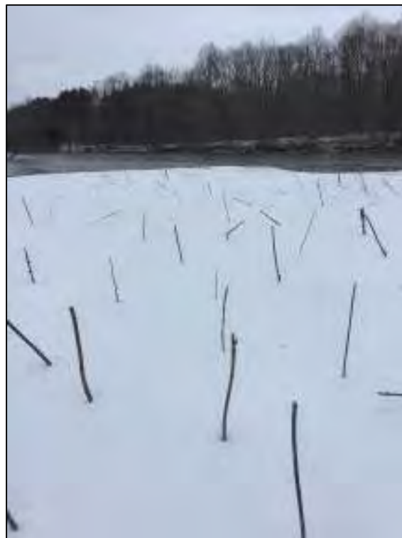
Photo 18: Live stakes knocked down on plunge pool area peninsula.
