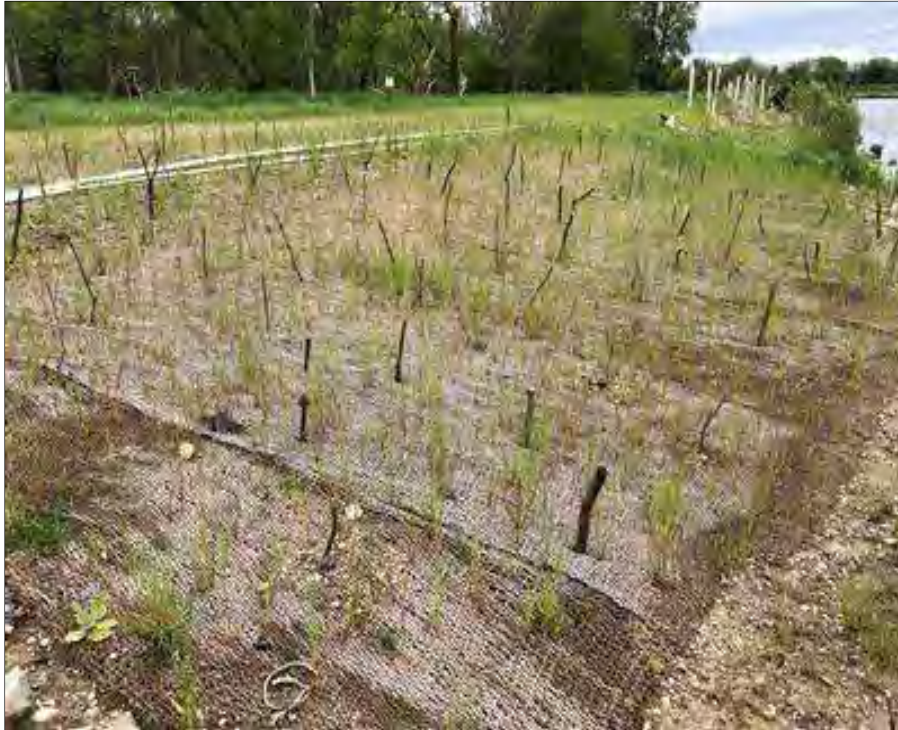
Photo 17: BRSA 6 oxbow discharge area – live stakes not showing signs of growth.
