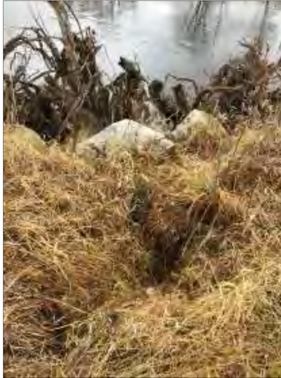
Photo 5: Approx. 10 square feet of surface erosion observed on BRSA 1 bank.
