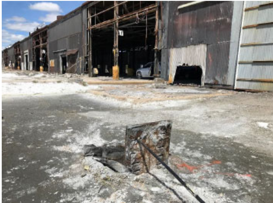
Figure 3: Dilapidated Robertson Siding contaminated with PCBs and asbestos moving to storm drain
