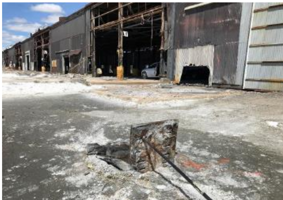
Figure 2: Dilapidated Robertson Siding contaminated with PCBs moving to storm drain.
