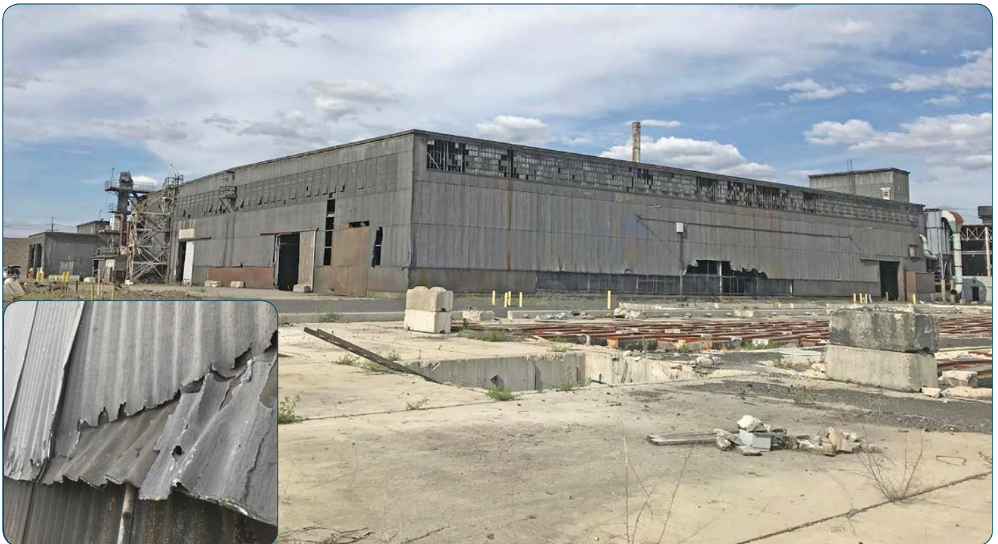
Crews will remove highly contaminated siding (see inset) from a number of on-site buildings.
