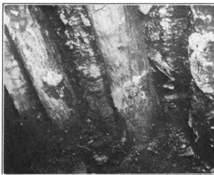
Fungus Growth on Untreated Portion of Mine Timbers. Upper Portion of Timber Treated, Lower Portion Untreated.
