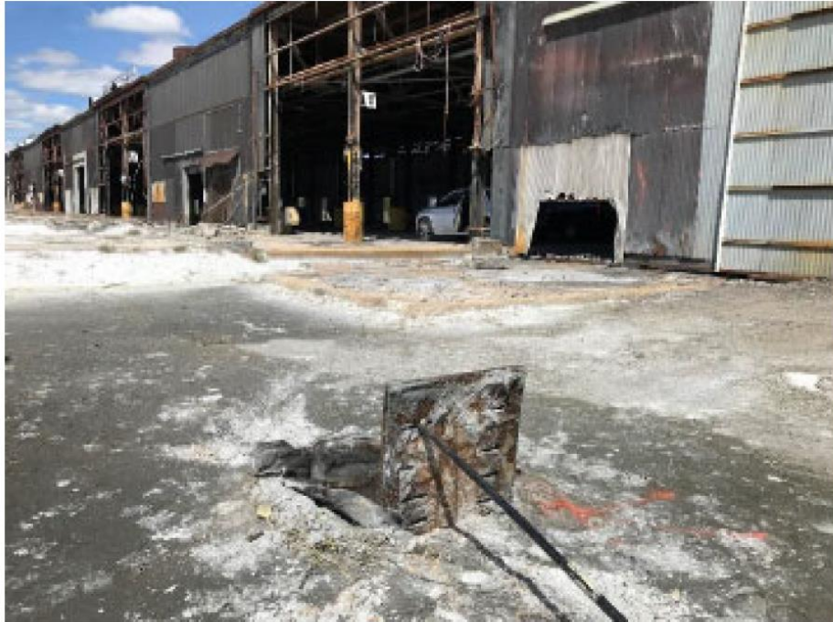
12 Dilapidated Robertson Siding contaminated with PCBs and asbestos moving to storm 13 drain
