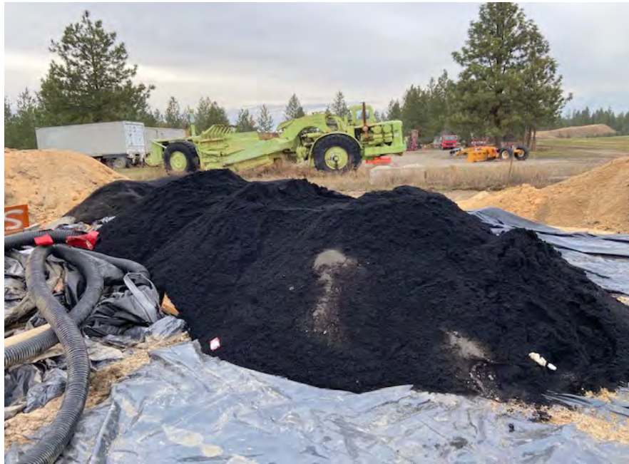
Photograph 29. Stockpiled granulated activated carbon (GAC) from carbon vessels. (November 3, 2020)
