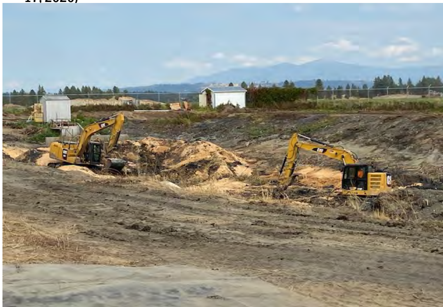
Photograph 11. Clean Harbors mixing wood pellets into lower pond sediment using a track hoe. Soil pad constructed for water treatment system. (September 17, 2020)
