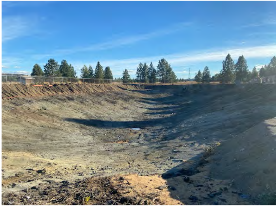
Photograph 23. Sediment removal completed from lower pond. (October 15, 2020)
