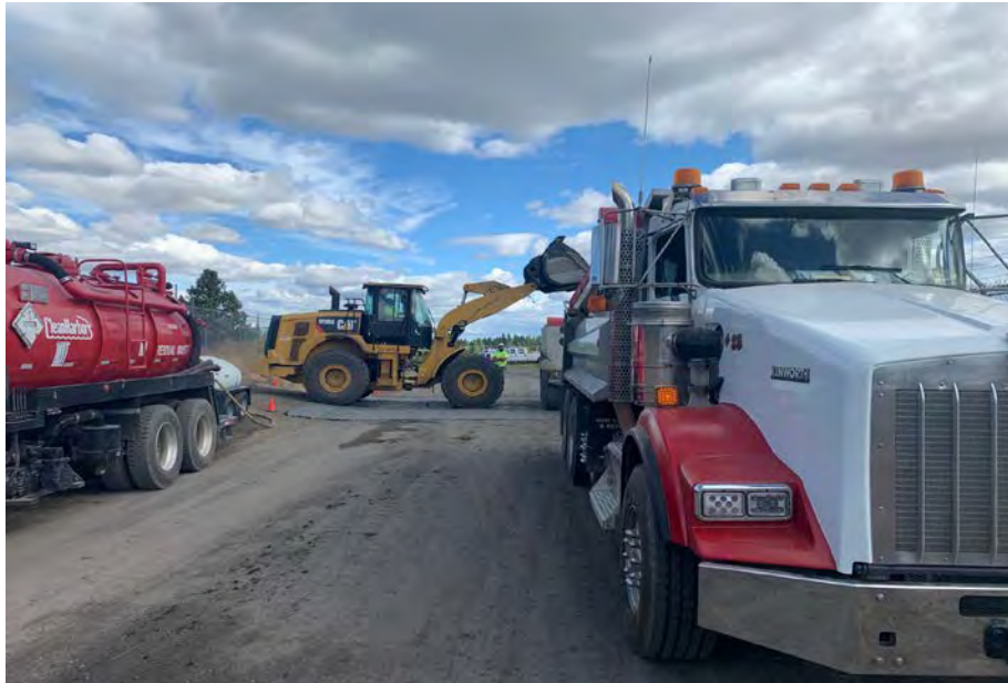
Photograph 3. Clean Harbors loads sediment from upper pond into haul trucks. Drop cloth pictured in roadway. (August 27, 2020)
