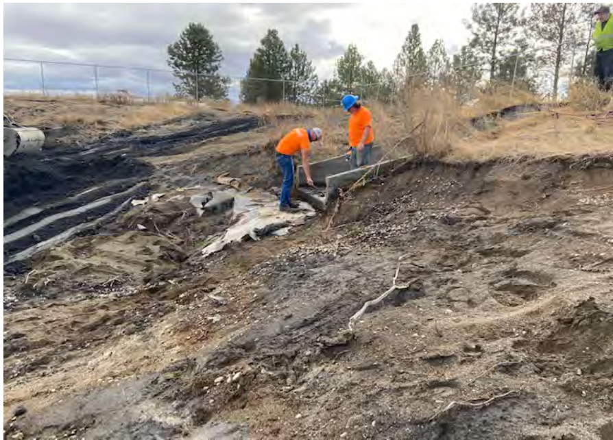
Photograph 21. Steel plate removed at inlet of lower pond. (October 12, 2020)
