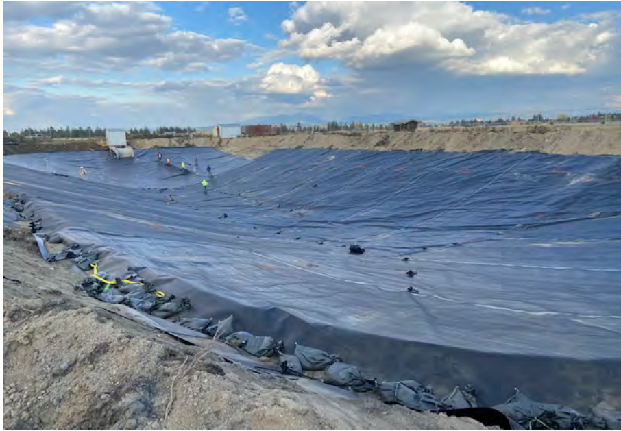
Photograph 27. Geosynthetic liner installation in lower pond. (October 22, 2020)
