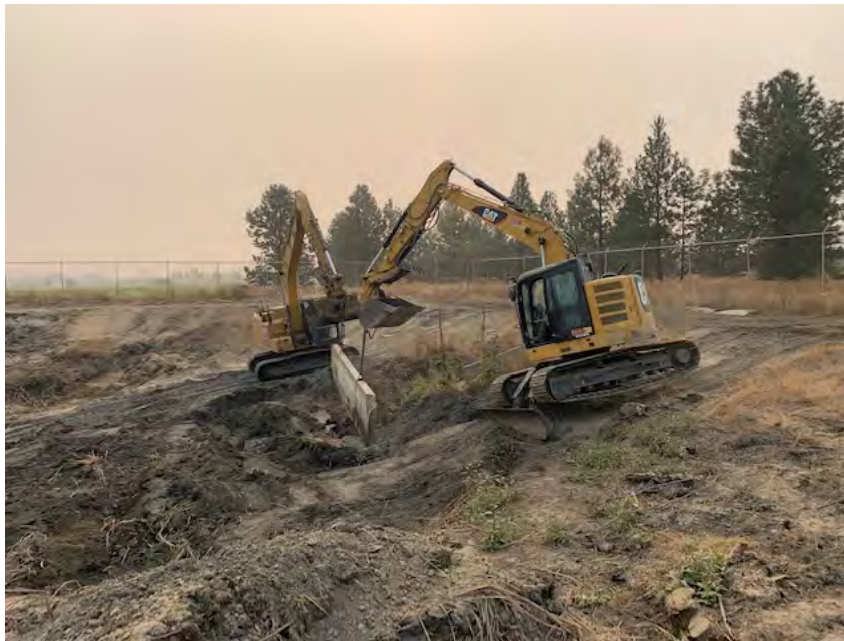
Photograph 21. Steel plate removed at inlet of lower pond. (October 12, 2020)
