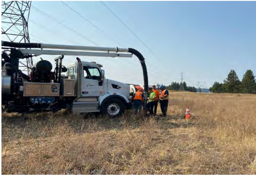
Photograph 15. Clean Harbors conducting cleanout of the conveyance piping at Vault #4. (October 2, 2020)
