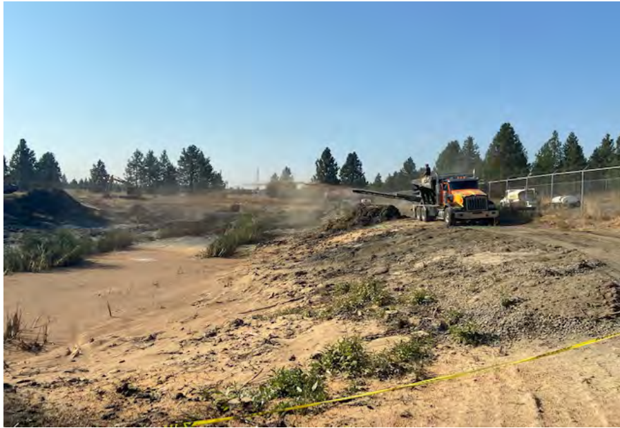
Photograph 9. Conveyor Aggregate Delivery (CAD) truck spreading absorbent wood pellets into the lower pond. (September 11, 2020)
