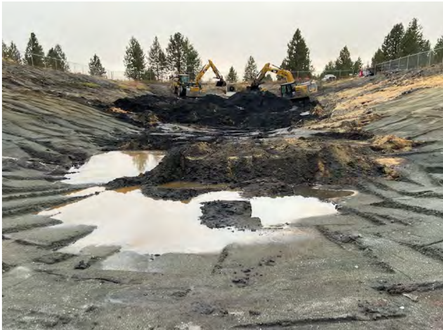
Photograph 14. Clean Harbors removing sediment from the lower pond for disposal. (October 1, 2020)
