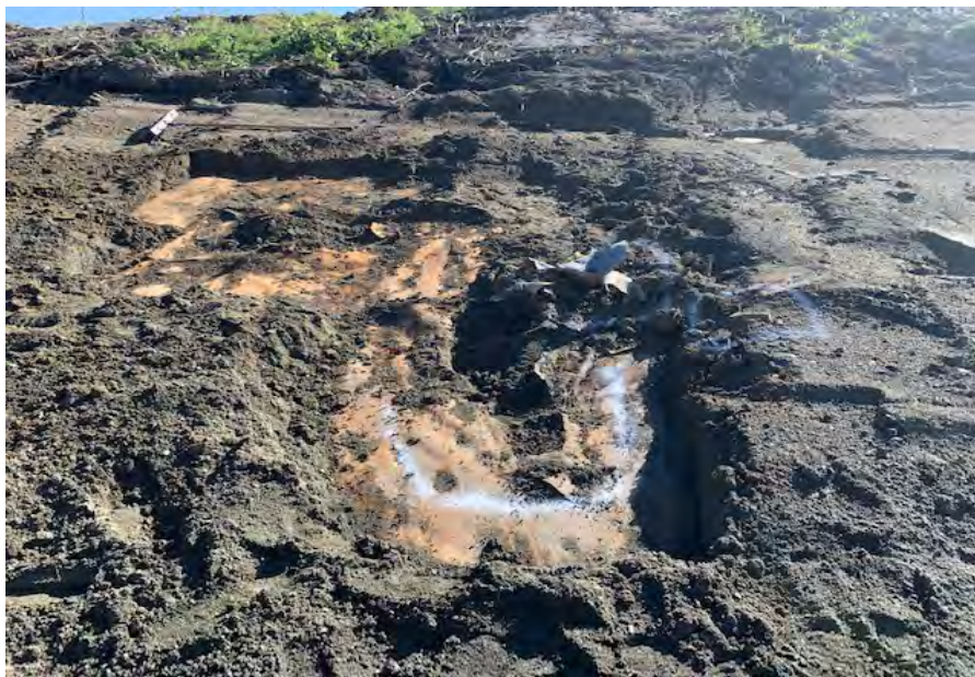
Photograph 18. Liner damage identified in lower pond. (October 6, 2020)
