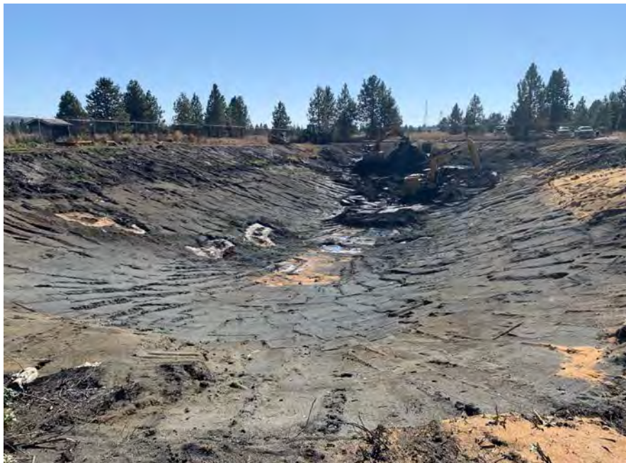
Photograph 20. Lower pond sediment removal. (October 7, 2020)
