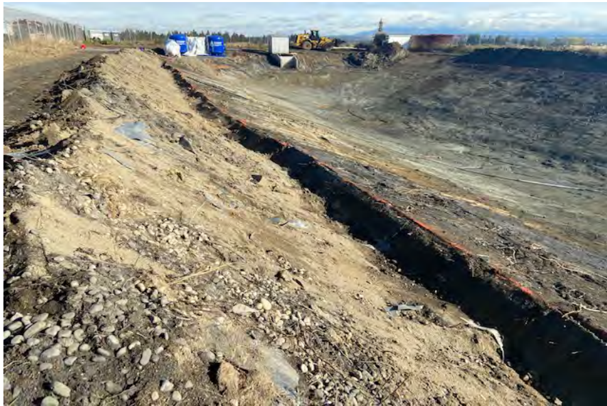
Photograph 23. Sediment removal completed from lower pond. (October 15, 2020)
