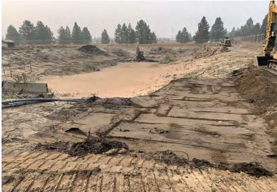
Photograph 11. Clean Harbors mixing wood pellets into lower pond sediment using a track hoe. Soil pad constructed for water treatment system. (September 17, 2020)
