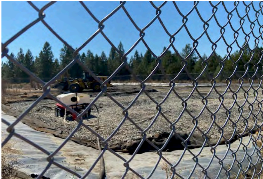
Photograph 4. Clean Harbors removing sediment from upper pond. Water buffalo used for dust suppression. (September 1, 2020)
