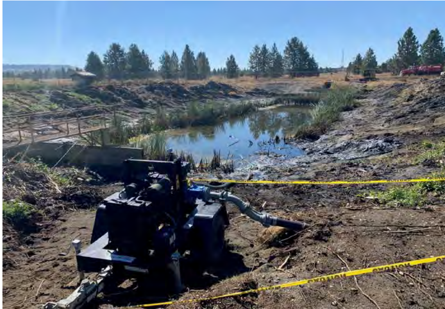
Photograph 7. 500 gallon per minute pump dewatering lower pond and discharging to upper pond. Pump inlet attached to floats and secured by ropes. (September 9, 2020)
