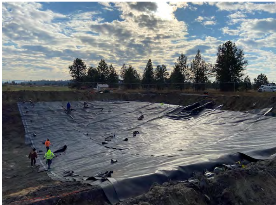
Photograph 26. Geosynthetic liner installation in lower pond. (October 22, 2020)
