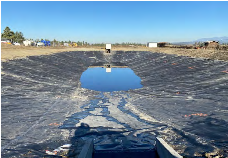
Photograph 27. Geosynthetic liner installation in lower pond. (October 22, 2020)
