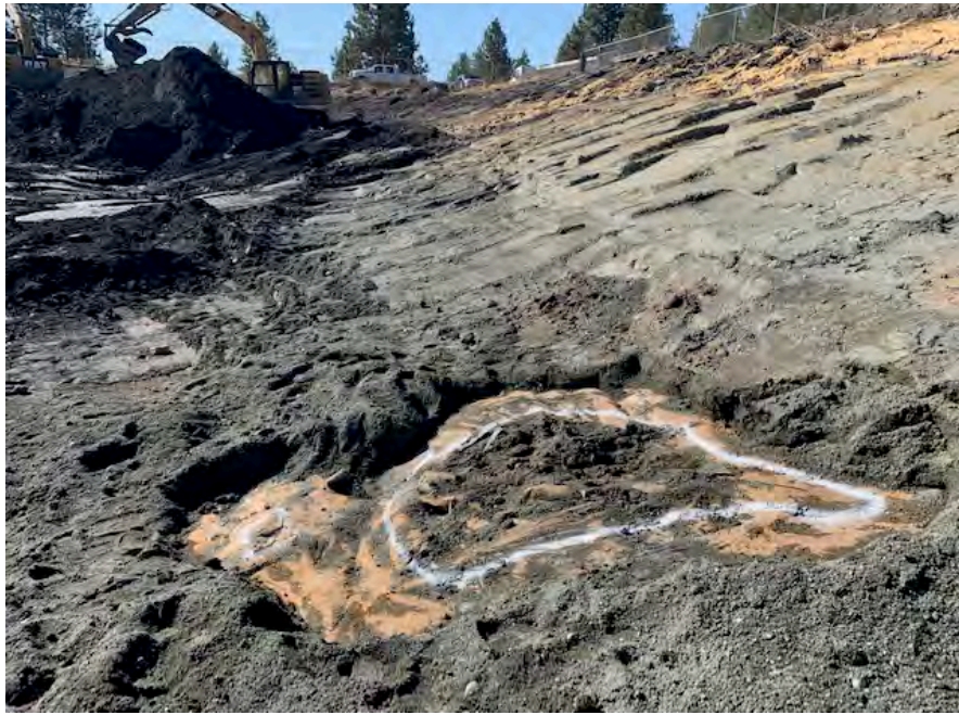
Photograph 19. Liner damage identified in lower pond. (October 6, 2020)
