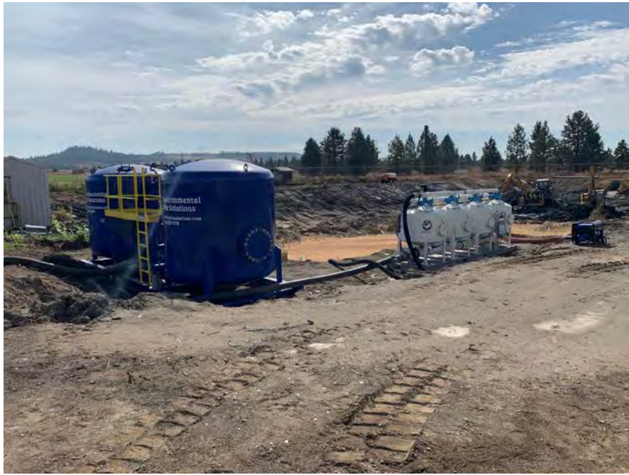
Photograph 13. Water treatment system (carbon vessels and sand filters) staged at north end of the lower pond. (September 30, 2020)
