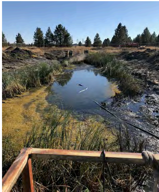
Photograph 7. 500 gallon per minute pump dewatering lower pond and discharging to upper pond. Pump inlet attached to floats and secured by ropes. (September 9, 2020)
