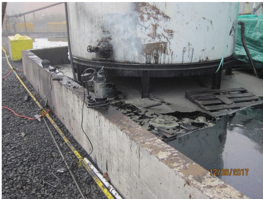
Figure 4: Wood vinegar and wood tar accumulated within secondary containment observed by Ecology during a 2017 inspection.
