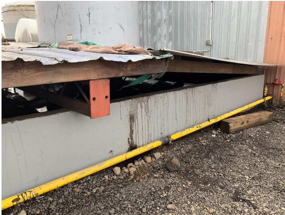
Figure 5: Staining along containment sidewalls observed by EPA in 2021 suggests the potential for releases of hazardous substances from overflow and cracks in the walls.
