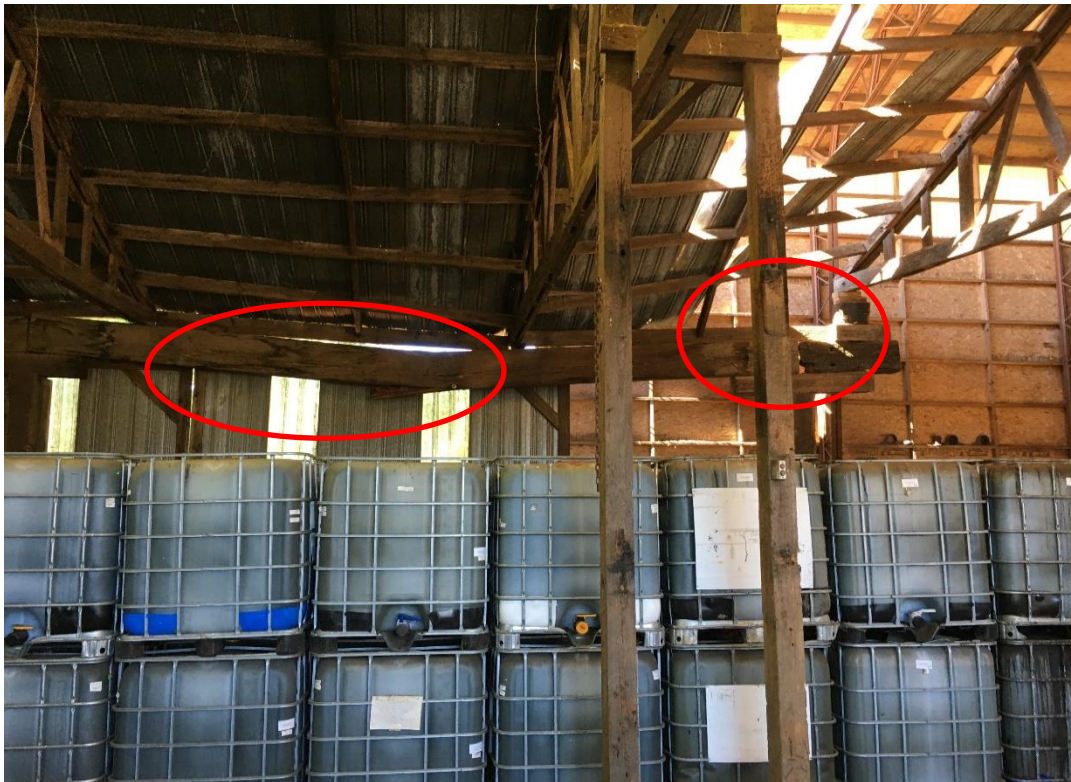
Figure 6: Totes containing 43,675 gallons of hazardous substances stored in the structurally unsound sawmill building days before it collapsed. Two key areas of concern to the Lewis County Building Official are circled in red.
