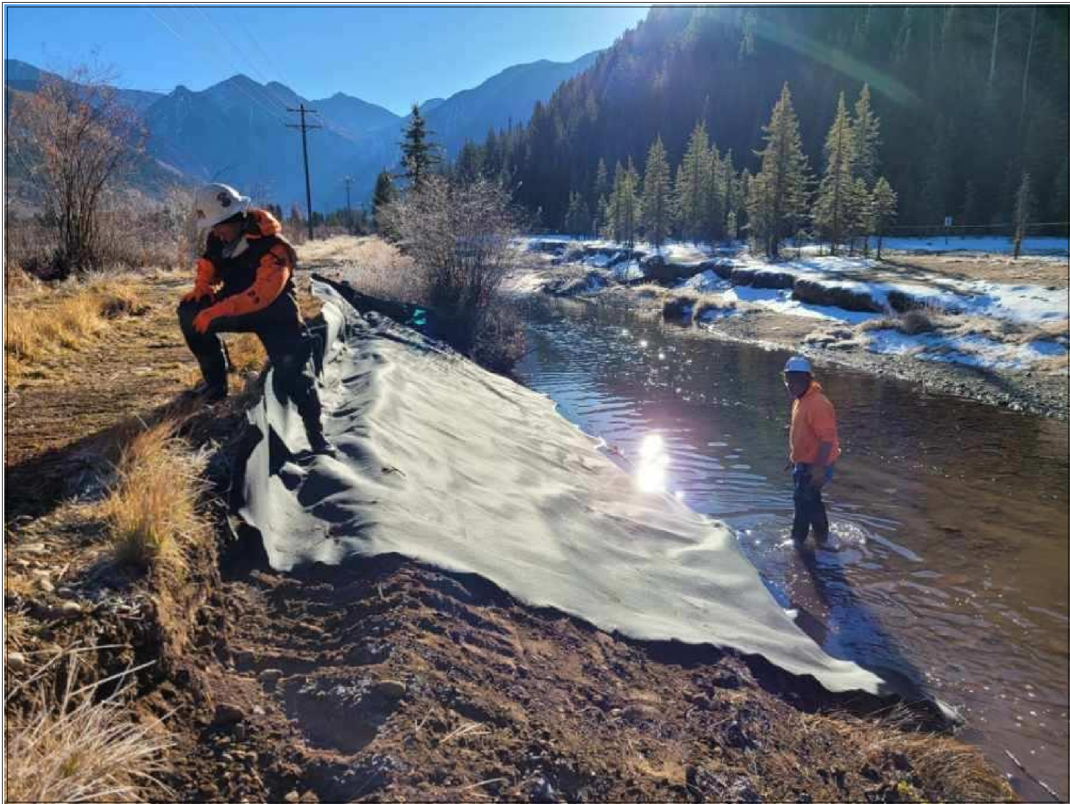
Liner installation on the north Riverbank.
