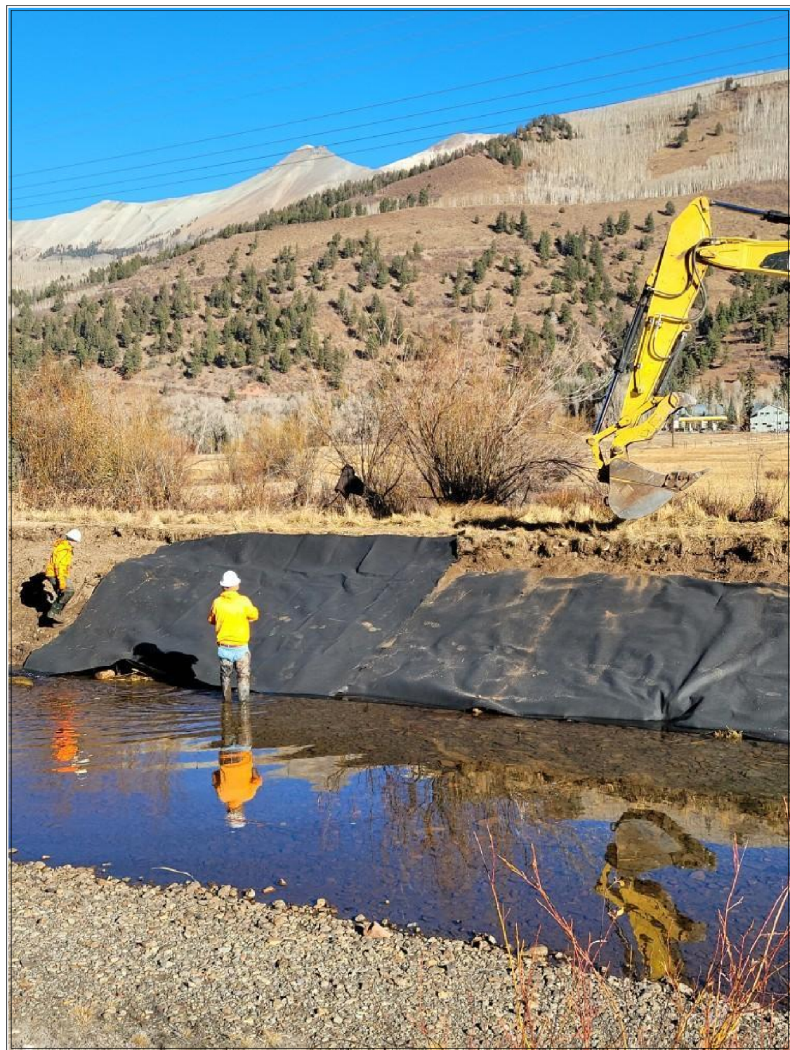
Installing a geo-textile liner to keep solids from passing through.
