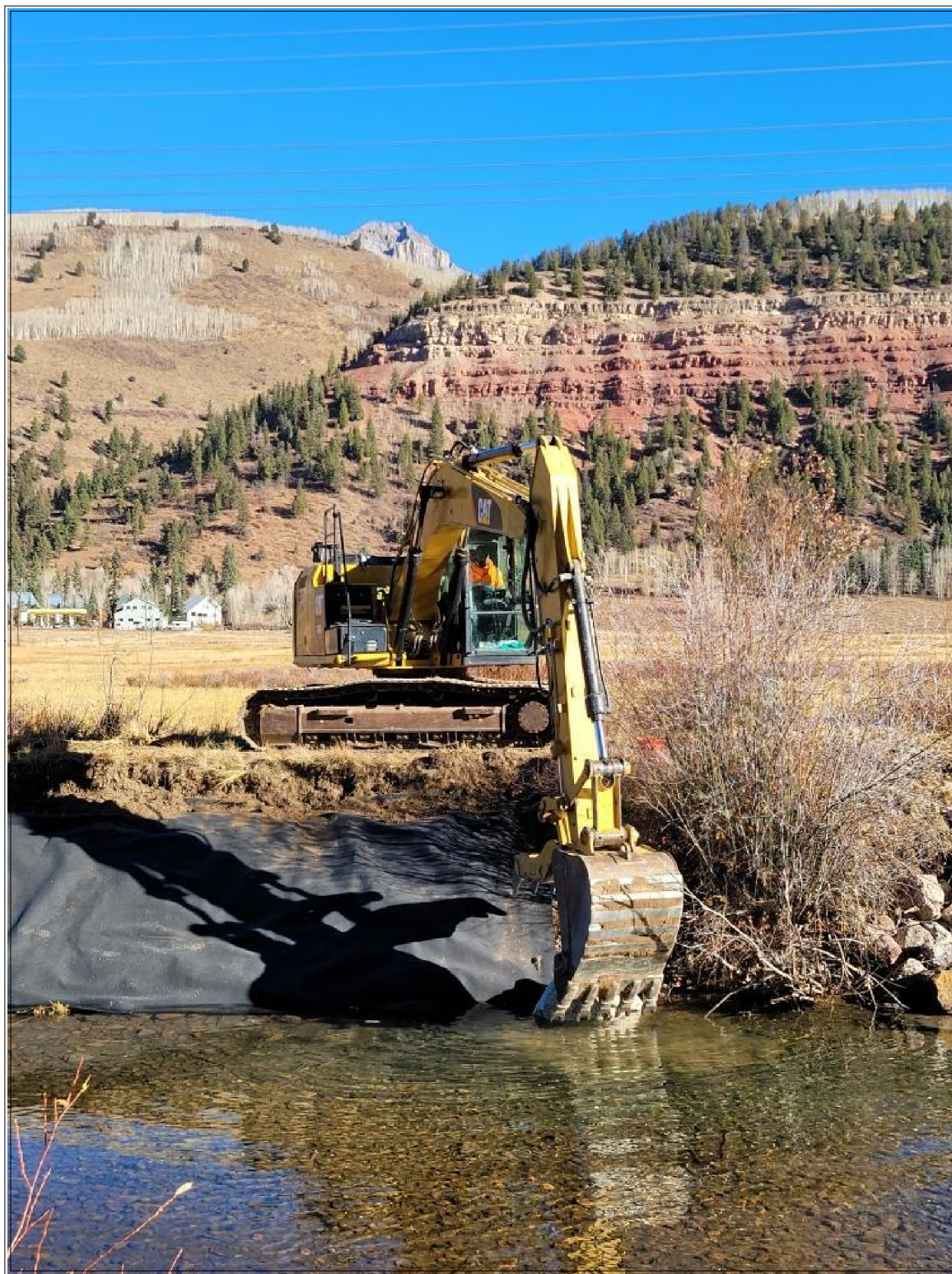
Securing the geo-textile liner with large rip rap.
