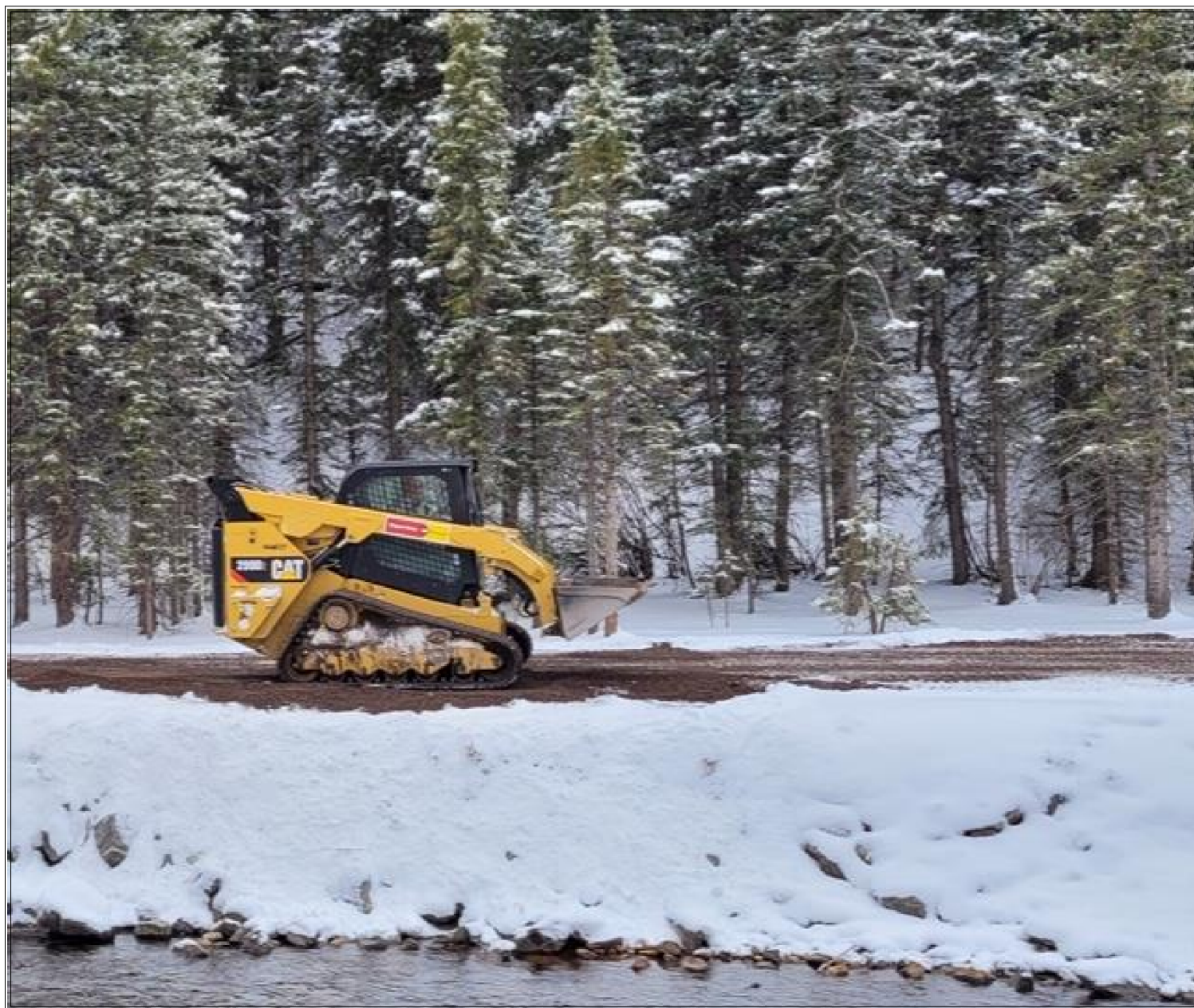
Road base install with front loader on south side of river.
