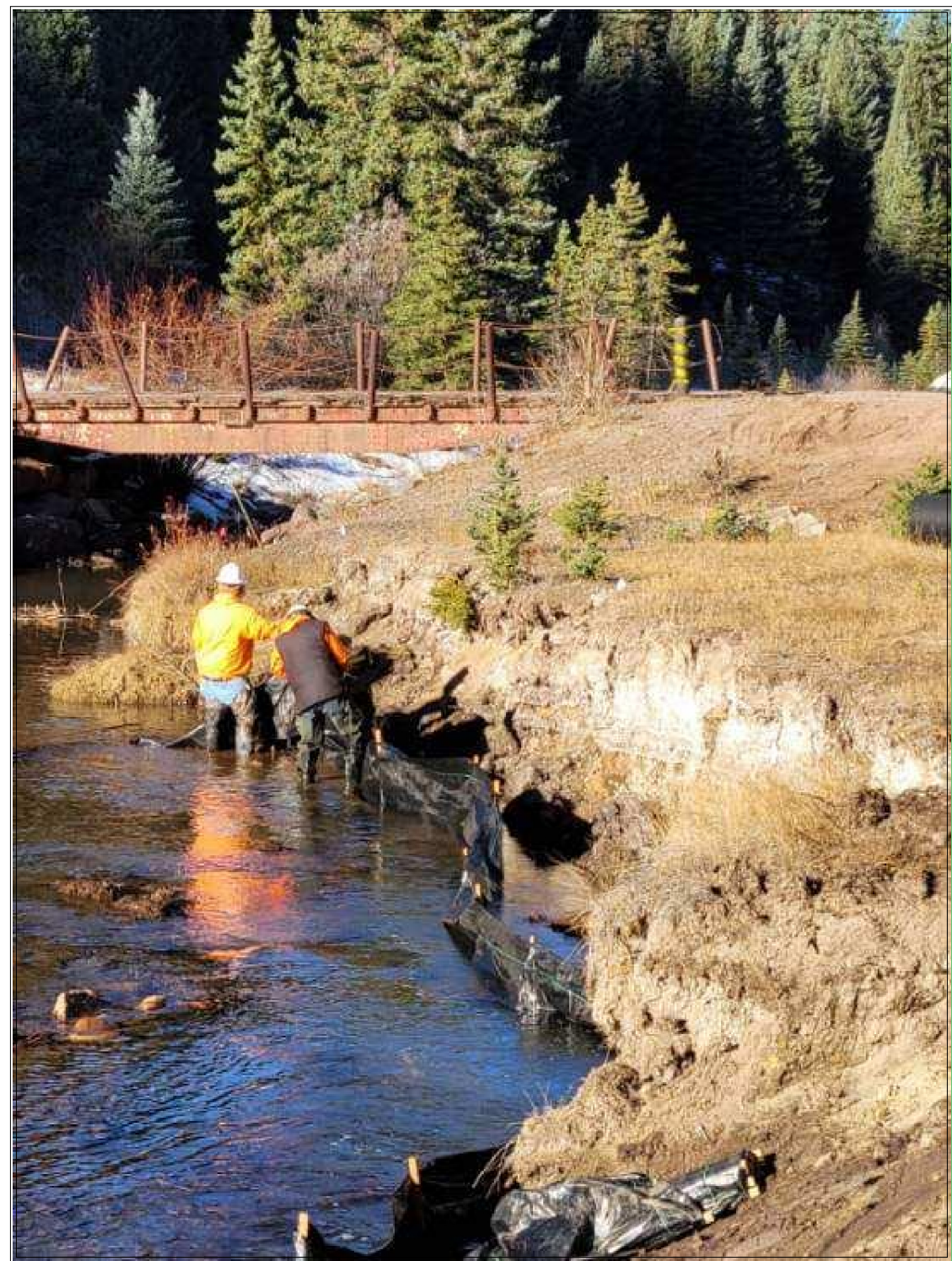
Installing erosion controls before the stream bank containing tailings is pulled back.
