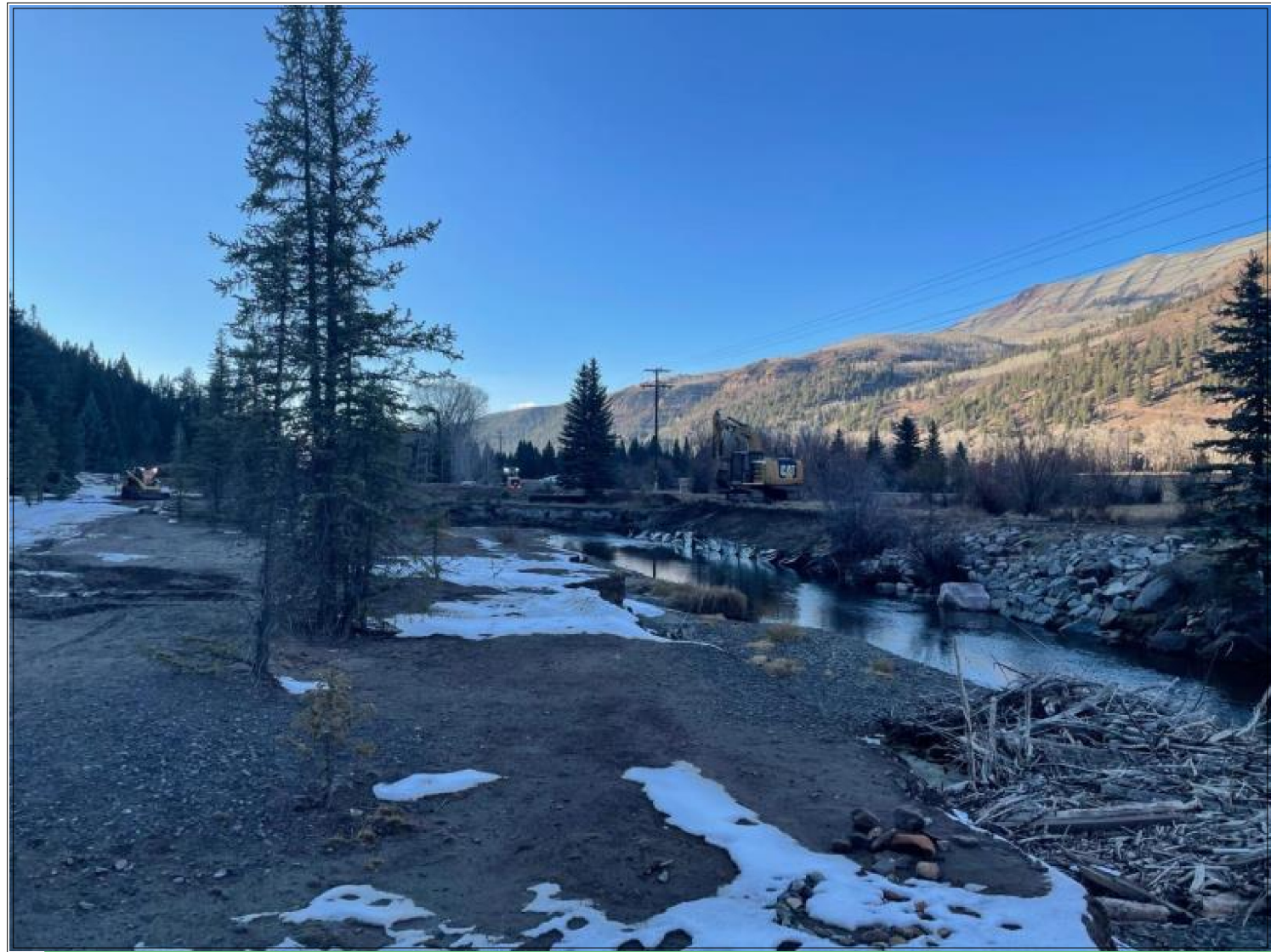
A portion of the rip rap completed on the north riverbank.
