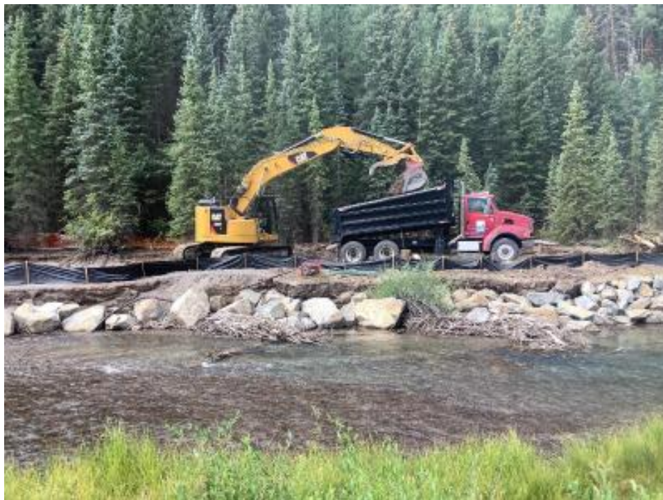
EPA contractor loading tailings within area ST1. The excavator loads tailings directly into dump trucks. Once loading is complete, trucks cover the load with a tarp and are cleaned prior to making the drive to the repository.
