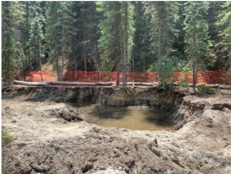
Ponding of water after excavation of tailings in the south-central portion of ST1. Tailings can still be seen as EPA contract crews continue removal actions.
