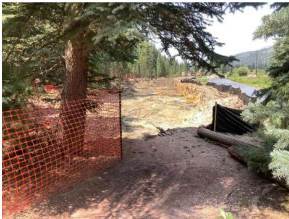
Excavated tailings up to the eastern-most fence line in ST1. Tailings can be visually identified by its characteristic coloring, grain size and deposition.
