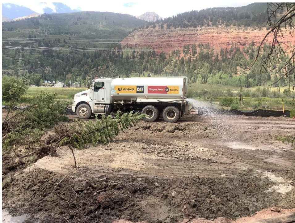
Water truck spraying water around ST1 to minimize dust particulates in the air.
