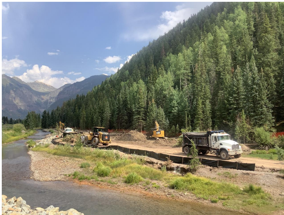
Dump truck with a load of tailings from ST1 heading to the Idarado repository. The loaded tailings are covered with a tarp and is watered down prior to the transport of tailings.
