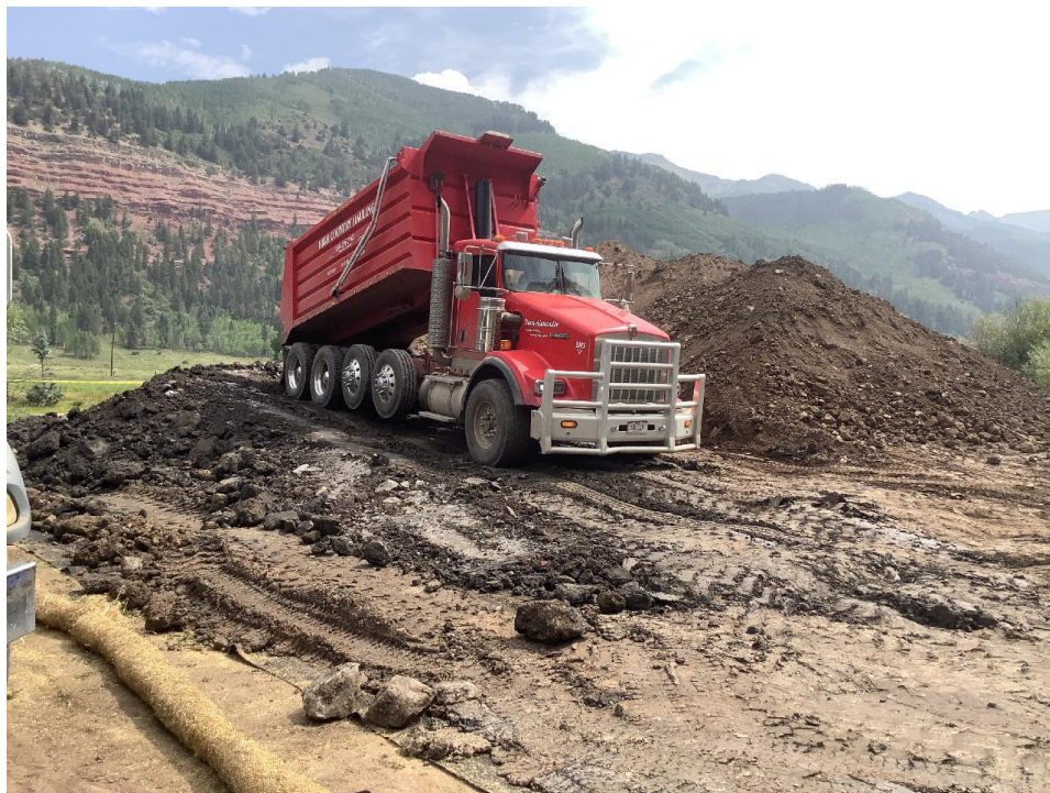
Dump trucks from local landslides delivering clean fill material/soil to site. Fill materials will be used for restoration and back filling excavation areas.
