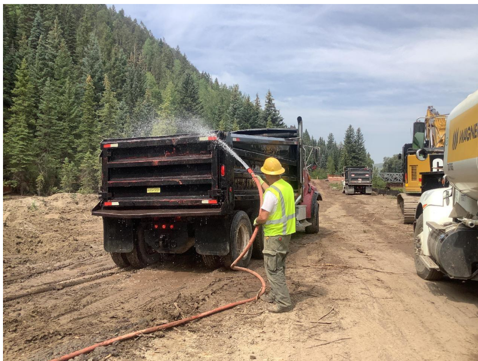
Dump truck operator washing down loaded truck and ensuring that the excavated tailings are watered down prior to departing.
