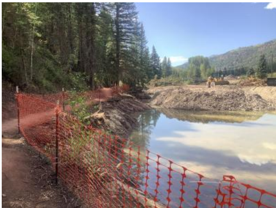
Backfill operations have begun in the western portion of ST1 Central, the excavated tailings are being replaced with clean soil.
