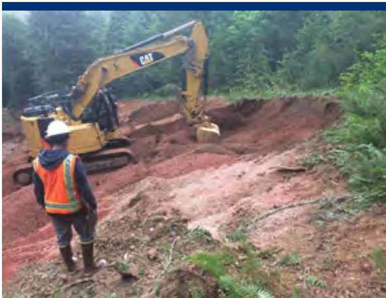
Photo 10 Tailings removal along right bank near station 3+50.
