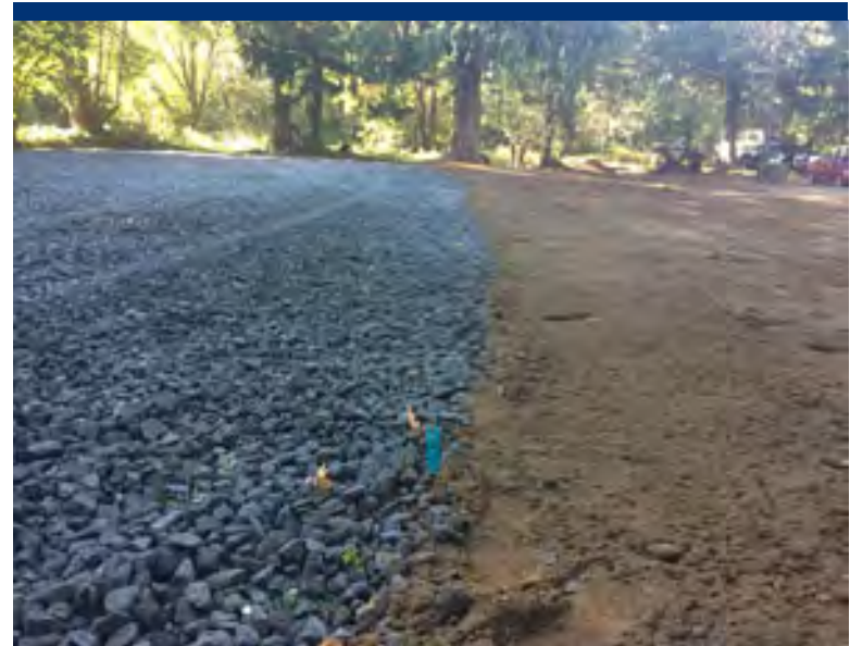
Photo 31 Gravel and clean soil backfill placed, compacted, and graded at DU10 and DU11.
