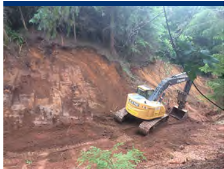
Photo 7 Excavation and scraping of left bank to clean between STA 4+25 and 5+00.
