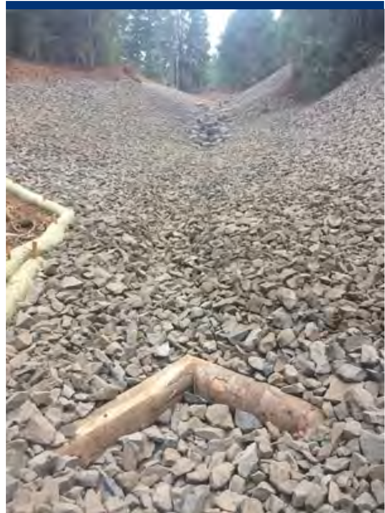
Photo 10 Completed wooden cross vane near Station 5+50.
