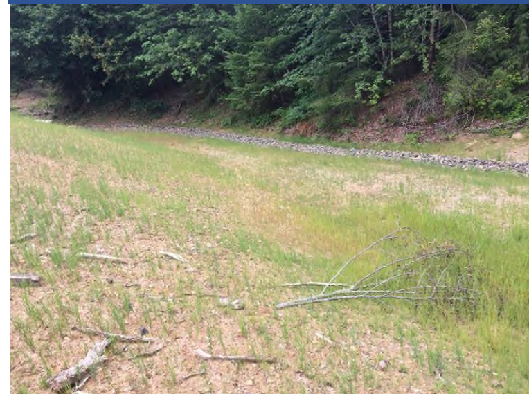
Photo 86 Section of Adit Creek reroute with negative drainage causing overflow, located on east side of repository.
