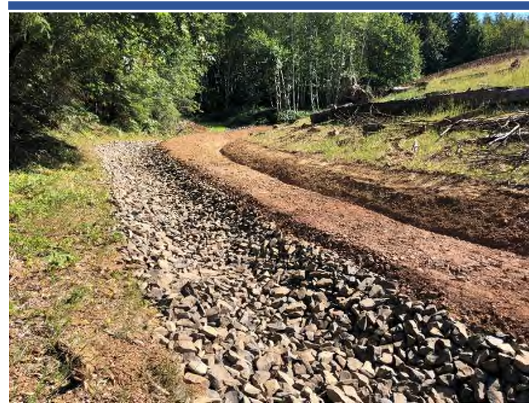
Photo 90 Completed Adit Creek reroute enhancement to improve flow and drainage around repository.
