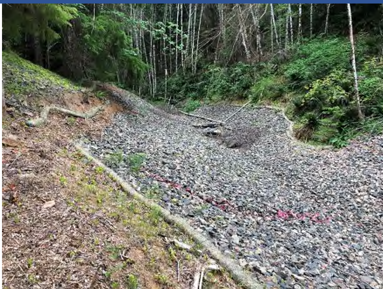
Photo 65 Looking upstream at Furnace Creek Old Furnace right bank slope failure. Downstream extent of slide marked in pink.
