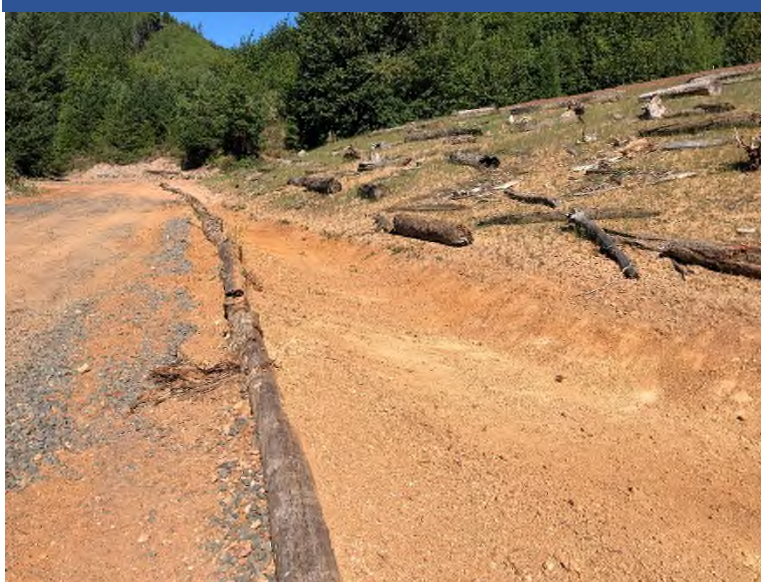
Photo 91 Repository drainage channel excavated by ERRS to be wider and deeper to improve flow and capacity.
