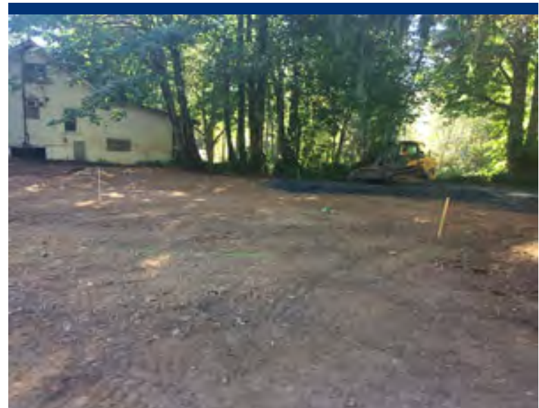
Photo 21 ERRS placing gravel into DU03, with backfill stakes marked at 1-foot.
