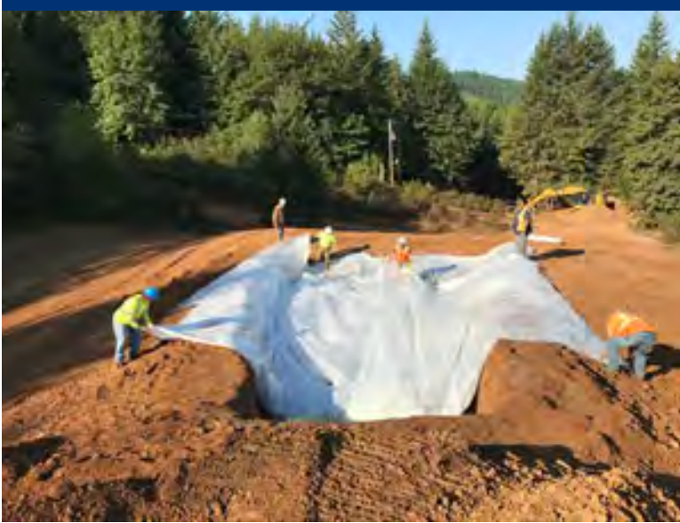
Photo 28 Burial of soil containing high concentrations of mercury and micro beads within the repository.
