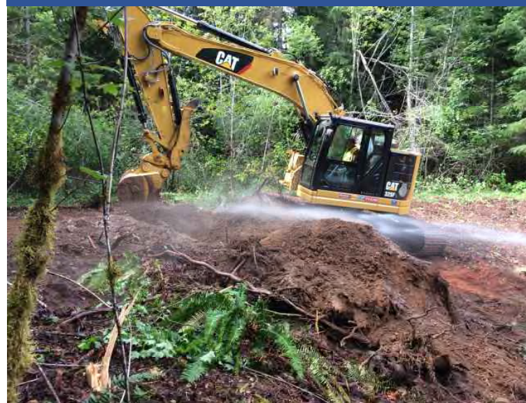
Photo 10 ERRS conducting dust control while excavating OPWA Upper/South unit.
