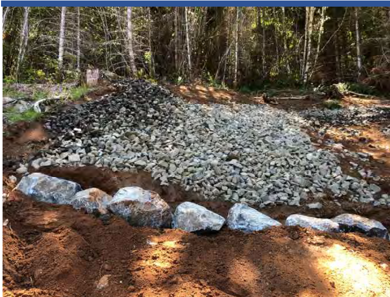
Photo 59 Repaired right bank slope failure area with keyed-in boulders along toe of slope, and rock armor.
