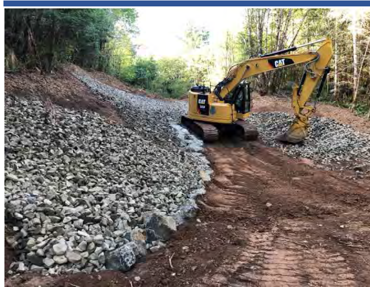
Photo 32 ERRS placing boulders in keyed-in trench along toe of right bank slope of OPWA Upper/South unit.
