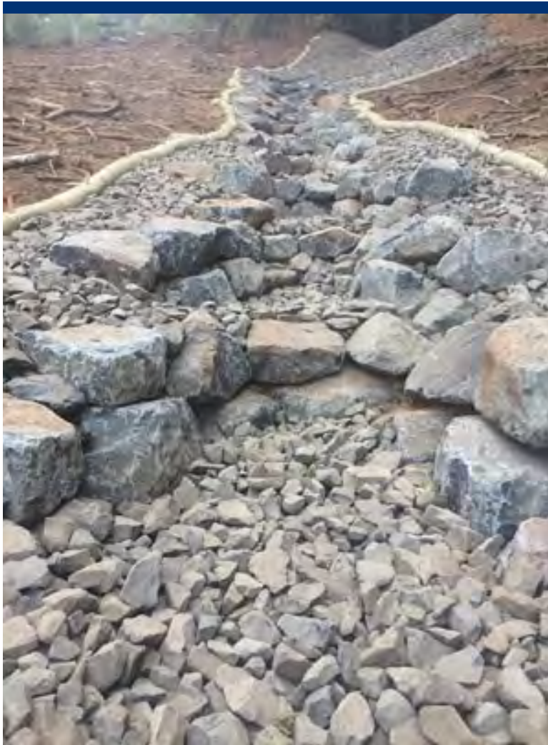
Photo 9 View of completed cross-vanes between Stations 2+50 and 3+00.
