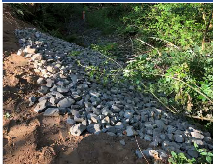
Photo 38 Rock-armored overflow spillway at northwest extent of OPWA Lower/North unit.
