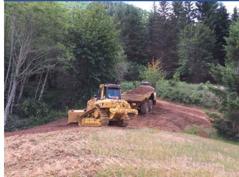
Photo 42 ERRS placing excavated contaminated material hauled from OPWA removal area into repository.
