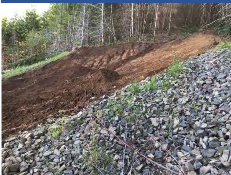
Photo 57 Left bank slope of Adit Creek seep pulled down to 2:1 slope.
