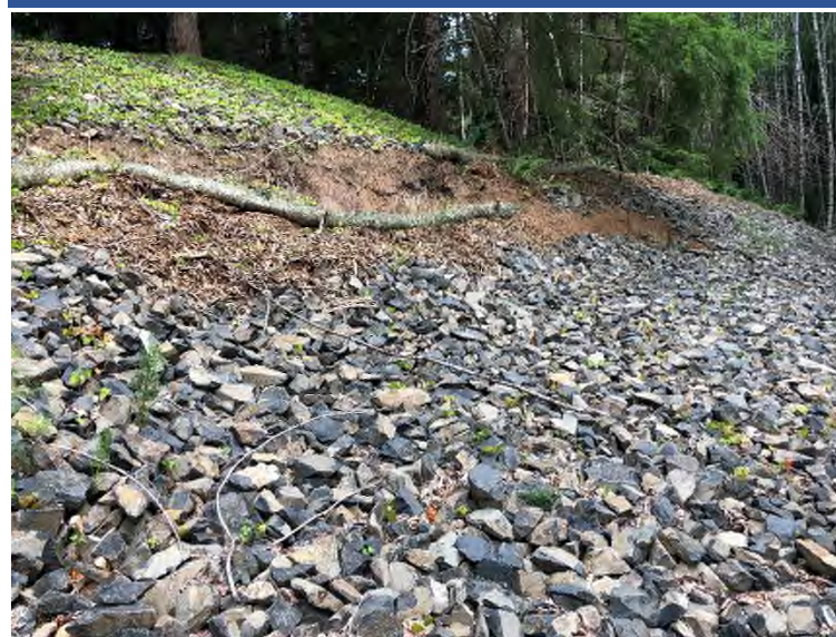
Photo 66 Slope failure and exposed contaminated bank located near right bank of Furnace Creek at STA 1+00.
