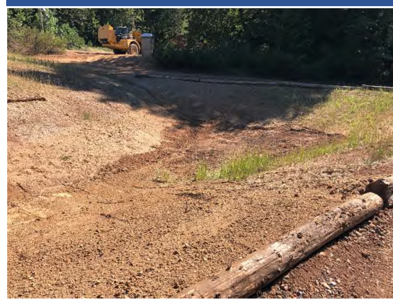
Photo 92 Repository stormwater retention pond with 4'-6" of sediment excavated by ERRS.
