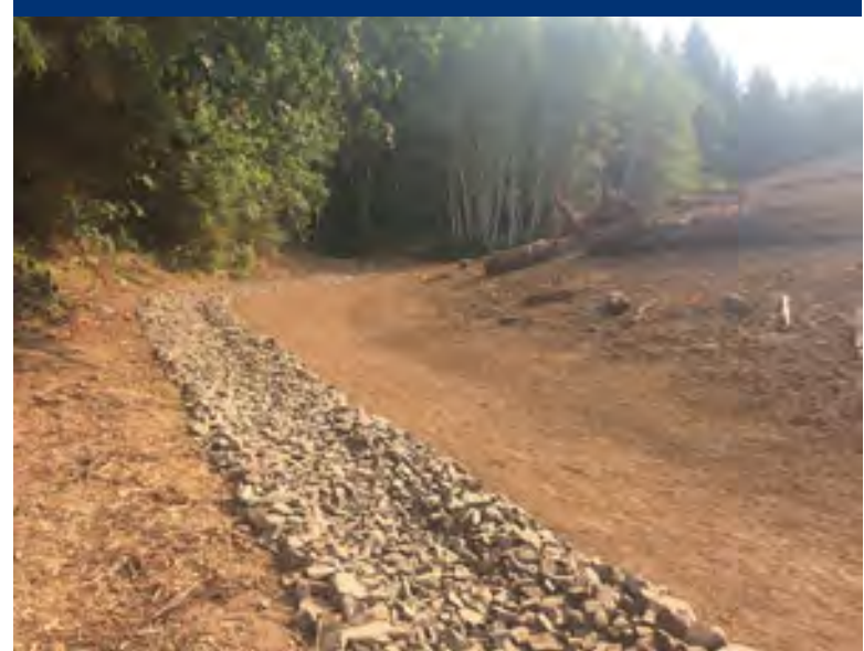
Photo 16 View of completed Adit Creek re-route around repository.
