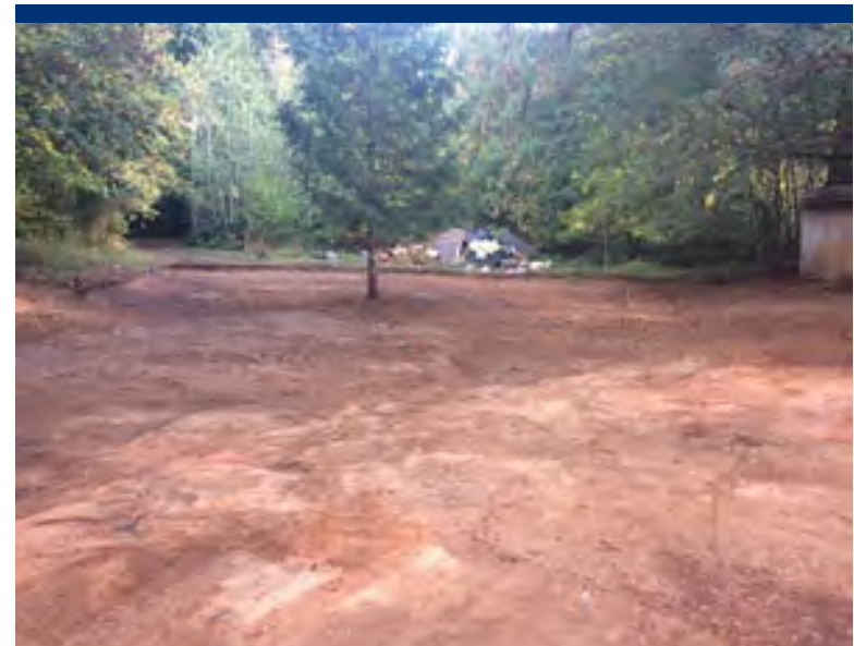
Photo 9 DU06 and DU08 excavated to 1-foot depth.
