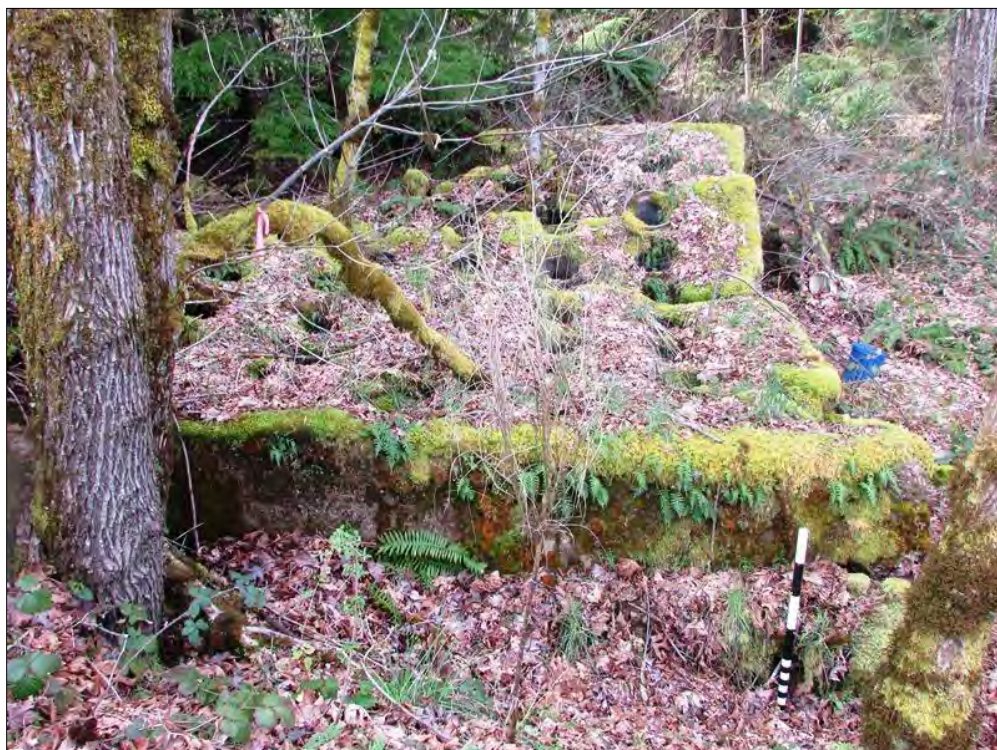
Figure 11. View looking south of the top of the uppermost slab showing the round holes where tile condenser pipes would have entered the mercury collection building.
