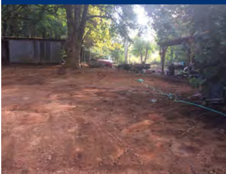
Photo 10 DU06 excavated to 1-foot depth, and DU09 scraped around base of trees.
