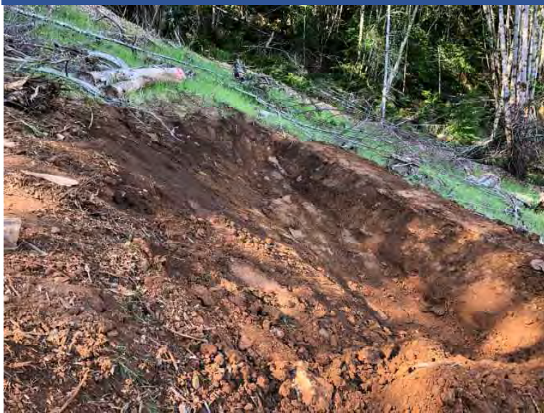
Photo 61 Left bank Adit Creek seep intercept channel installed by ERRS to direct flow into main Adit Creek channel.
