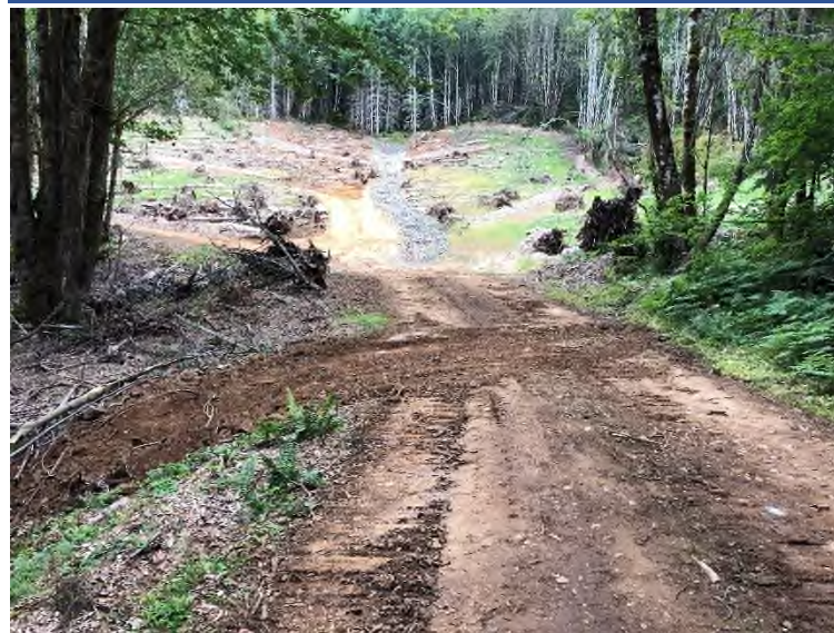
Photo 94 Water bar (shown prior to receiving gravel armor) across borrow source access road, and downgradient of BS01.
