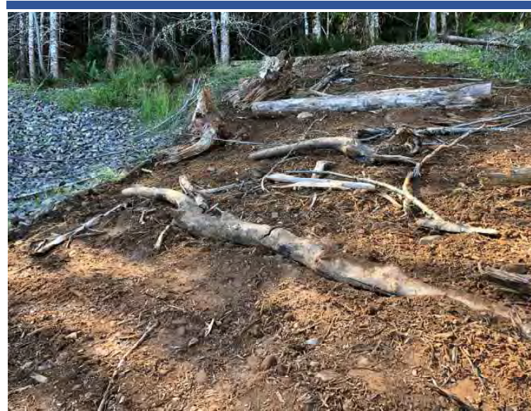
Photo 60 Repaired left bank slope failure area of Adit Creek seep, with slash and soil/mulch cover over rock armor layer.
