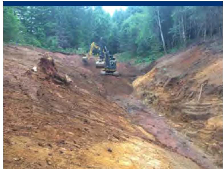
Photo 11 Looking upgradient across completed channel excavation, to excavation activities at STA 3+00.
