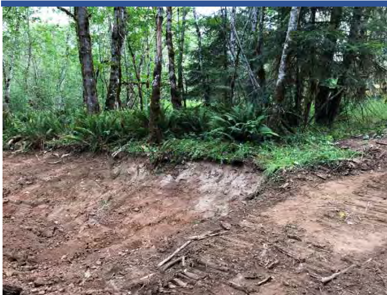
Photo 27 Final excavated leave surface of N extent OPWA Lower/N unit. Note: ashy material left in-place (<300 mg/kg Hg).
