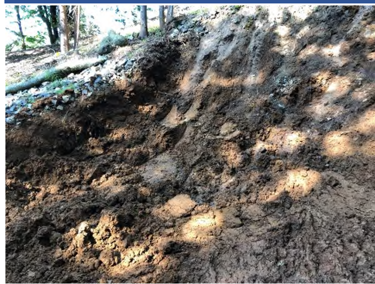
Photo 70 Saturated soils due to subsurface seep at downstream extent of excavated Old Furnace slope failure.
