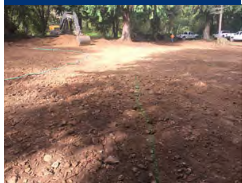
Photo 11 Painted line delineating placement of soil (to right/N) and gravel (to left/S) in DU10 and DU11.
