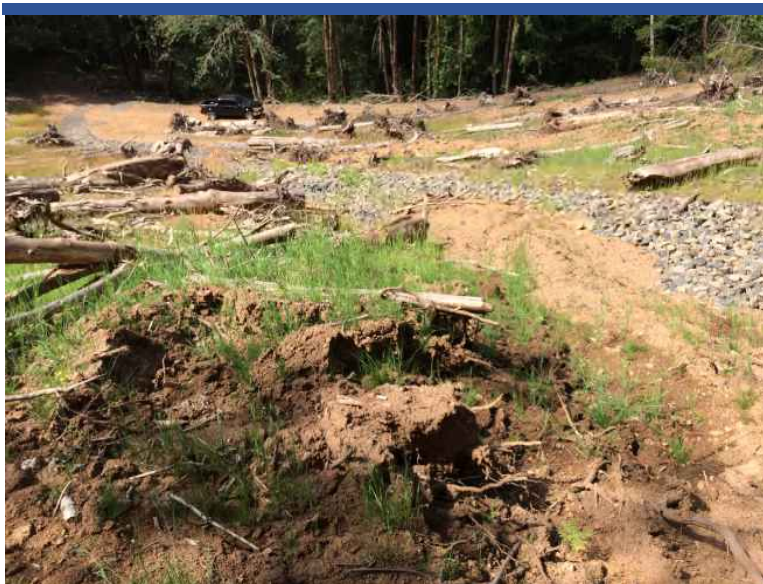
Photo 55 Looking downslope at left bank slope failure of Adit Creek seep at BS01.
