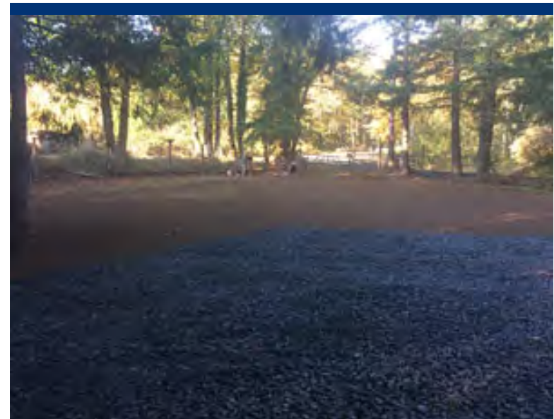
Photo 37 Gravel and clean soil backfill placed, compacted, and graded at DU04 and DU05.
