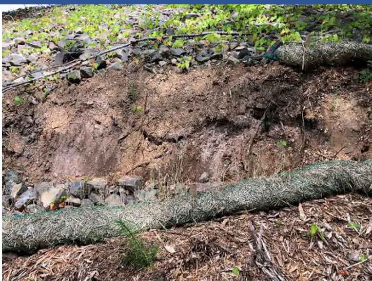
Photo 67 Slope failure and exposed contaminated bank located near right bank of Furnace Creek at STA 1+00.
