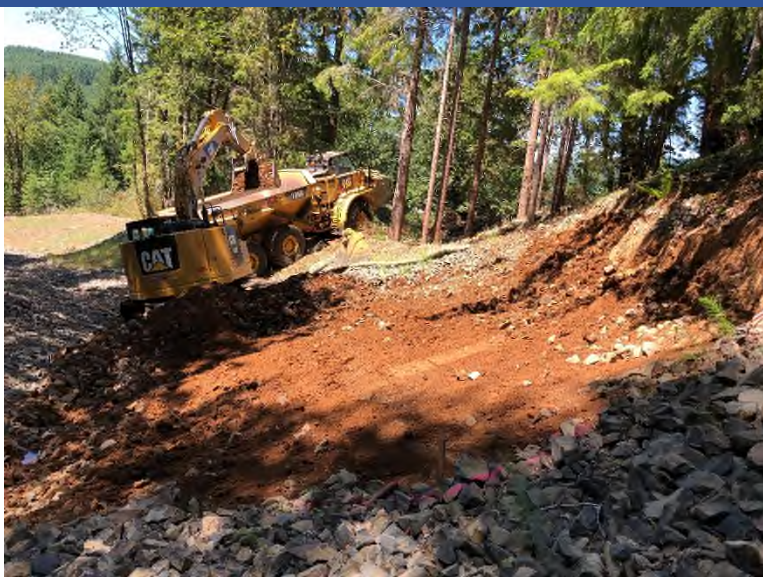
Photo 69 ERRS loading clean backfill excavated from Old Furnace slope failure.
