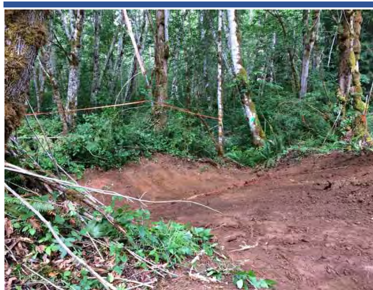
Photo 22 Excavated swale area in southwestern extent of OPWA Lower/North unit.
