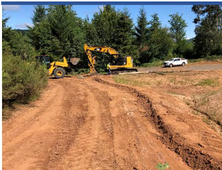
Photo 93 Drainage channel to direct surface flow from main access road away from repository stormwater retention pond.
