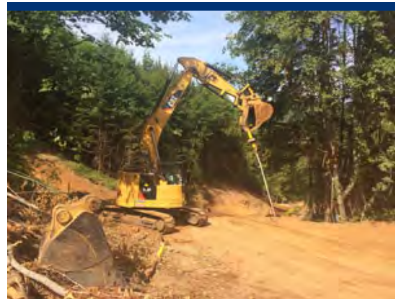
Photo 21 Abandonment of monitoring well MW-10, adjacent to the STA 2+00.
