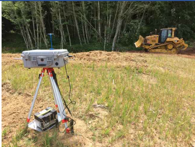
Photo 41 Air monitoring station AS-RP Dusttrak, located on top of repository. ERRS grading and prepping repository.
