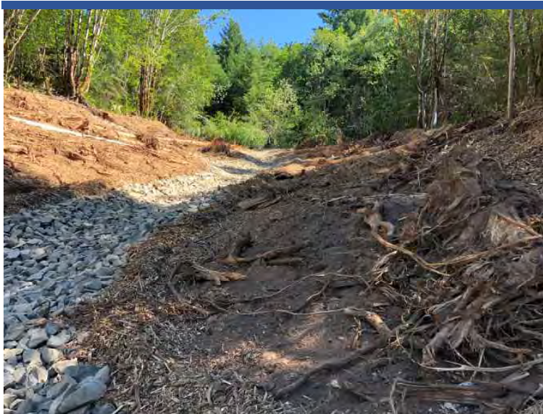
Photo 31 Restored section of OPWA Upper/South unit, with rock-armored constructed drainage channel, mulch and slash.
