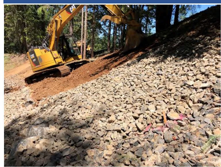
Photo 84 ERRS compacting restored slope in Furnace Creek Old Furnace slide repair area.
