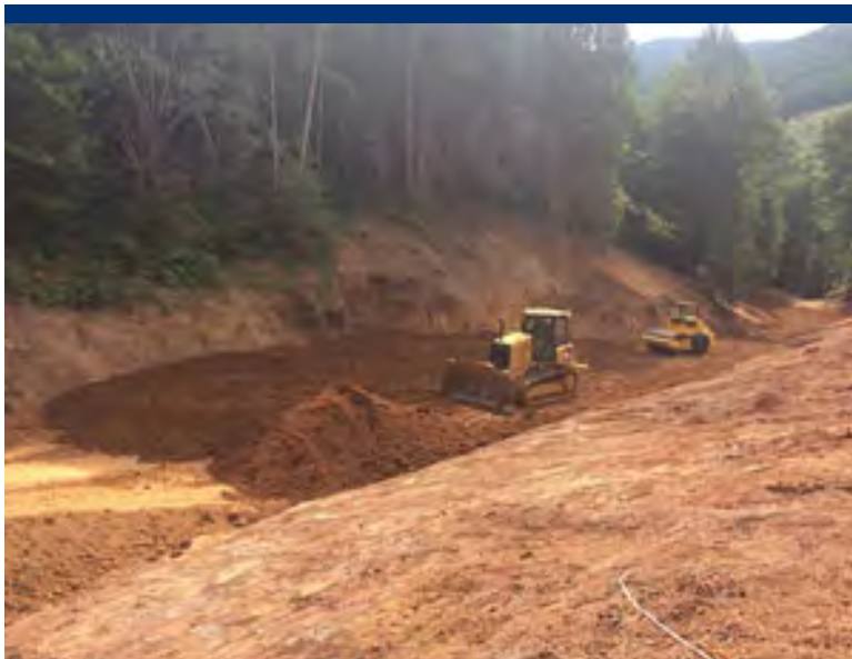
Photo 3 Backfilling Furnace Creek with clean fill material.
