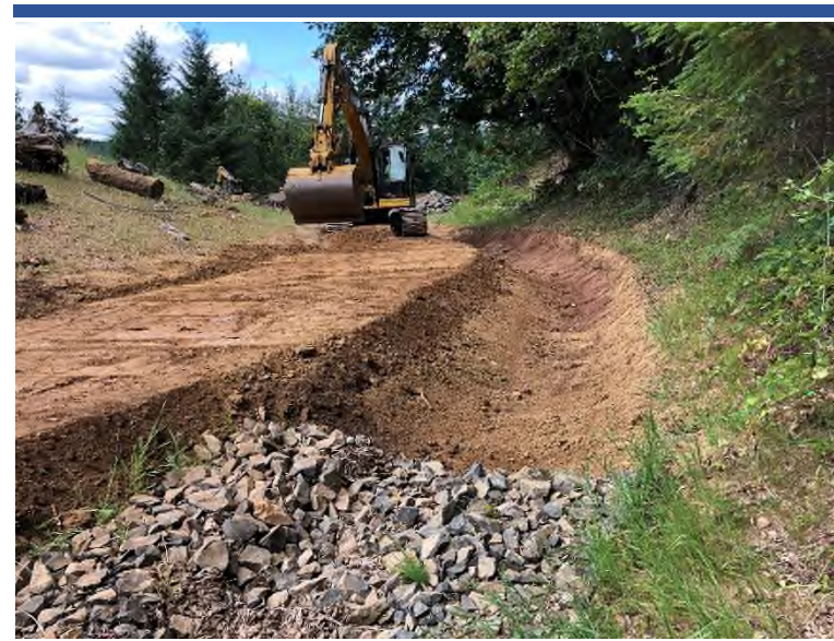
Photo 88 Widened and deepened Adit Creek reroute enhancement to improve flow and drainage around repository.
