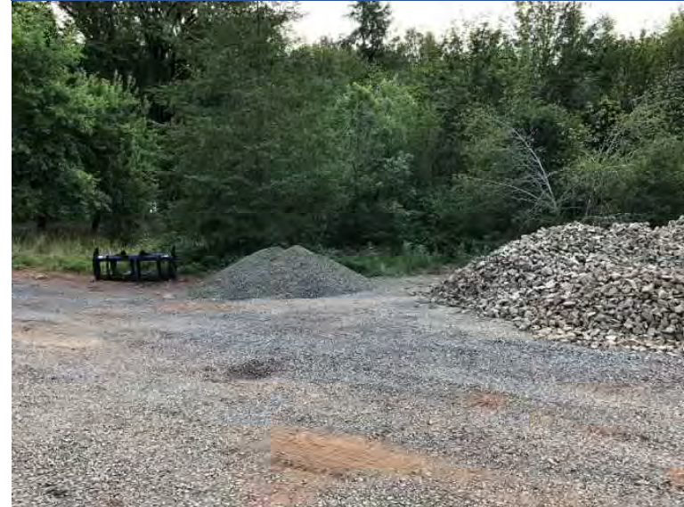
Photo 2 Stockpiled 1.5-inch-minus rock and 6-inch rock armor, staged in support zone area.
