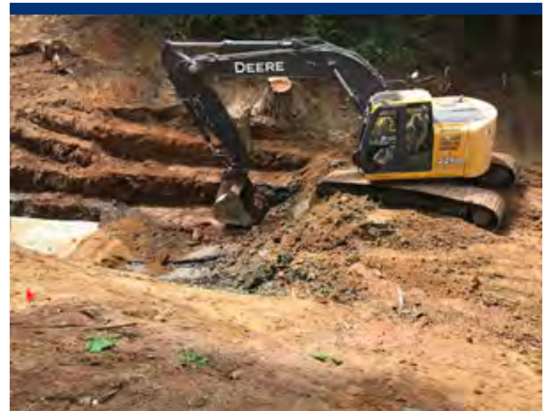
Photo 4 Removal activities utilizing benching near Station 1+50.
