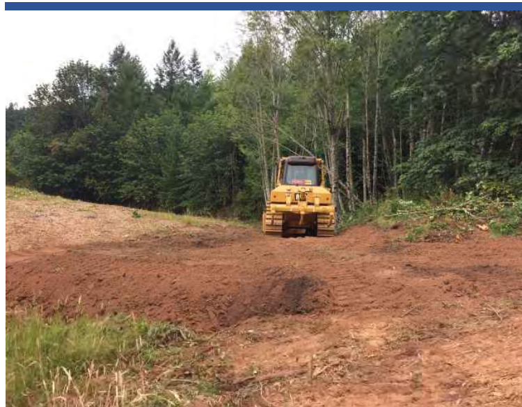
Photo 40 ERRS grading and prepping repository to receive material excavated from OPWA removal area.
