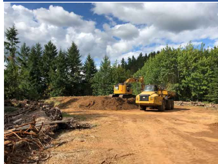
Photo 44 ERRS loading stockpiled residential removal material into haul truck, located in north laydown area.
