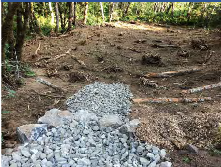
Photo 37 Restored section of OPWA Lower/North unit, with rock-armored constructed drainage channel and riprap.
