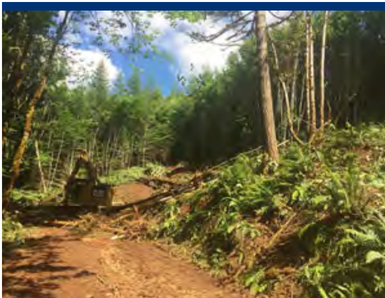
Photo 26 Clearing and grubbing activities at Borrow Source 1.
