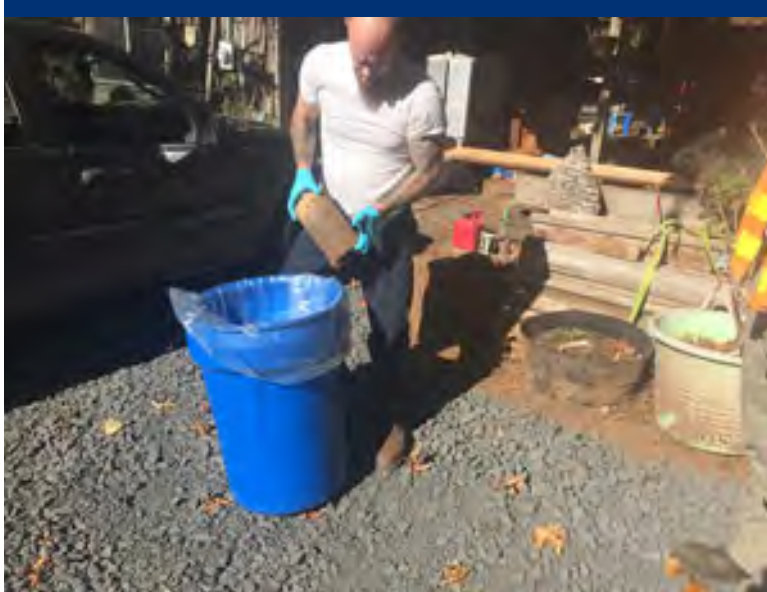
Photo 34 Subcontractor staging mercury flasks for off-site transportation and disposal.
