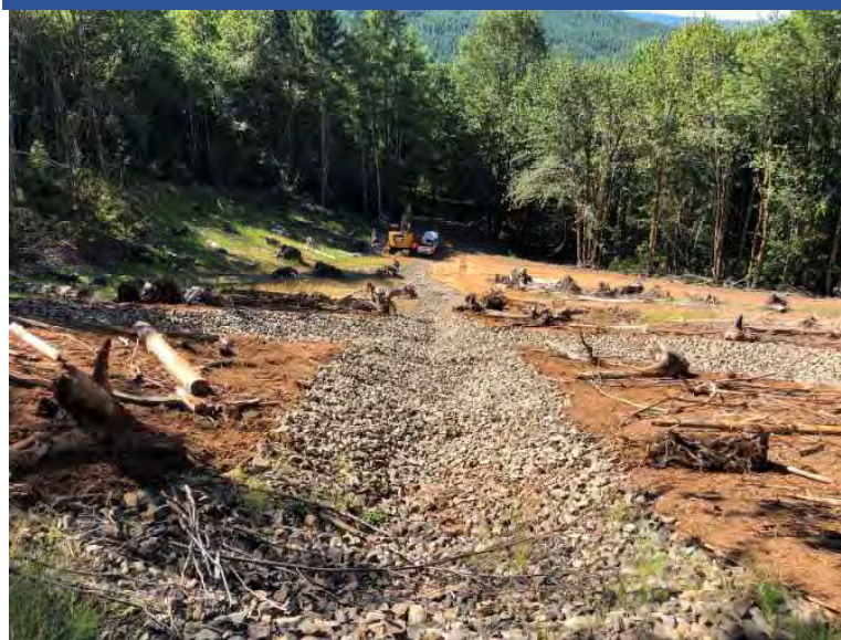
Photo 63 Looking downslope along main channel of Adit Creek seep, and completed left bank and right bank channels.
