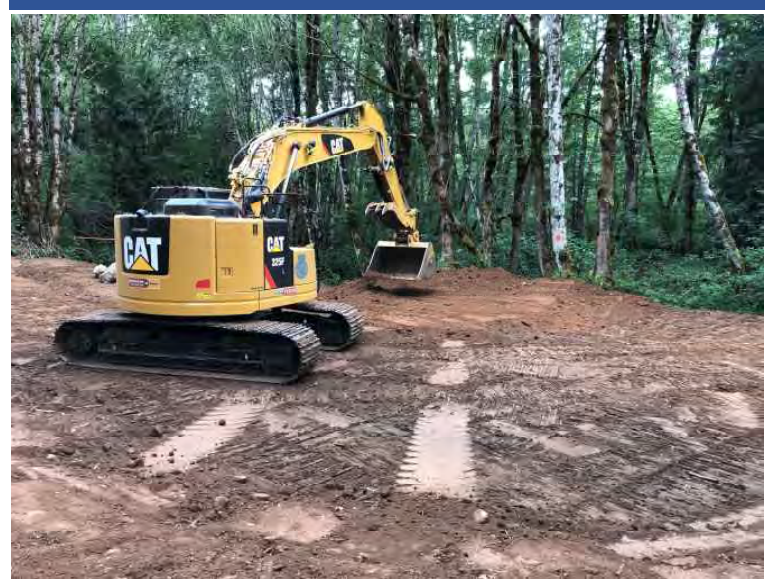
Photo 36 ERRS placing 1-foot clean cover cap in OPWA Lower/South unit.
