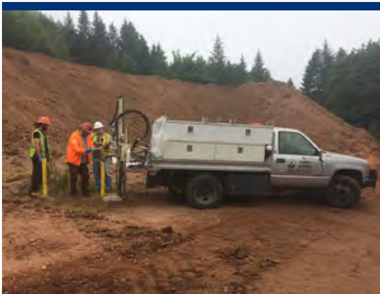
Photo 20 Abandonment of monitoring well MW-11, adjacent to the repository.
