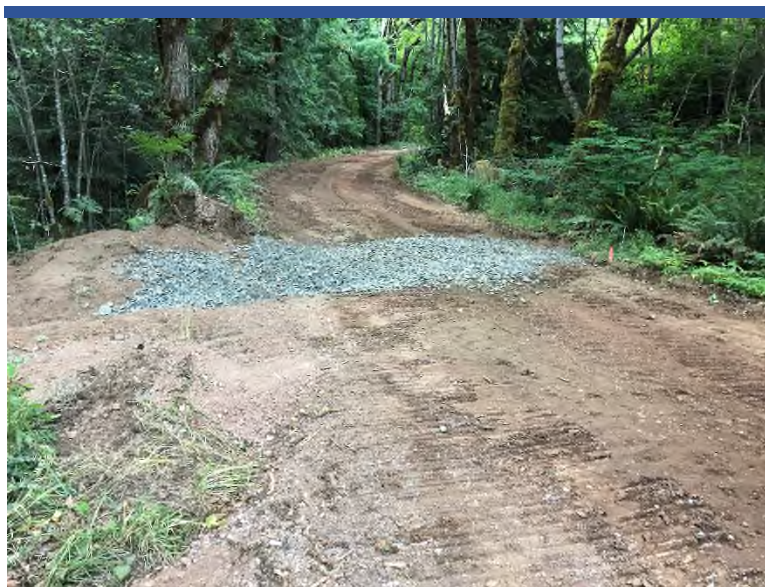
Photo 95 Completed water bar placed across main access road, near entrance gate and residence upper drive.
