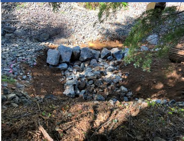
Photo 81 Completed boulder toe anchor at base of Furnace Creek Old Furnace slide repair, and installed rock layer backfill.
