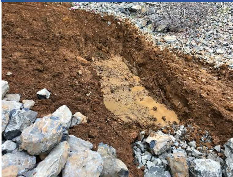
Photo 77 Groundwater infilling upgradient end of key anchor trench at toe of Furnace Creek Old Furnace slide repair area.
