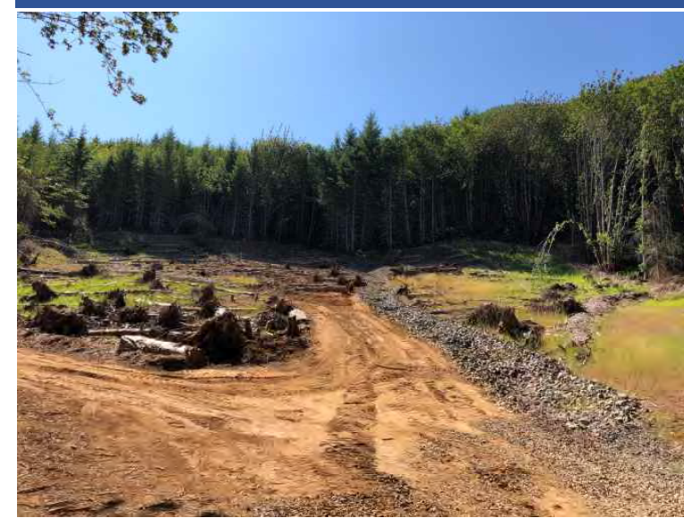
Photo 64 Looking up at BS01 borrow source repairs to address erosion and Adit Creek seep slope failure at top of slope.
