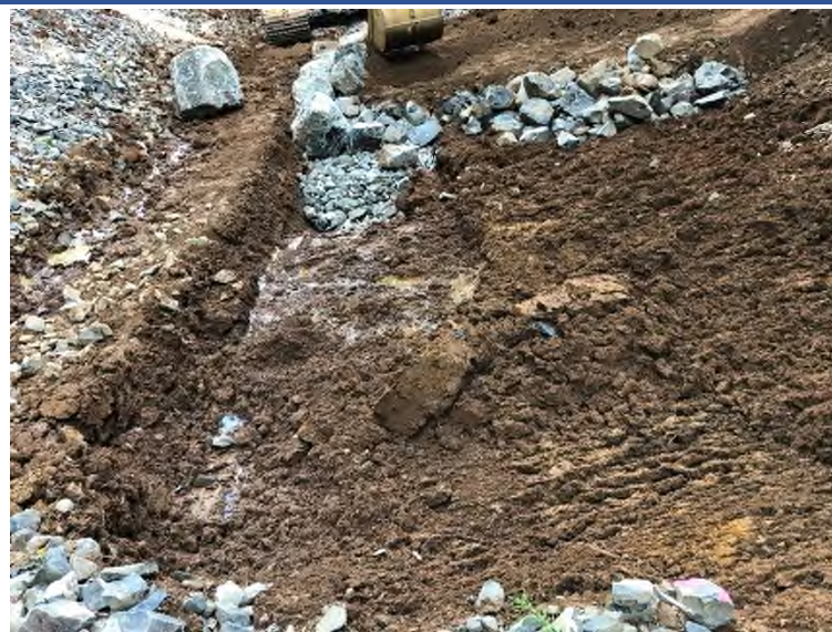
Photo 76 Groundwater infilling upgradient end of key anchor trench at toe of Furnace Creek Old Furnace slide repair area.
