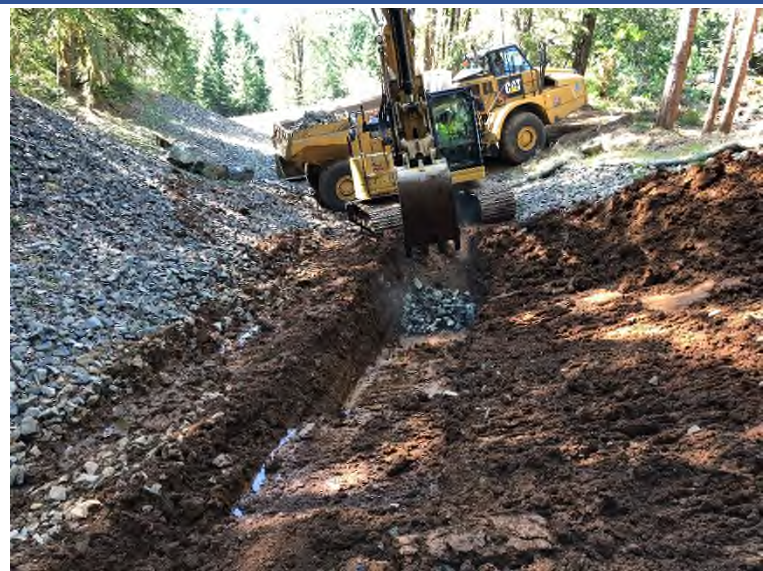
Photo 71 ERRS backfilling key trench with 6-inch rock for Furnace Creek Old Furnace slope failure repair.
