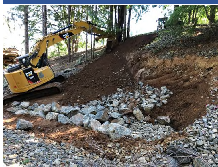
Photo 80 ERRS placing clean topsoil backfill over rock backfill layer in Furnace Creek Old Furnace slide repair area.
