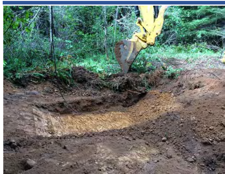
Photo 12 Excavated 'clean' clay layer, located at upper/southernmost boundary extent of OPWA Upper/S unit.
