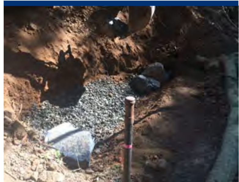
Photo 6 Placement of key ledge on RCV gravel bedding, at terminus of lower series of RCVs at STA 8+89.
