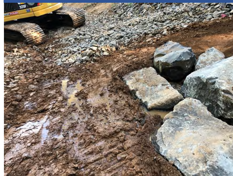
Photo 82 Groundwater flowing out from anchor trench installed for Furnace Creek Old Furnace slide repair action.
