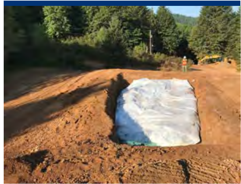
Photo 29 Burial of soil containing high concentrations of mercury and micro beads within the repository.
