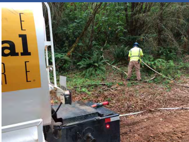
Photo 5 ERRS saturating OPWA Upper/South unit with the water truck for dust control prior to clearing/grubbing activities.
