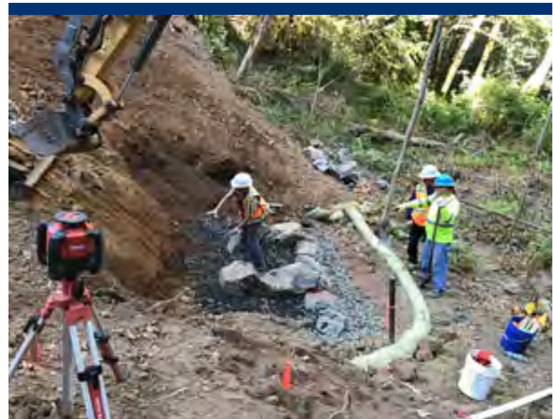
Photo 8 Initial Rock cross-vane construction near Station 8+50.
