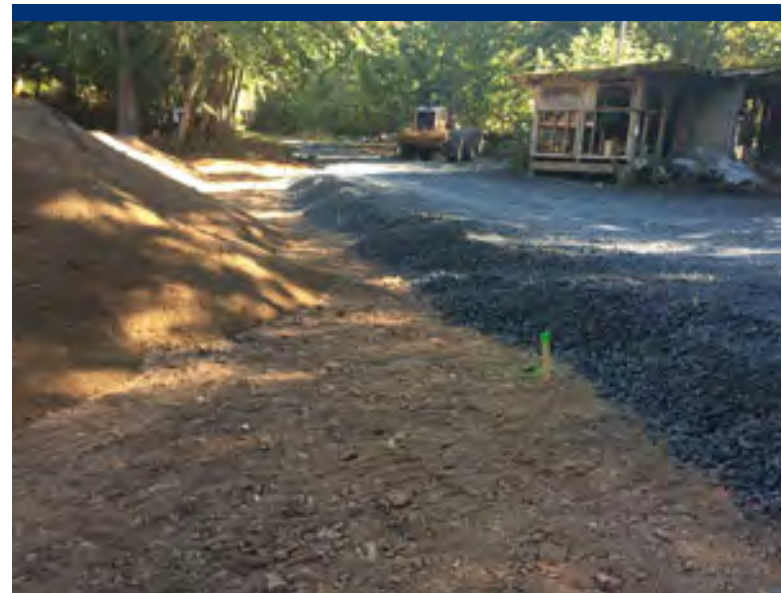
Photo 25 Staked out for one-foot backfill in DU10 and DU11.
