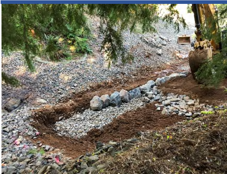
Photo 79 ERRS placing clean topsoil backfill over rock backfill layer in Furnace Creek Old Furnace slide repair area.
