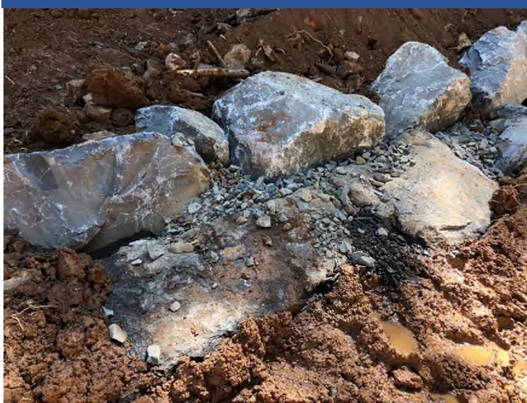
Photo 83 1.5-inch-minus gravel pack placed in interstices of boulder toe anchor at base of Furnace Creek Old Furnace slide.
