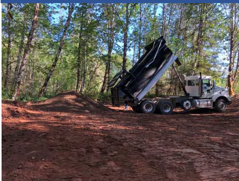
Photo 35 Off-site haul truck delivering loam material for clean backfill in OPWA Lower/South unit.
