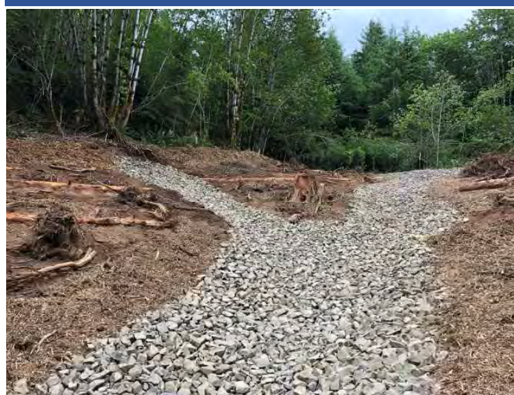
Photo 30 Restored section of OPWA Upper/South unit, with rock-armored seep and constructed drainage channel.
