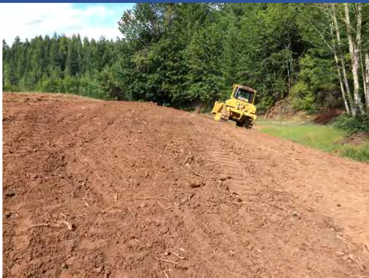
Photo 43 ERRS grading southern slope of expanded repository area.
