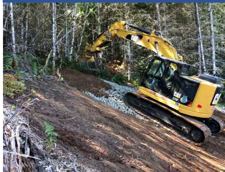
Photo 58 ERRS compacting soil/mulch cover over 6-inch rock armor layer on right bank slope of Adit Creek seep.
