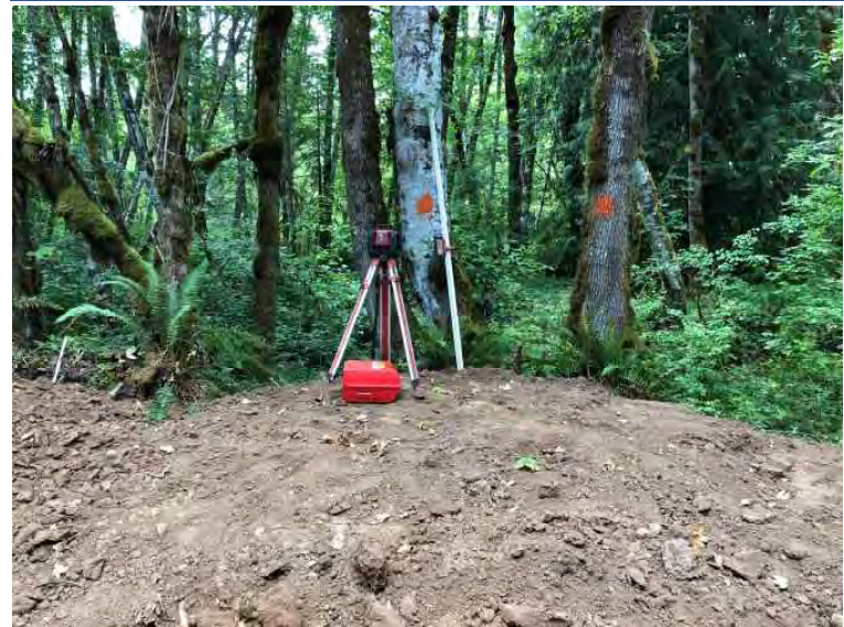
Photo 34 Laser level set up in OPWA Lower/North unit to check for slope and drainage gradient.
