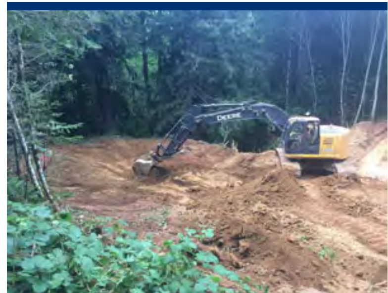
Photo 15 Excavator clearing left bank between STA 8+00 and 8+75.
