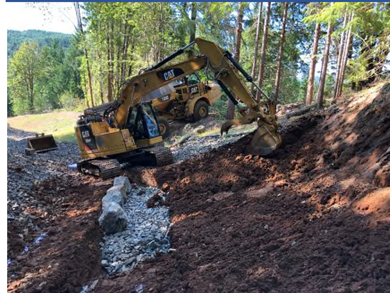
Photo 72 ERRS excavating saturated soils surrounding subsurface seep, located at downstream extent of excavation.
