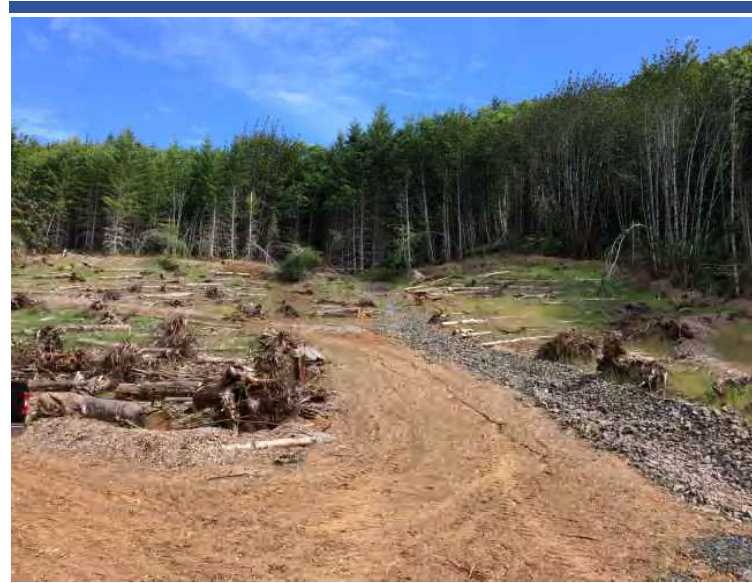
Photo 48 Looking up at BS01 borrow source erosion and Adit Creek seep slope failure at top of slope.
