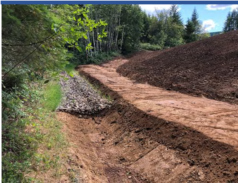
Photo 89 Widened and deepened Adit Creek reroute enhancement to improve flow and drainage around repository.
