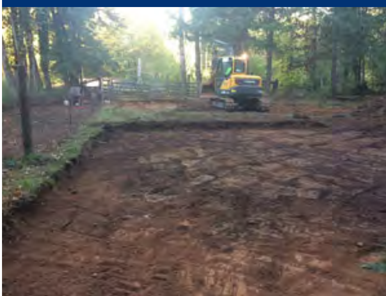
Photo 22 ERRS excavating DU04 to one foot depth.
