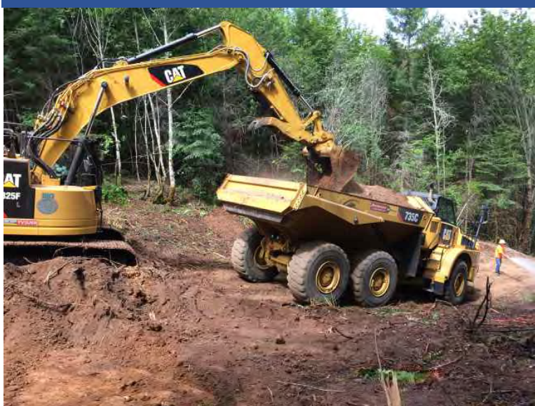
Photo 13 ERRS excavating OPWA Upper/South unit and loading on-site haul truck.
