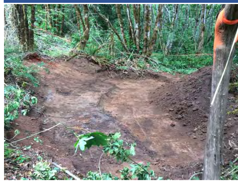
Photo 18 SE extent of OPWA Lower/North unit, excavated in 1-foot benches to target contaminated lenses of ashy material.
