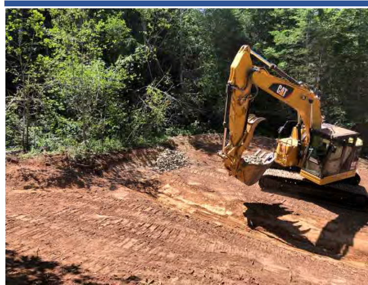
Photo 28 ERRS placing rock armor on contaminated material left in-place at southernmost extent of OPWA Upper/S unit.
