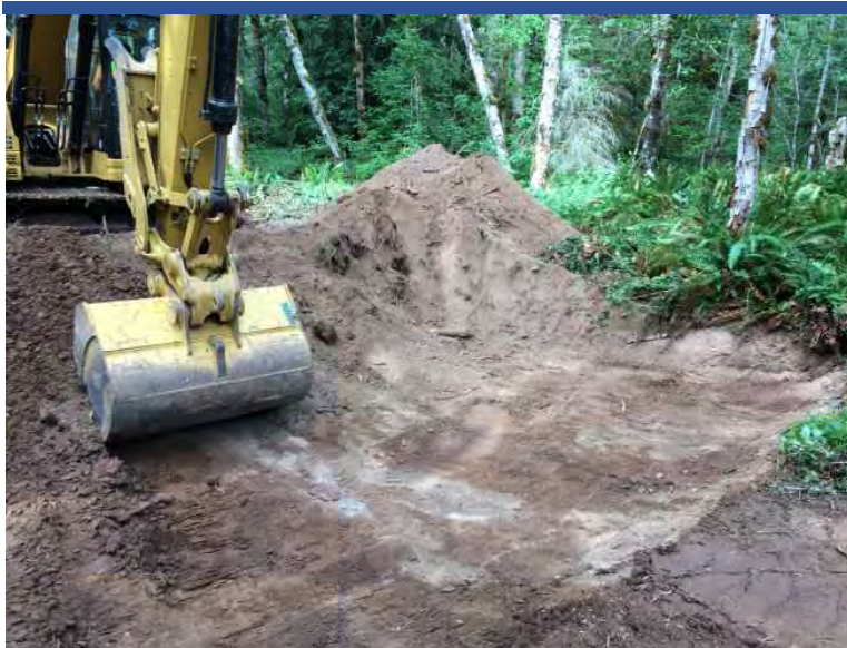
Photo 19 ERRS excavating contaminated lenses of ashy material at SE extent of OPWA Lower/North unit.
