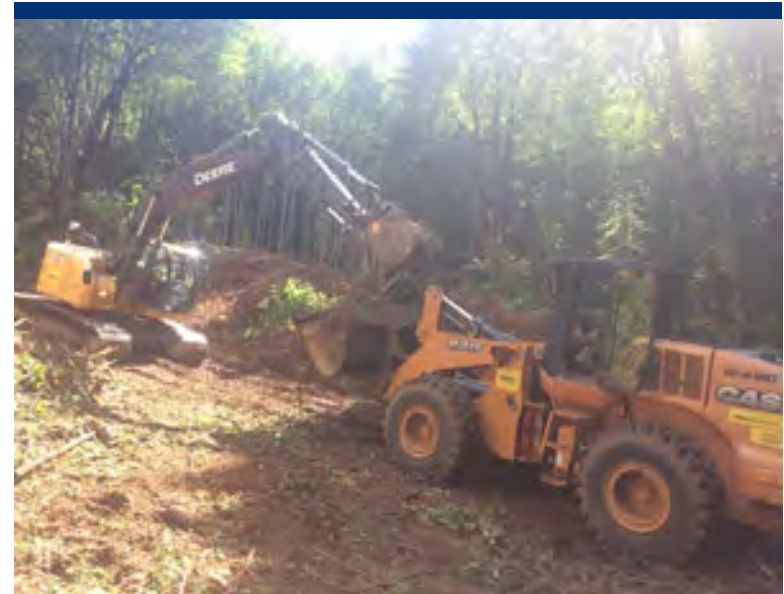
Photo 25 Clearing and grubbing activities at Borrow Source 1.
