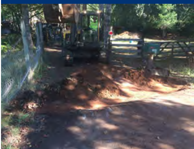
Photo 14 ERRS scraping entrance to main driveway to determine stability of subgrade for gravel bedding.
