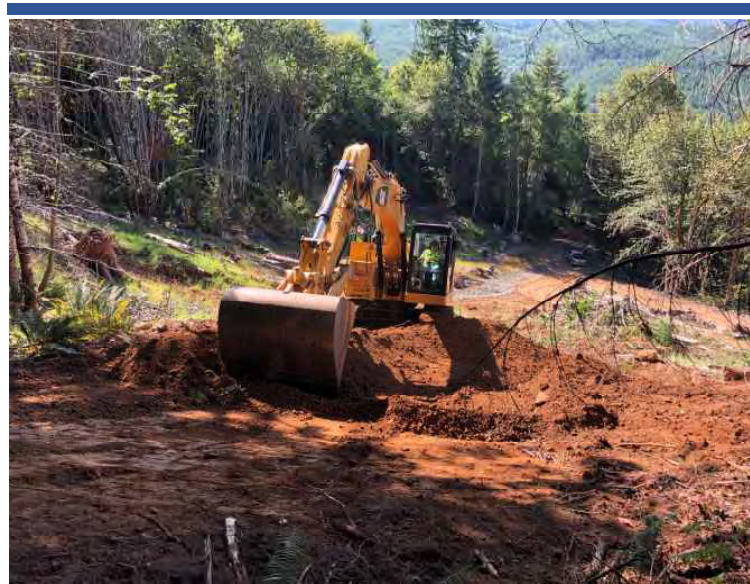
Photo 56 ERRS clearing vegetation above right bank slope failure of Adit Creek seep at BS01, and pulling down slope material.
