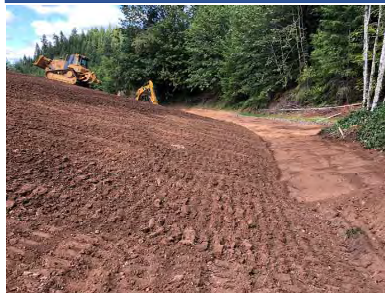
Photo 46 ERRS conducting final grading activities on expanded repository area.
