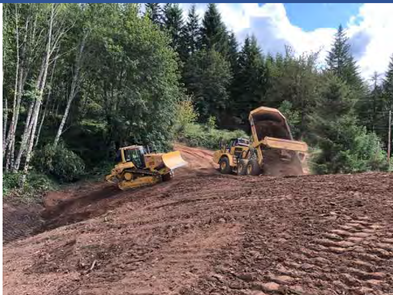
Photo 45 ERRS placing stockpiled residential removal material for main repository 'clean' cap.
