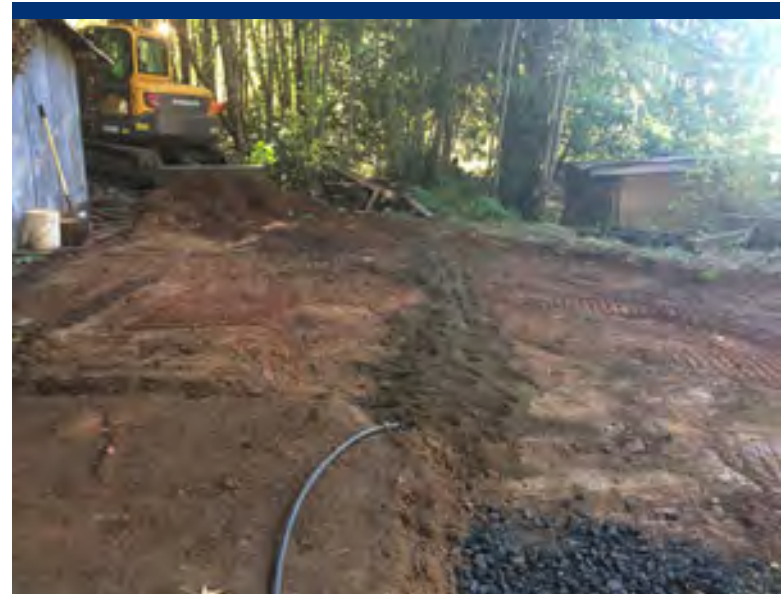
Photo 27 Protective soil backfill placed around water supply line, prior to placement of gravel.
