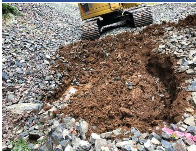
Photo 68 ERRS excavating test pit at upstream extent of toe of Furnace Creek Old Furnace slope failure. Water in pit.
