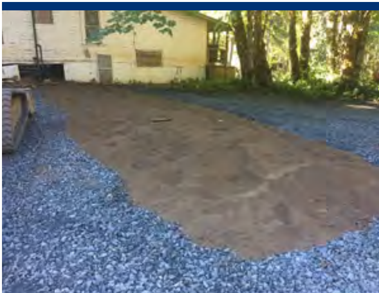
Photo 24 Protective soil backfill placed around septic tank system, prior to placement of gravel.
