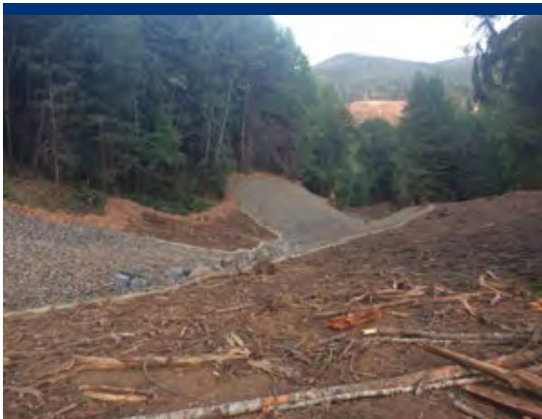
Photo 13 Looking downgradient along restored Furnace Creek channel and slopes with slash.
