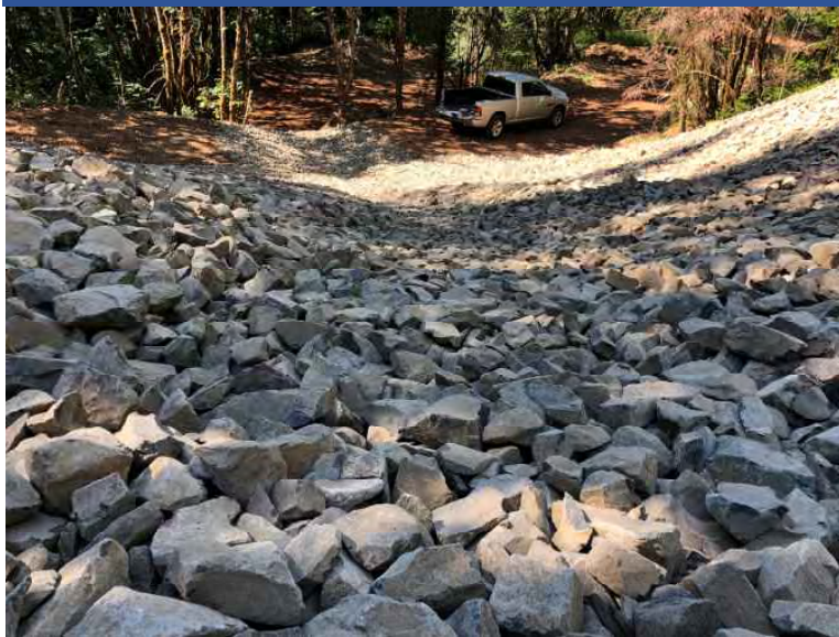
Photo 33 Restored section of OPWA Upper/South unit, with rock-armored slopes and constructed drainage channel.
