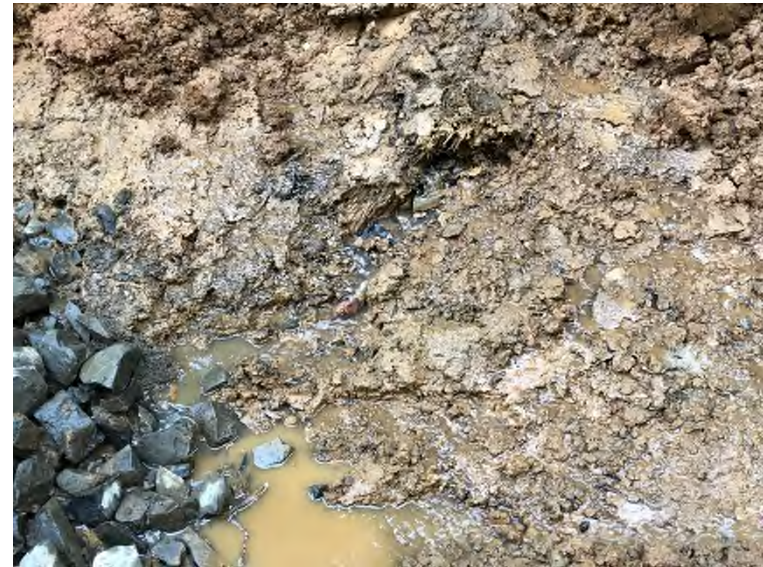
Photo 78 Groundwater and exposed tailings in key anchor trench at toe of Furnace Creek Old Furnace slide repair area.
