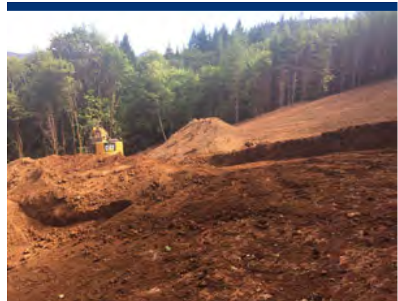
Photo 27 Stockpiling of fill material from Borrow Source 1.
