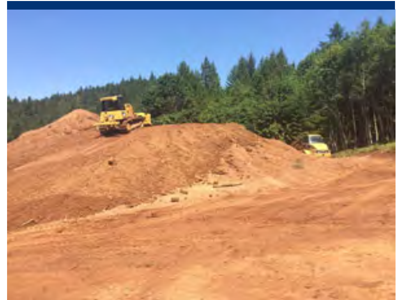
Photo 13 Haul truck dumping excavated material at repository and dozer grading repository.
