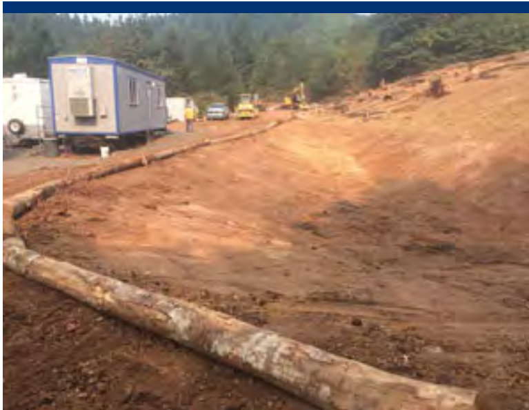
Photo 23 Completed repository retention pond.
