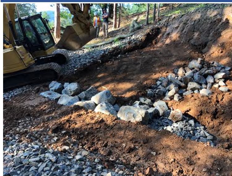
Photo 74 ERRS compacting clean backfill over rock layer slope in Furnace Creek Old Furnace slide repair area.
