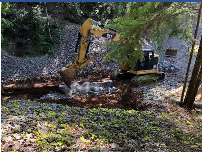
Photo 73 ERRS placing boulder toe anchor above rock-filled key trench at base of Furnace Creek Old Furnace slide repair.
