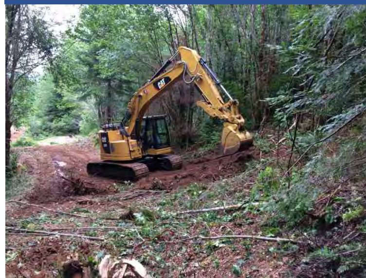
Photo 6 ERRS conducting clearing and grubbing activities at OPWA Upper/South unit.
