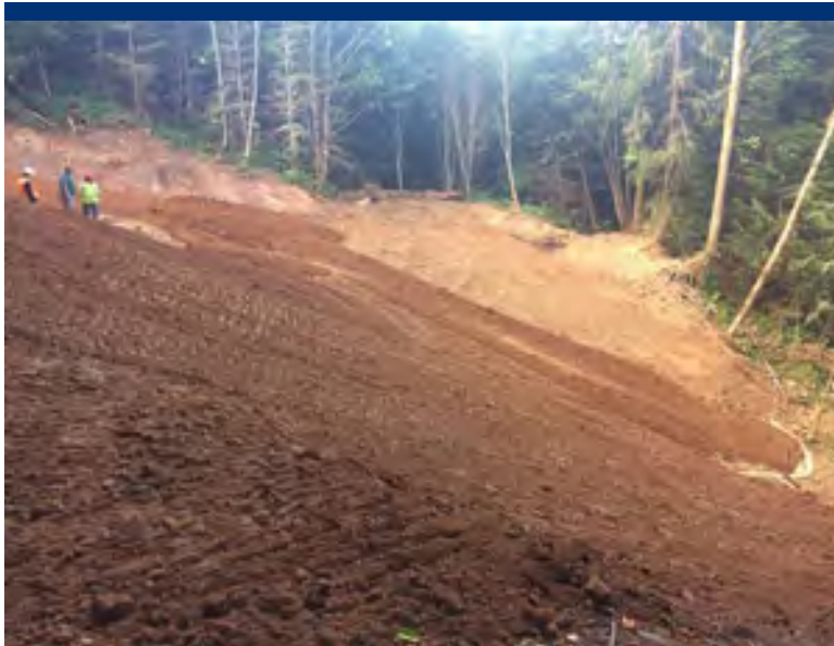
Photo 5 Lower reach of Furnace Creek removal area with backfilled and graded channel and slopes, near STA 8+50.
