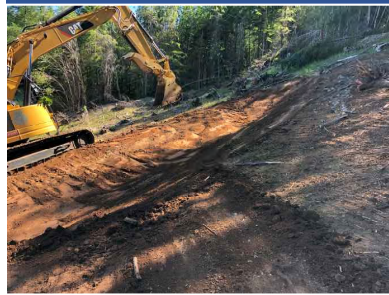
Photo 62 Right bank Adit Creek seep intercept channel installed by ERRS to direct flow into main Adit Creek channel.
