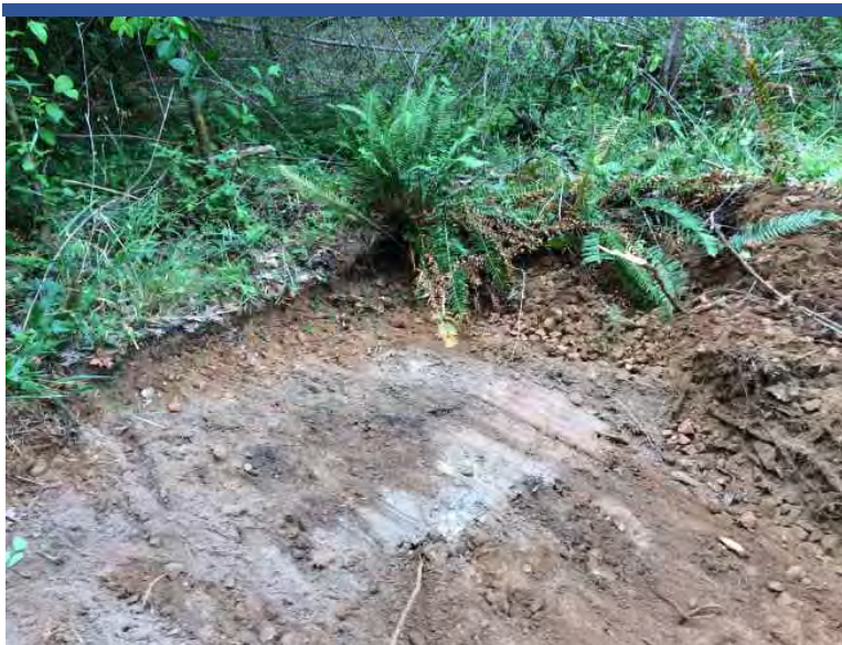
Photo 11 Excavated upper/southernmost boundary extent of OPWA Upper/S unit. Contaminated ash layer visible.
