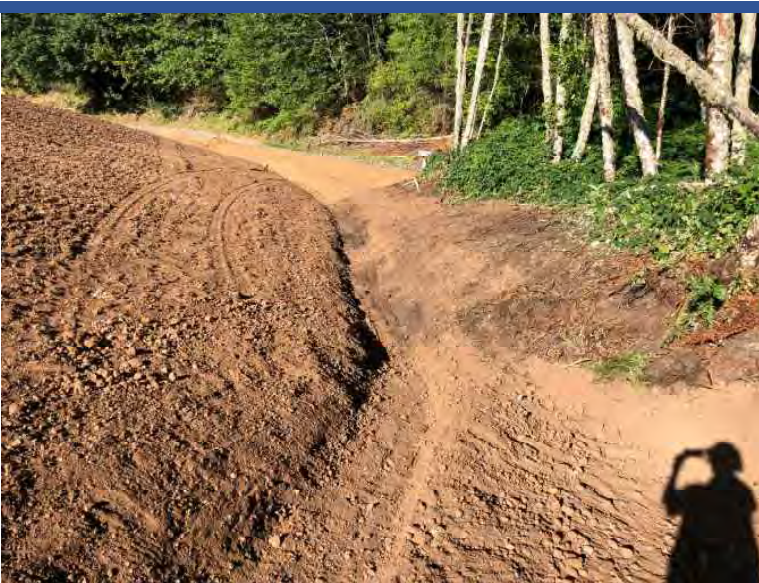
Photo 47 Looking east along toe of south extent of expanded repository, and stormwater drainage channel.
