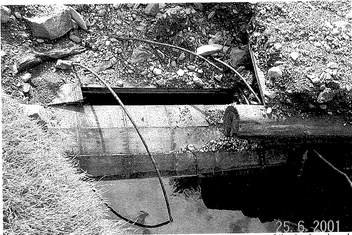
Top of penstock showing one of the broken staves, and one of the broken bands
