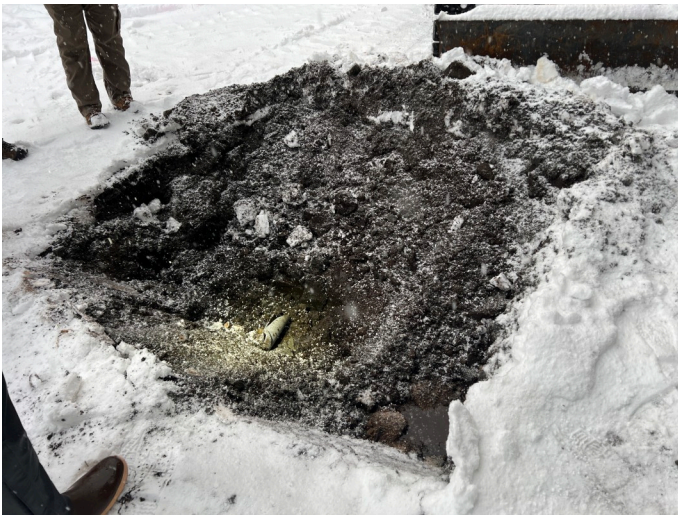
Overview of more exposed abandoned utility conduit.
