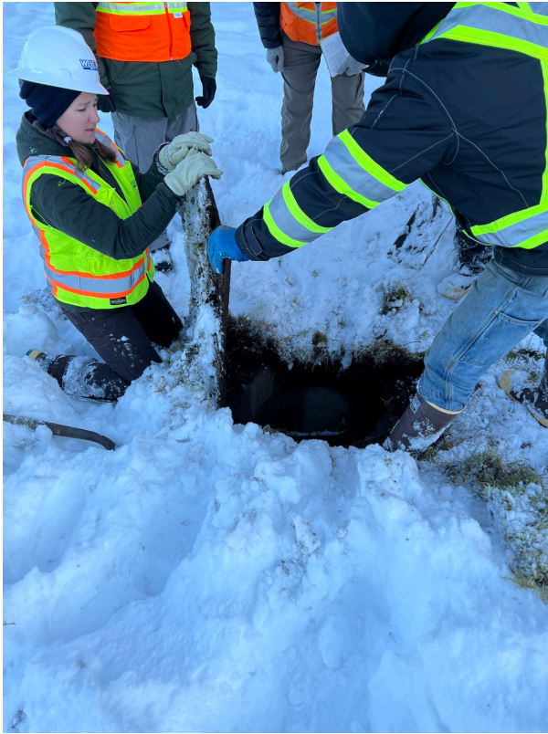
NE 38. Removal of storm drain cover.
