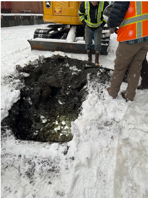
SE 57°. Removal of small likely abandoned utility pipe.
