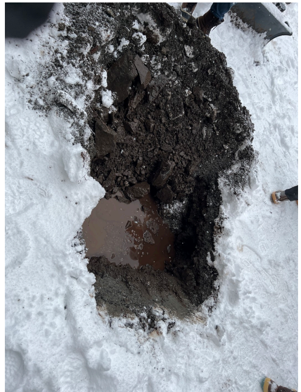
Overview of completed excavation to 2'.
