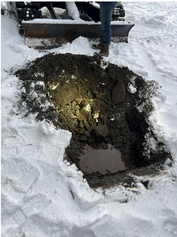
Overview of second location and ground water at 15" below the surface.
