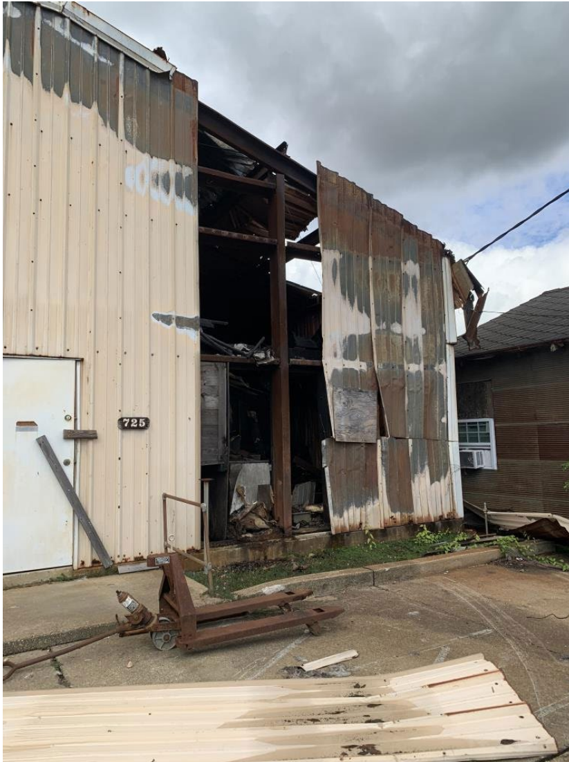
Missing portion of the wall on the East side of the facility post-Hurricane Ida
