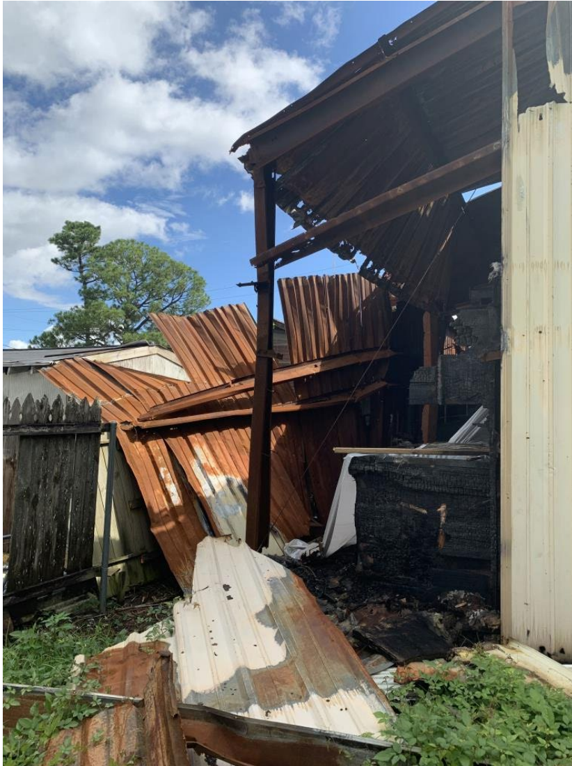
Missing portion of the wall on the West side of the plating facility post-Hurricane Ida
