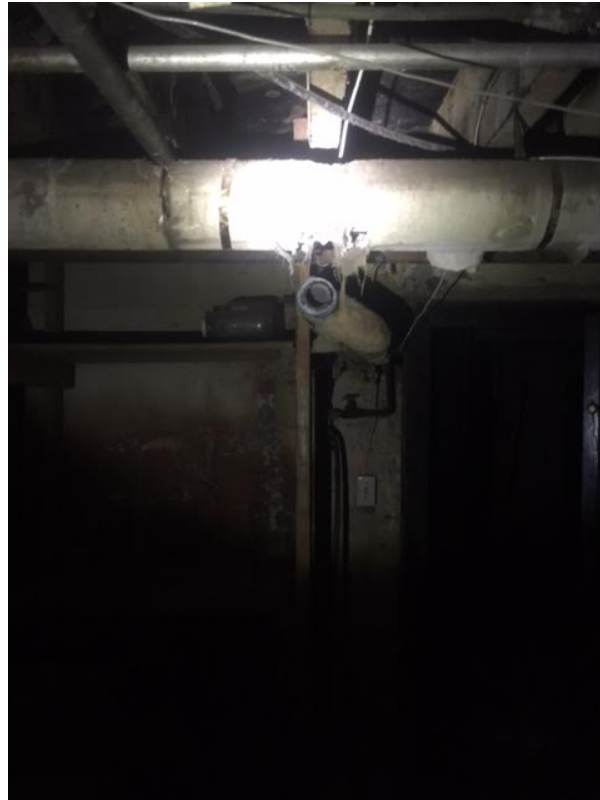
Photo 11: Asbestos positive thermal systems insulation in the basement of the hotel/lounge building.
