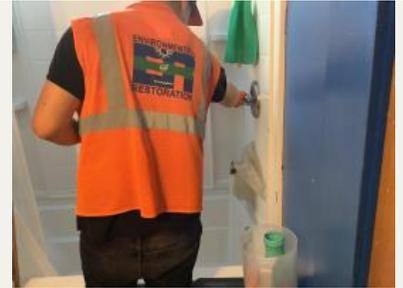
Description: Monitoring water for contamination during the flushing of an external water tap.
