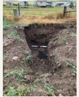
Description: Control valve in water distribution system piping installed by the operator at lot 1 to isolate the contaminated homes.
