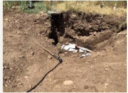
Description: Absorbent pads used to collect the oily substance of concern from water collected under the control valve located at lot 7.
