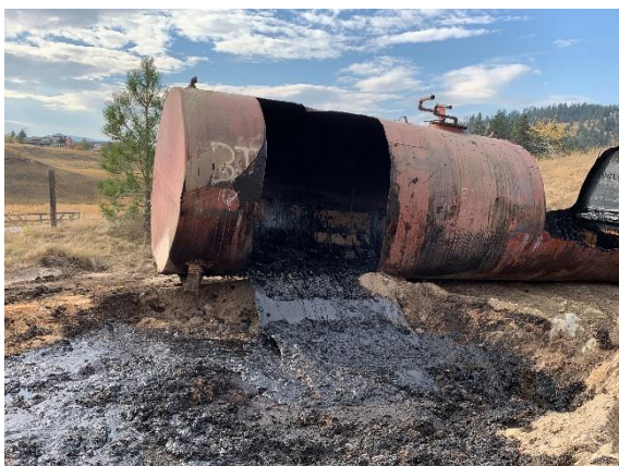
Tank #13 draining into solidification pit #2
