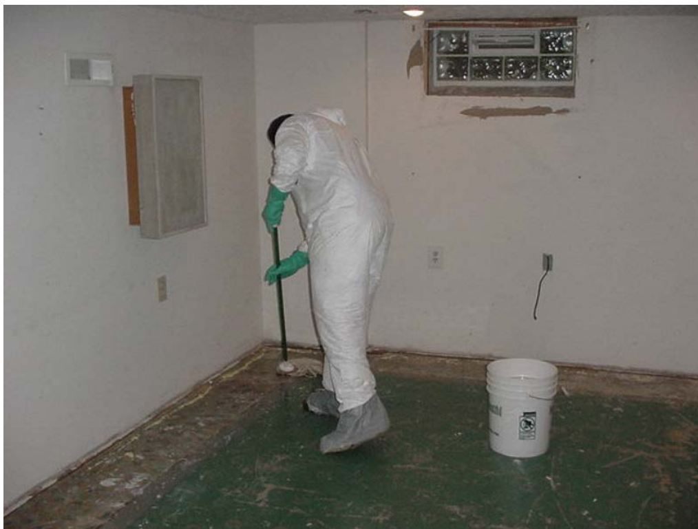
Photograph 9-4 Mopping floors with mercury treatment solution
