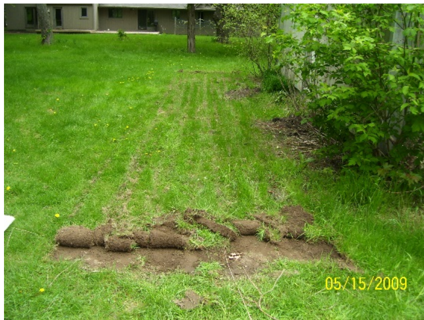
Photograph 9-17 View of a soil/sod cutting operation
