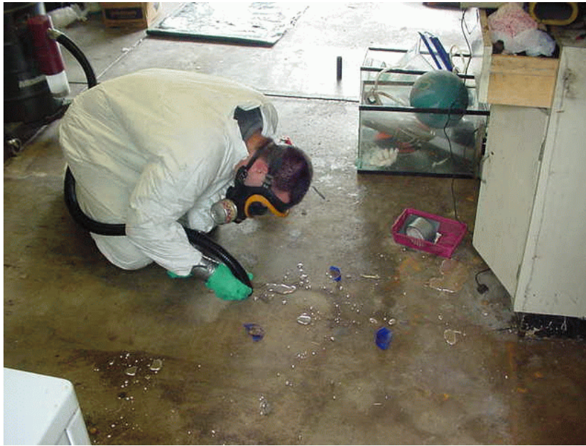
Photograph 9-3 Removal of elemental mercury with a mercury vacuum
