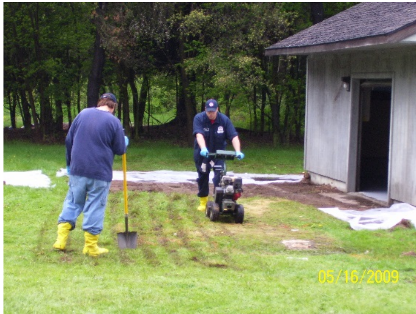
Photograph 9-16 View of a soil/sod cutting operation
