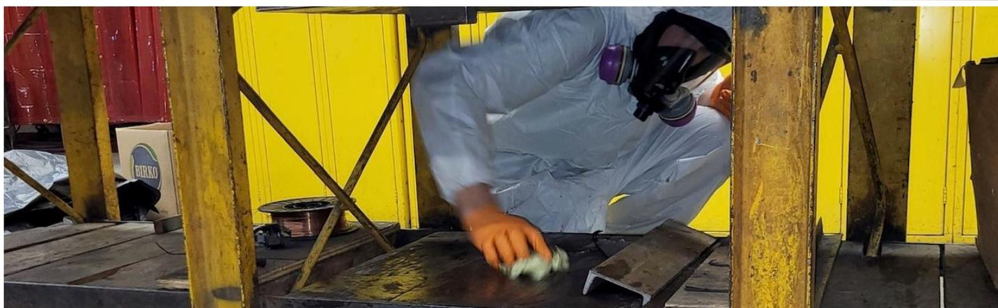
**Photo Description:** EPA's Response Team treating the surfaces of the Welding Shop table with a solution to chemically react with the mercury and create a non-hazardous solution.
