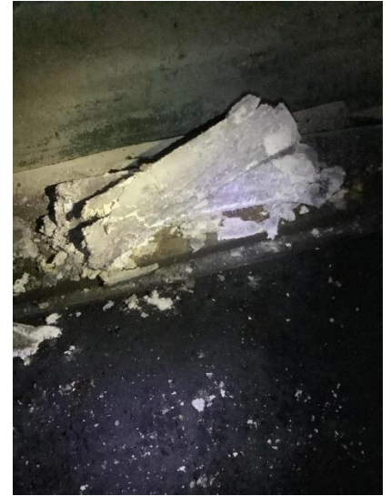
Image 2: Friable asbestos on the floor of the site.
