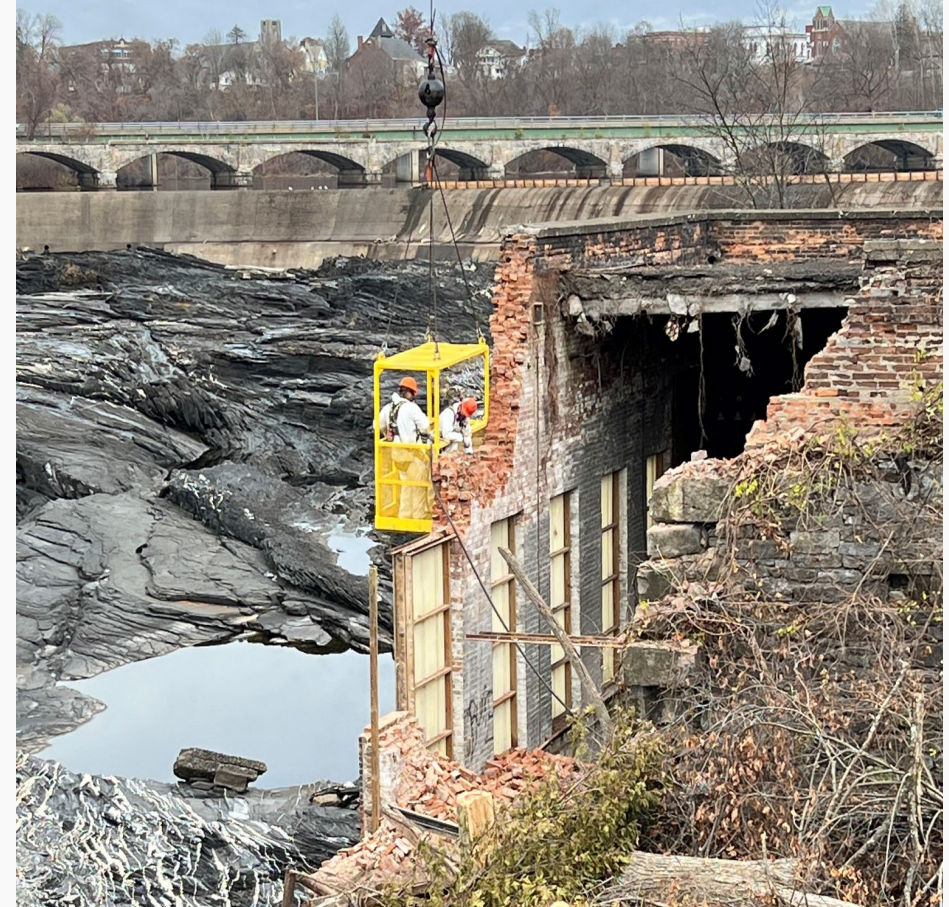
This photo shows the Powerhouse building being carefully dismantled using hand tools to limit disturbances to bedrock and minimize fallen debris into the river
