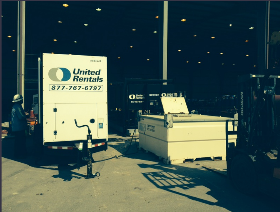
Chiller system installation. The generator, fuel oil tank and chiller are shown
