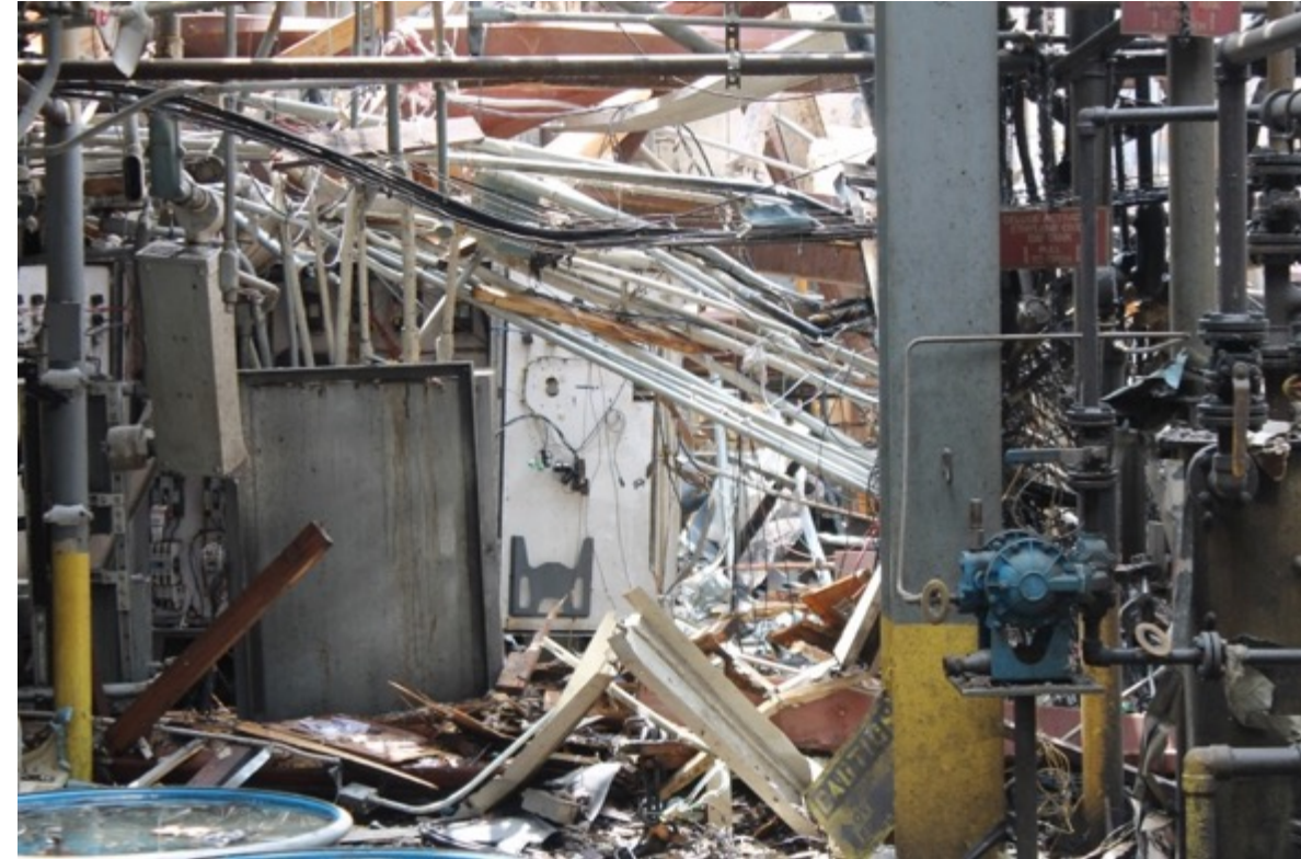
The plant building, formerly a control room, was destroyed by the explosion and fire, and was the location where the decedent, a plant operator, was found.
