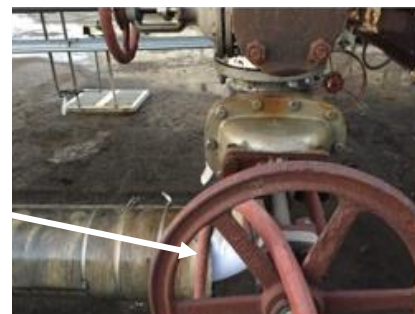
Figure 4-12 Circle left picture is Fire Command; middle upper circle is the MC 331 trailer at the loading terminal; circle that links to the right side picture is the 14-inch pipeline valve with a blown gasket.
