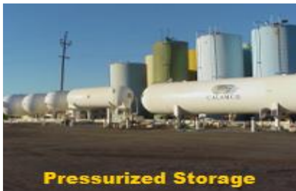
Figure 4-8 Left Pressurized bullet tanks (500 tons capacity); Right One of two Low pressure (0.5 psi) low pressure ammonia 20,000 tons of ammonia storage.
