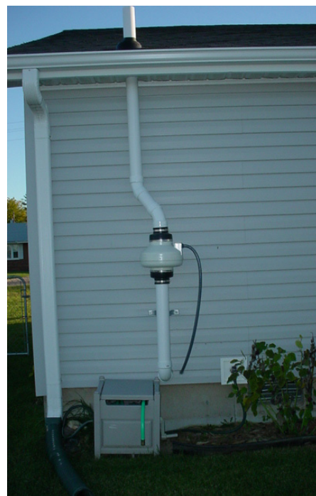
Figure 4-3. Active subslab depressurization system.
