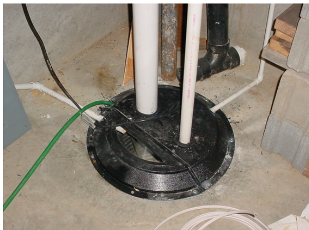
Figure 4-2. Passive sump mitigation system.
