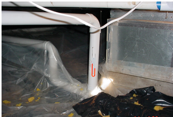
Figure 4-4. Crawl-space mitigation using submembrane depressurization. Courtesy Kansas Department of Health and Environment
